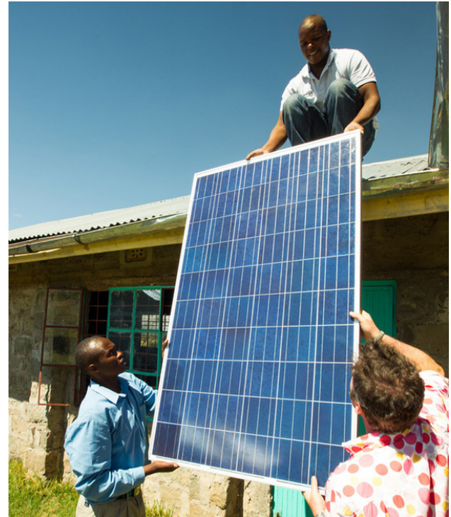
Wireless network infrastructure was powered by solar energy.
