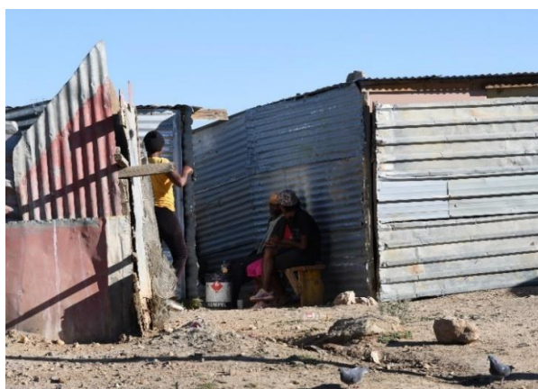
SAEP is working with the City of Windhoek to develop an approach to electrify more households in informal settlements. Photo: SAEP
