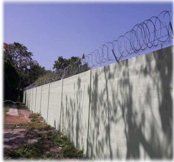
Figure 2: Newly constructed perimeter fencing at St. Jago High School
