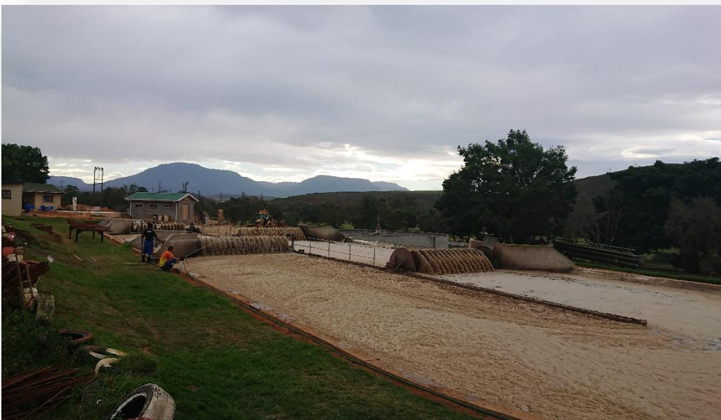
Figure 6 Hessequa Municipality Waste Water Treatment Works
