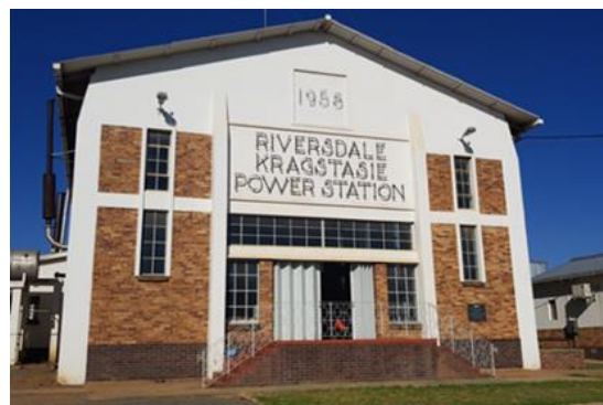
Photo 3: The Hessequa Power Station
