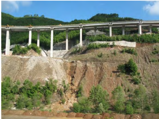
Photo 3. Highway construction without erosion control (and dissecting the country north-south and east-west)
