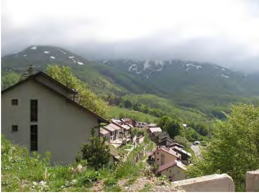
(Photo 6. Construction of the tourist village at Prevala/Prevallac in Malet e Sharrit/Šar Planine National Park adjacent to Zone 1 (the structures and ancillary features are illegal).)
