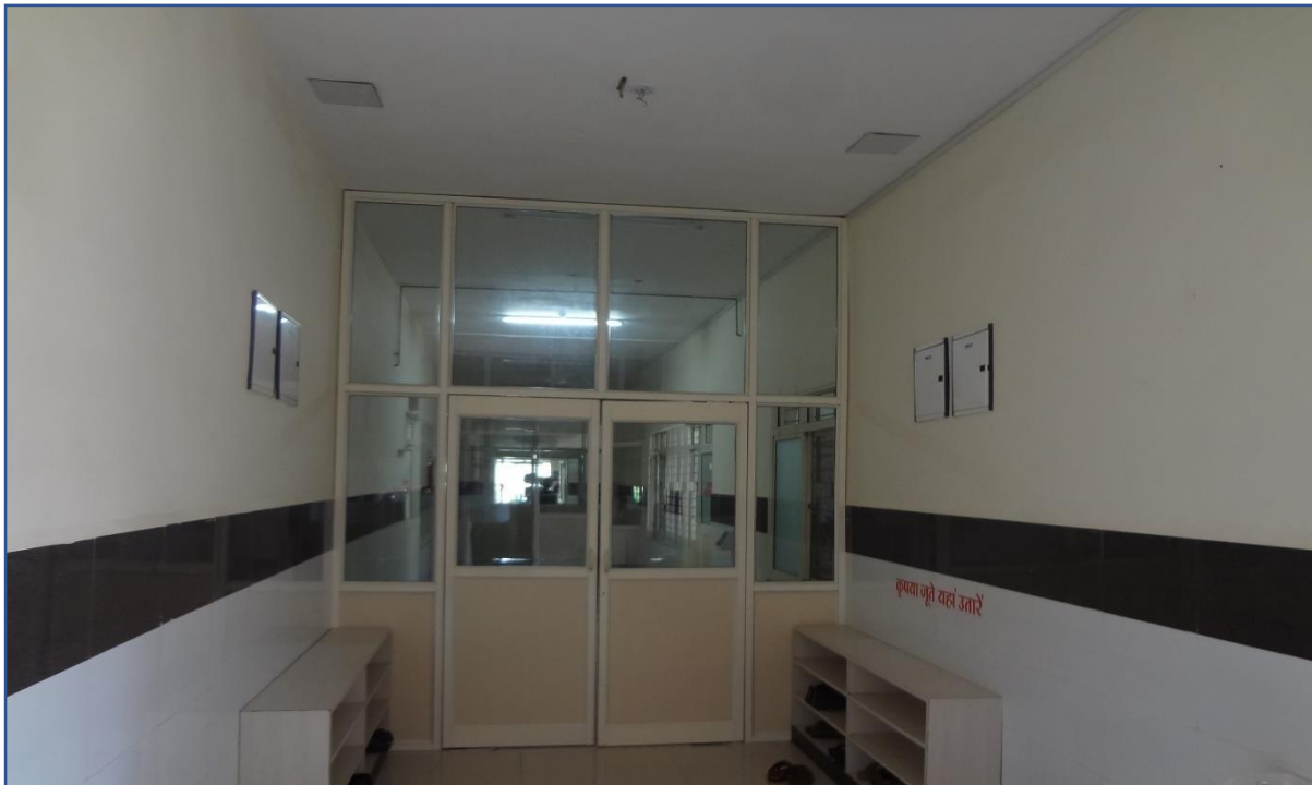
Separate partitioned section inside IPU to accommodate infant and pediatric wards with dining and waiting areas. All steps must be ensured for proper aseptic conditions in wards.
