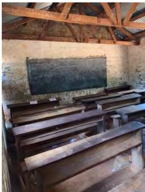
PHOTO 4 CLASSROOM IN GARCIA NURSERY AND PRIMARY SCHOOL IN YAMBIO
