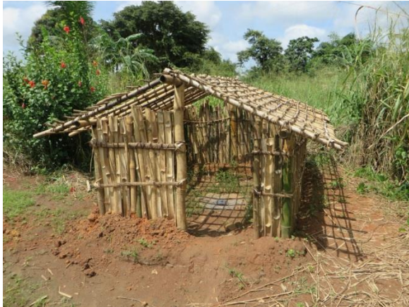
Superstructure construction of a burial pit in progress CS Triangle Bas-Uélé
