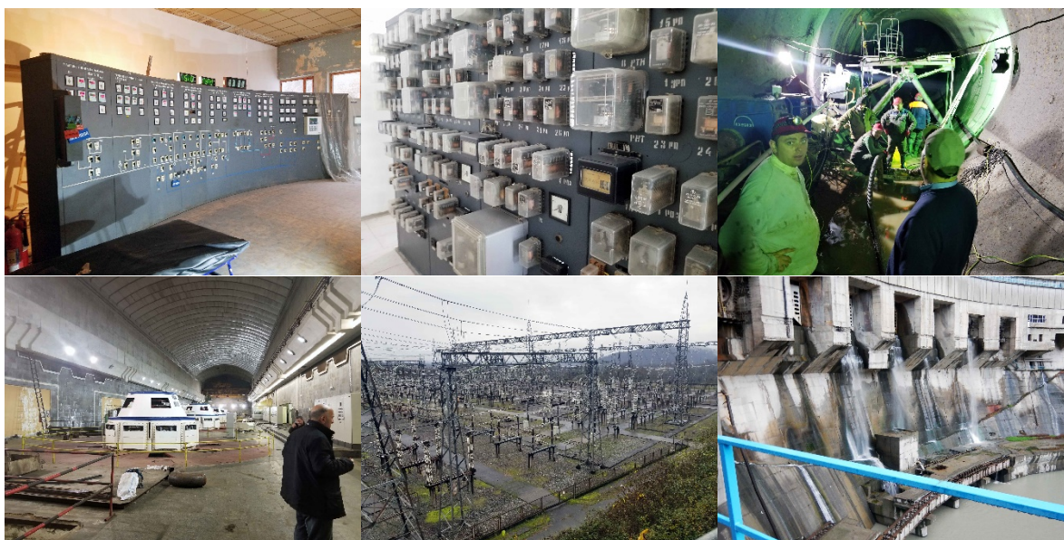
Inspection of Enguri Hydro Power Plant
