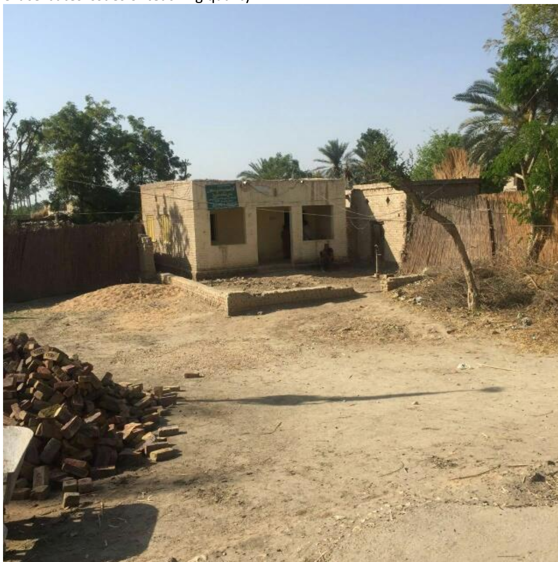
A single room school in Khairpur, which is also used as an NFE Centre
