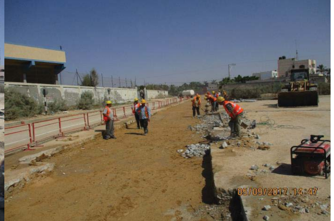
Photo No.04: Surface restoration work trench excavation and compaction Date: September 5, 2017
