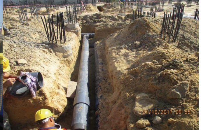
Photo No.40: RO building - installation of underground PVC pipes. Date: October 21, 2017
