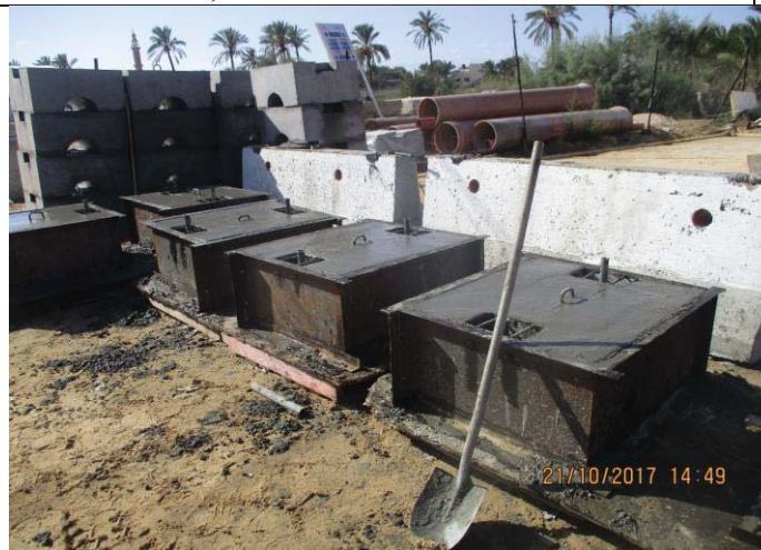
Photo No.41: Weight collars for outfall pipeline activities. Date: October 21, 2017
