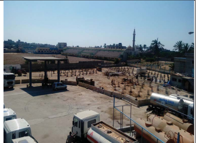
Photo No.26: Piles construction activities Date: July 19, 2017
