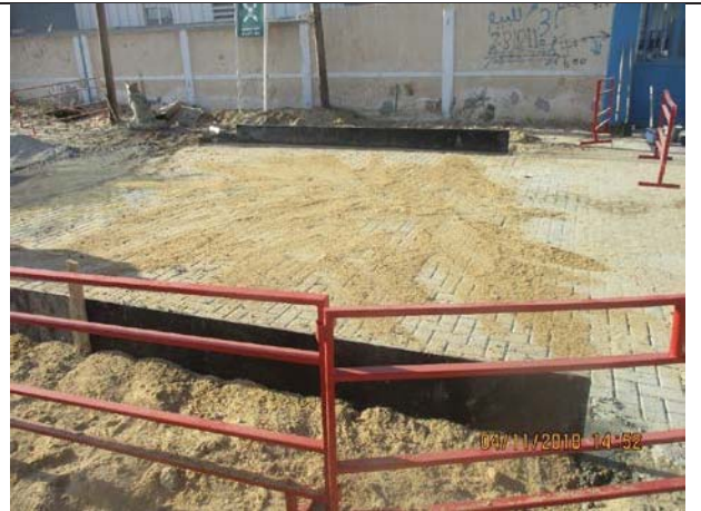
Photo No.02: Tiles reinstatement works front of construction site Date: November 04, 2018
