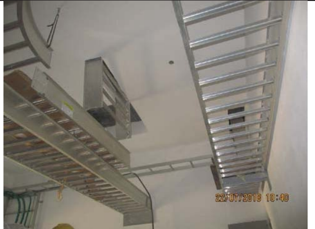
Photo No.26: Cable ladder installation inside electrical room Date: July 22, 2018
