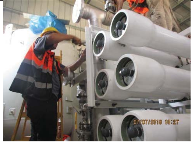
Photo No.08: Continue assembly of 2 nd pass RO skid Date: July 07, 2018
