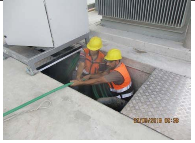
Photo No.26: Connection works for cables of generator area. Date: September 23, 2018
