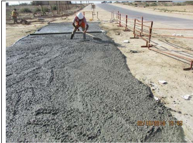
Photo No.01: Casting concrete for reinstatement works above chambers Date: October 02, 2018
