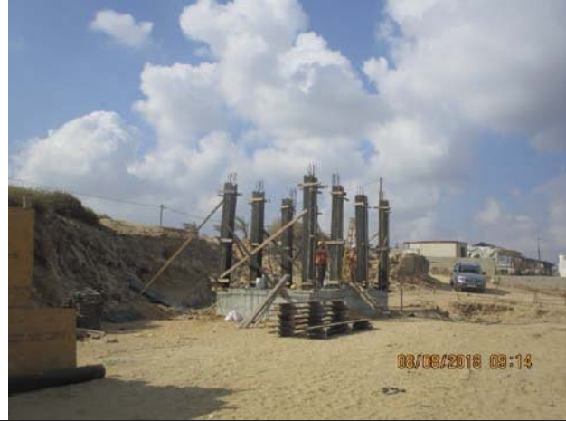
Photo No.15: Shuttering works for electrical room columns Date: August 08, 2018
