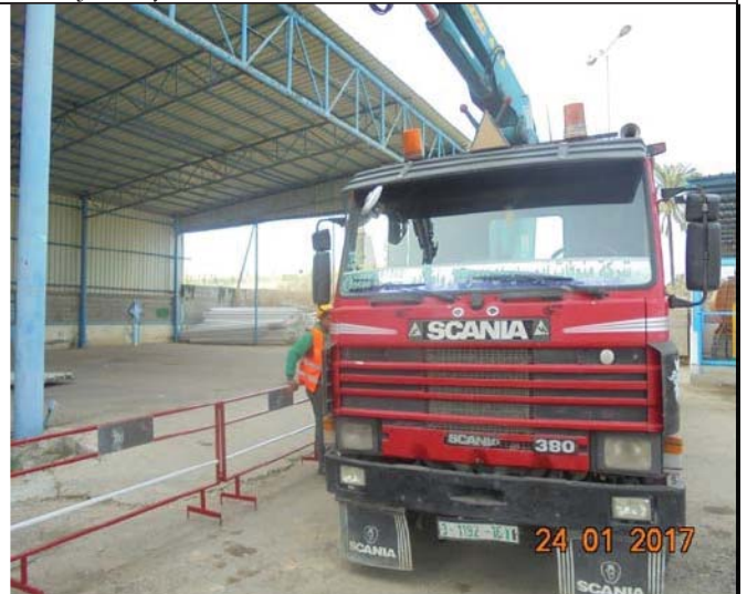
Photo No.04: Start demolition of existing canopy steel structure Date: January 24, 2017
