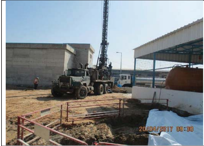
Photo No.17: Piles construction at the RO building.
