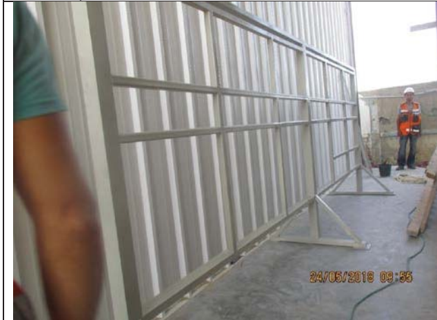
Photo No.21: PV system canopy installation for pretreatment area. Date: May 24, 2018
