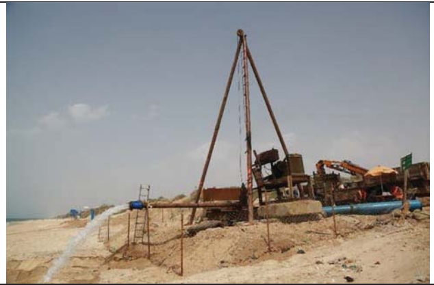
Photo No.02: Pumping test for beach well No.2 Date: May 02, 2018
