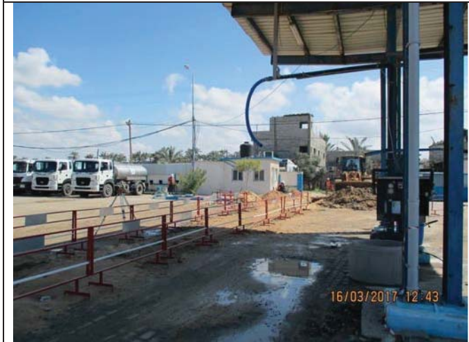
Photo No.13: Storm water catchment relocation. Date: March 16, 2017
