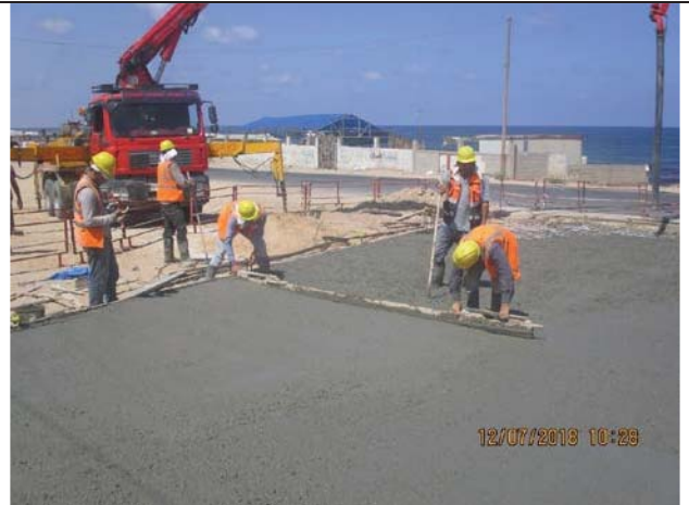
Photo No.16: Concrete reinstatement on Al-Rasheed Street Date: July 12, 2018
