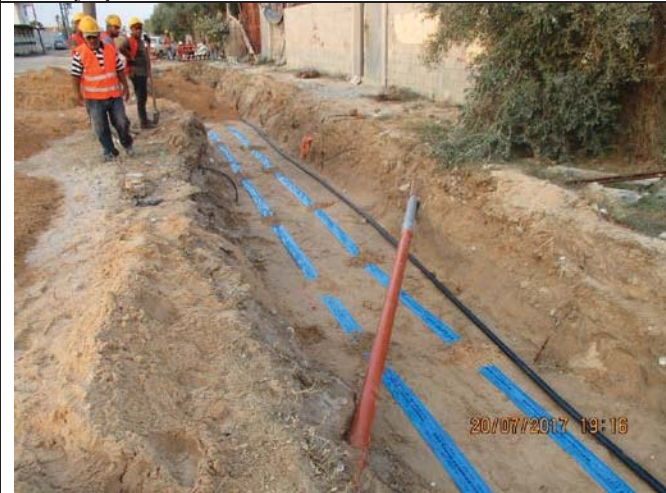
Photo No.33: Pipeline (outfall and intake) warning tape installation. Date: July 20, 2017
