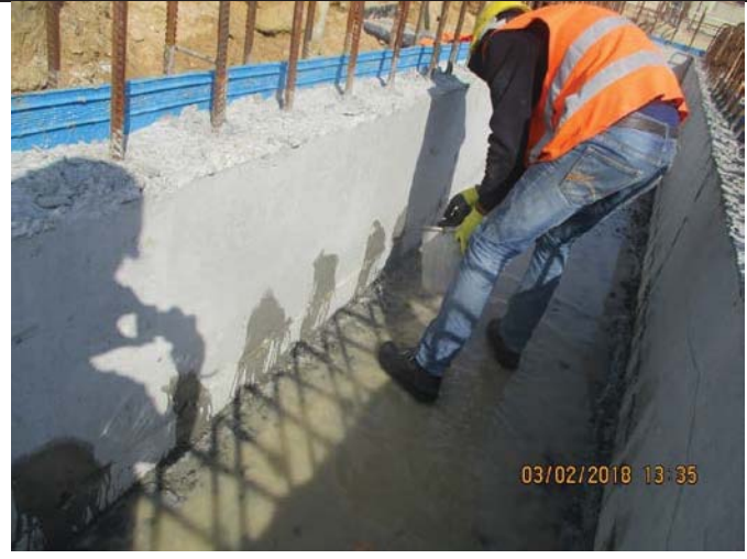
Photo No.04: Repairing works for the generator pad trench
