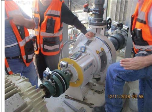
Photo No.07: Alignment works for shaft coupling of pumps Date: November 12, 2018
