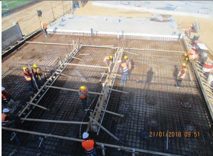
Photo No.23: Steel Reinforcement for pretreatment foundation. Date: January 18, 2018
