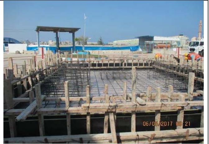
Photo No.02: Fuel tank relocation activities Date: May 06, 2017
