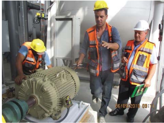
Photo No.07: Leveling and alignment works for pumps Date: September 06, 2018
