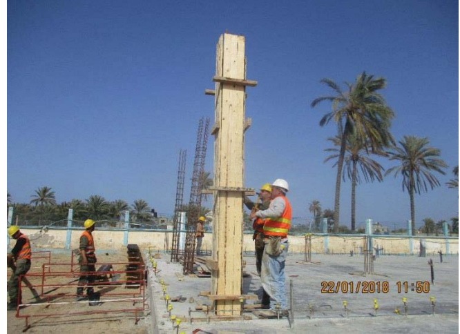
Photo No.28: Steel reinforcement and formwork for electrical room columns.
