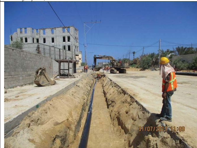
Photo No.41: Installation of 450 mm & 315 mm HDPE pipes. Date: July 31, 2017
