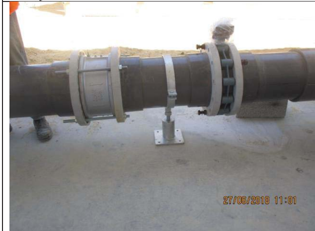
Photo No.29: Pipe support installation Date: June 27, 2018
