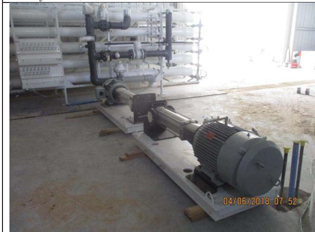
Photo No.05: Installing pressure pump Date: June 04, 2018
