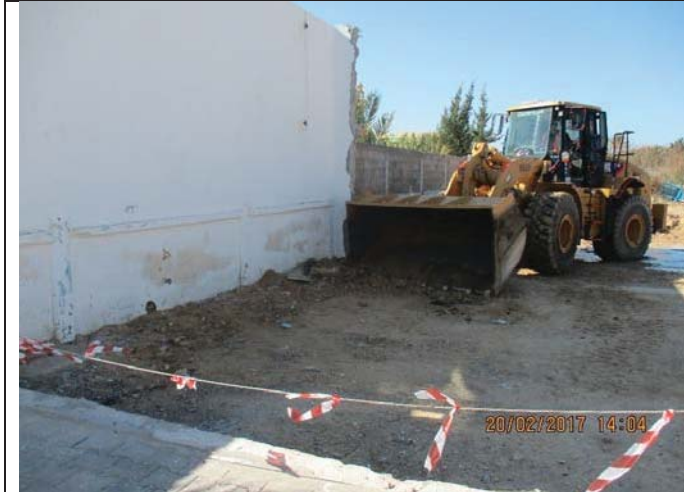
Photo No.17: Site cleaning and leveling Date: February 20, 2017
