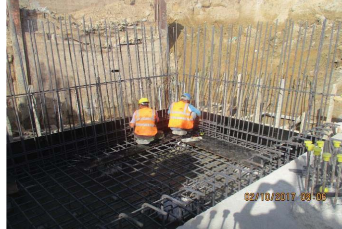
Photo No.03: Brine tank construction activity (steel reinforcement work ) Date: October 2, 2017
