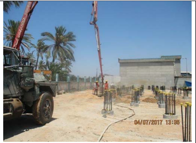
Photo No.08: Pile construction activity. Date: July 04, 2017
