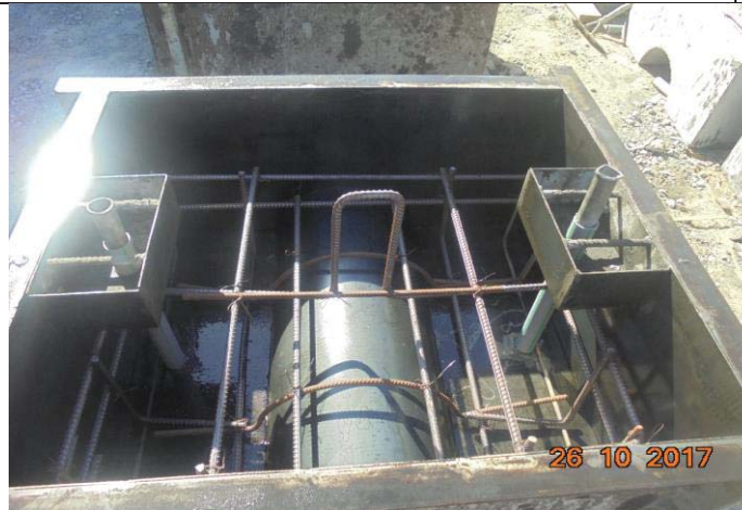
Photo No.51: Outfall pipeline construction activity (weight collar) Date: October 26, 2017
