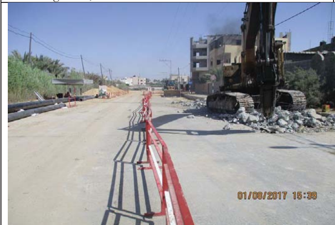
Photo No.03: Pipeline preparation activities (demolish road concrete surface). Date: August 01, 2017
