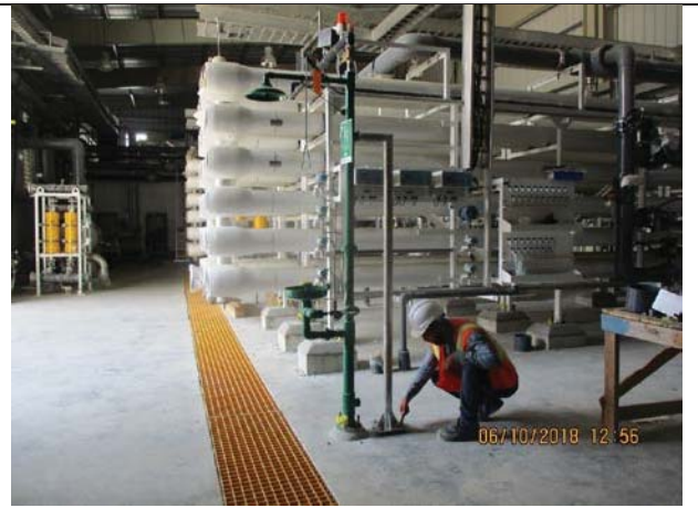
Photo No.04: Steel support installation for eyewash. Date: October 06, 2018
