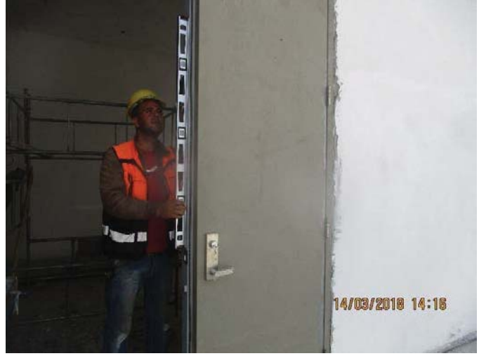
Photo No.12: Door installation for electrical room. Date: March 14, 2018
