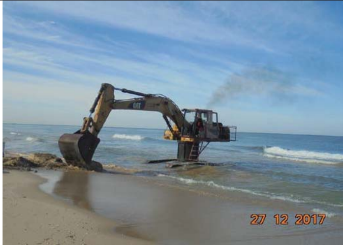
Photo No.49: Trial run for outfall pipeline installation Date: December 27, 2017
