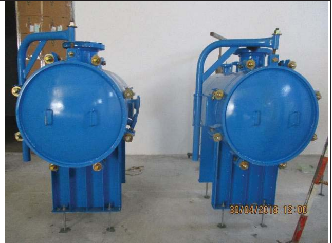
Photo No.44: Mechanical equipment installation Date: April 30, 2018
