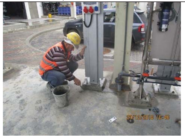
Photo No.28: Punch list activities Date: December 29, 2018
