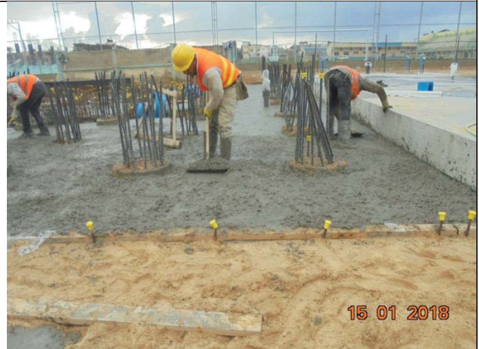
Photo No.16: Shuttering works and steel reinforcement for RO foundation (phase 2). Date: January 14, 2018
