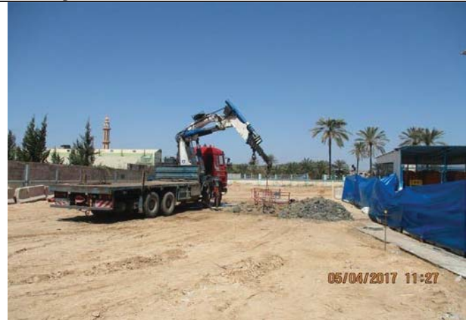
Photo No.07: Installation of reinforcement steel case. Date: April 05, 2017
