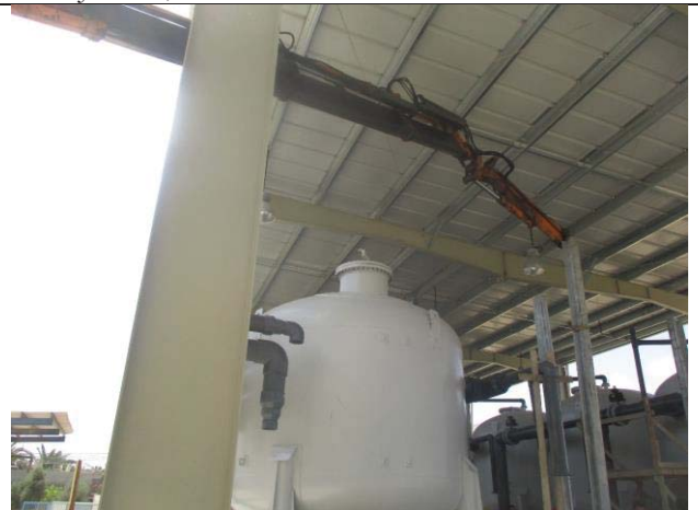
Photo No.24: Steel support installation for pretreatment area. Date: June 23, 2018
