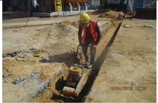
Photo No.20: Backfilling works for duct banks. Date: April 15, 2018
