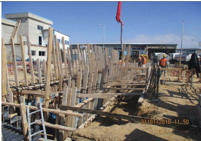
Photo No.49: Casting concrete for generator pad trench Date: January 31, 2018
