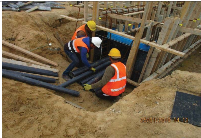
Photo No.35: Electrical conduits installation for generator pad trench. Date: January 25, 2018
