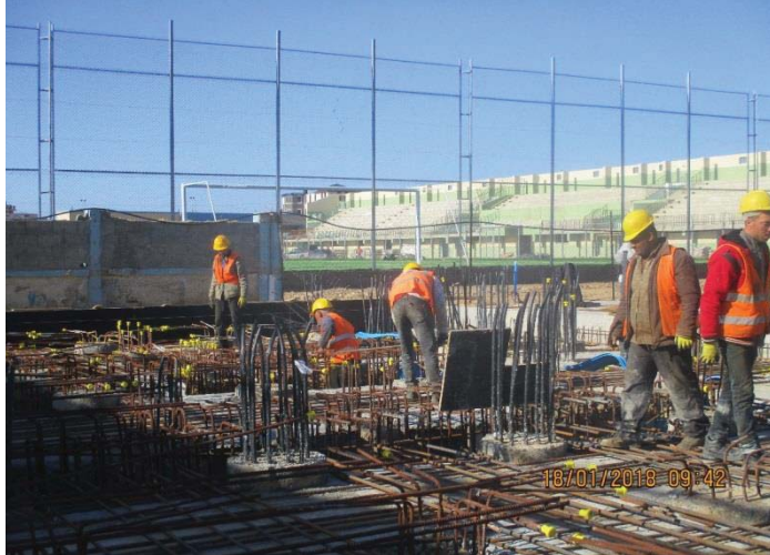
Photo No.23: Steel Reinforcement for pretreatment foundation. Date: January 18, 2018
