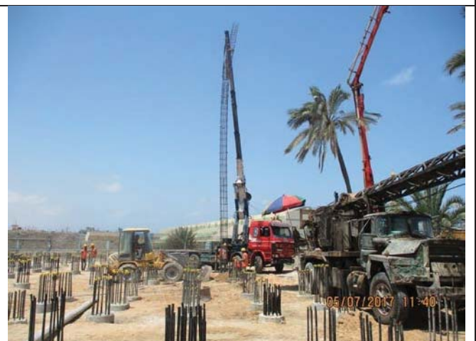
Photo No.10: Piles reinforcement case installation. Date: July 05, 2017
