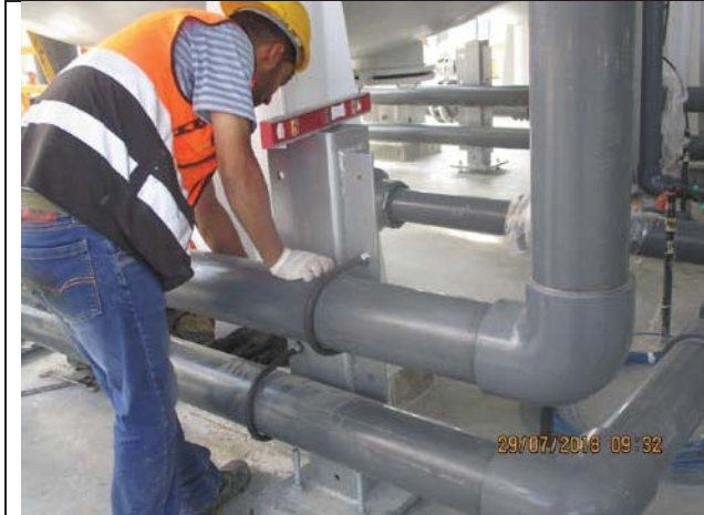
Photo No.37: Clamps installation Date: July 29, 2018
