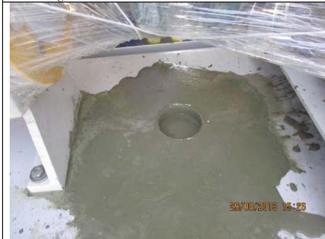
Photo No.27: Grouting works for feed pumps. Date: August 29, 2018
