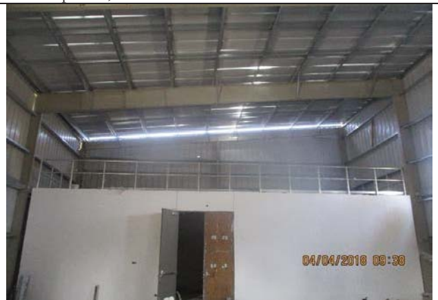
Photo No.10: Handrail installation for electrical room slab. Date: April 04, 2018
