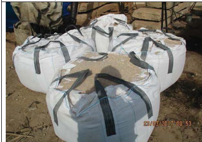
Photo No.27: Continue hydrogeology investigation for beach wells – gravel back filling.
