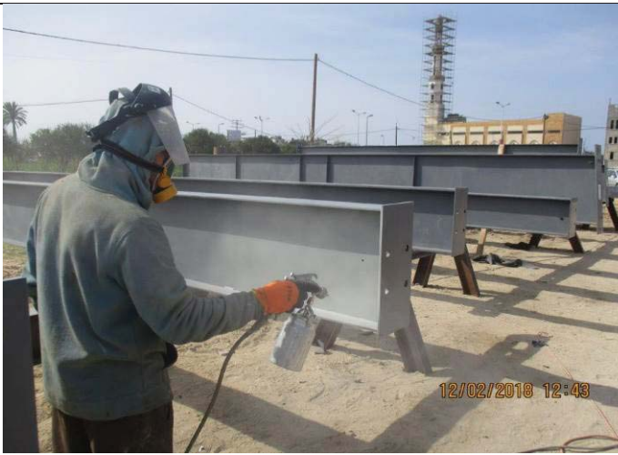
Photo No.19: Continue epoxy coating for steel structure Date: February 12, 2018
