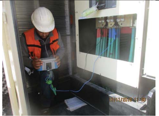
Photo No.08: Electrical works and tests inside electrical room Date: November 17, 2018
