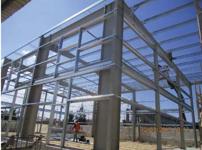
Photo No.09: Continue works in workshop walls Date: March 12, 2018
