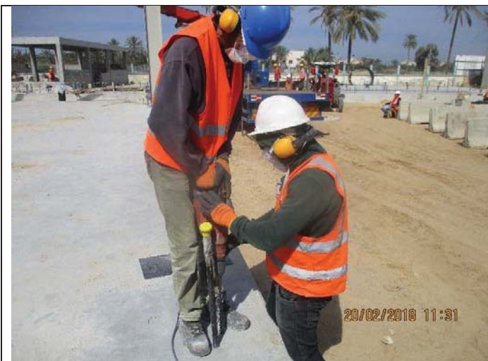
Photo No.29: continue drilling works to install anchor bolts for pretreatment steel structure. Date: February 20, 2018
