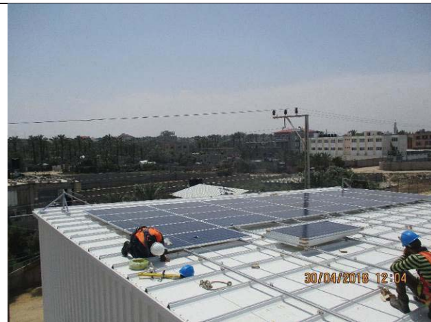
Photo No.45: PV panels installation for pretreatment canopy Date: April 30, 2018
