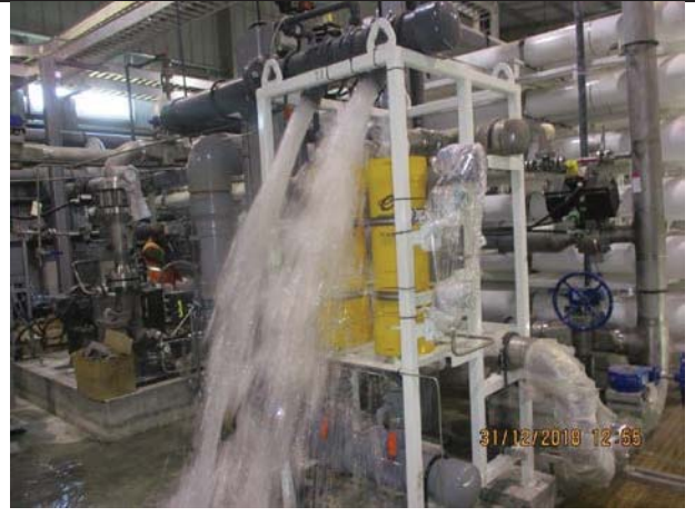
Photo No.32: Flushing RO pipes Date: December 31, 2018
