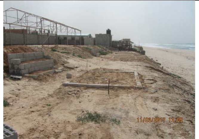
Photo No.06: Survey works to allocate proposed beach wells 01, 02 & 03 coordinates based on the new layout. Date: March 11, 2017
