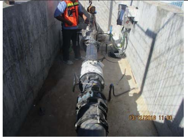
Photo No.14: Manifold installation for beach wells Date: December 13, 2018
