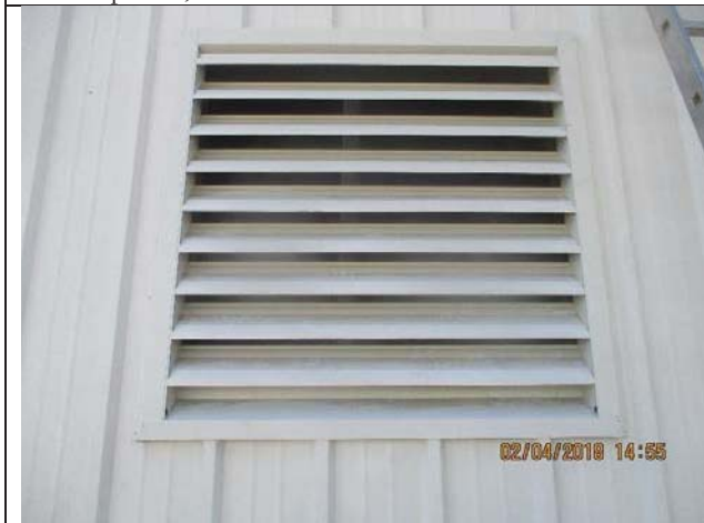
Photo No.03: Louver installation for workshop area. Date: April 02, 2018
