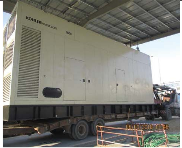
Photo No.08: Generators installation Date: September 06, 2018
