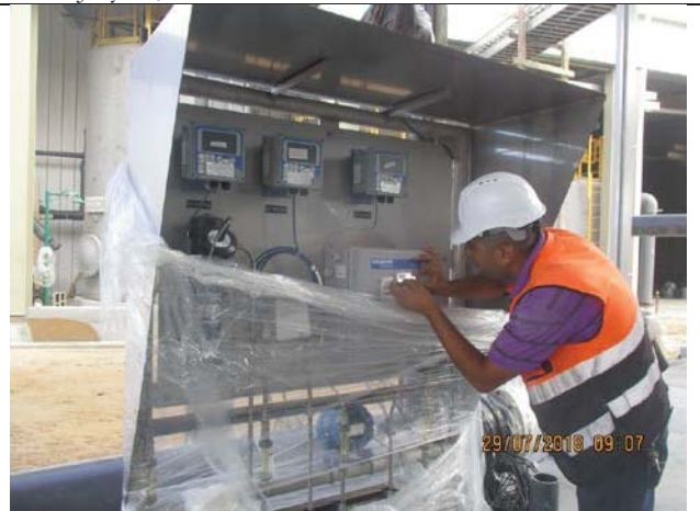
Photo No.36: Electrical works for instrumentation in pretreatment area. Date: July 29, 2018
