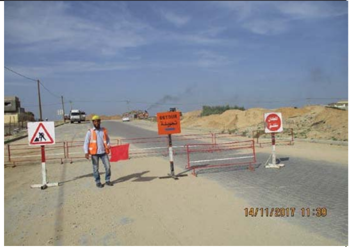
Photo No. 18: Intake pipe line construction activity. Date: November 14, 2017
