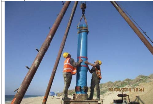
Photo No.21: Casing installation for beach well No.1 Date: April 16, 2018
