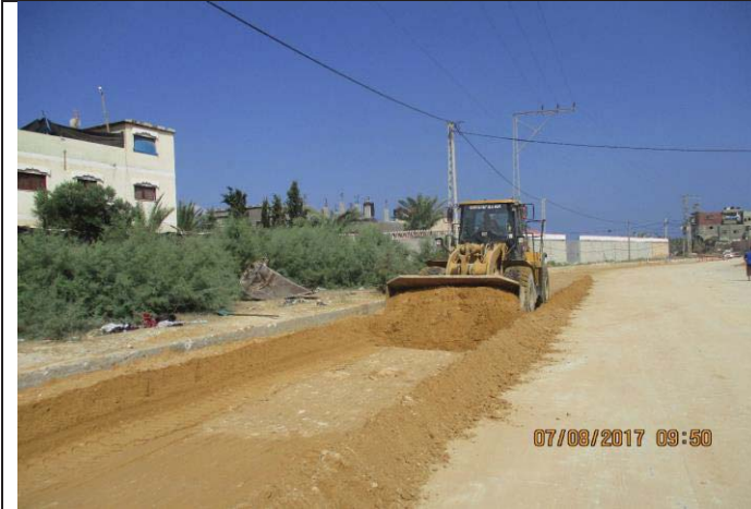
Photo No.19: Pipeline construction activities (backfilling the trench). Date: August 07, 2017
