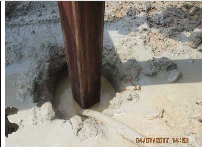
Photo No.07: Drilling piles using Bentonite. Date: July 04, 2017
