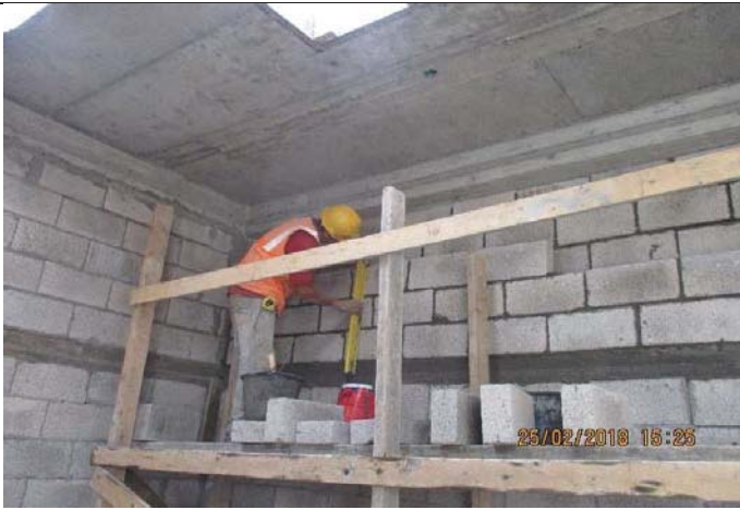
Photo No.37: Continue masonry works for electrical room walls. Date: February 25, 2018.
