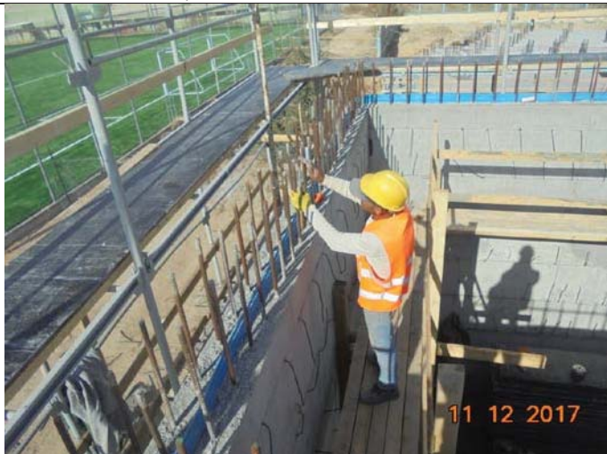
Photo No.23: Internal Formwork at raw water & backwash tanks. Date: December 11, 2017
