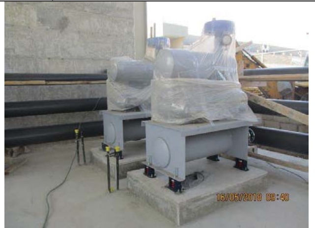
Photo No.16: Blowers installation inside pretreatment area Date: May 16, 2018
