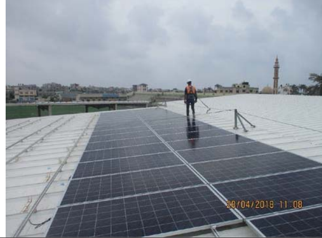
Photo No.39: PV panels installation for generator canopy Date: April 28, 2018
