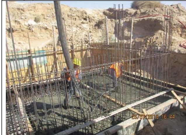
Photo No.33: Casting concrete for the electrical room pad Date: July 26, 2018
