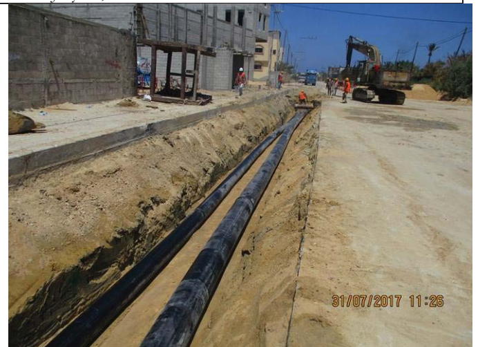
Photo No.40: HDPE pipeline welding. Date: July 30, 2017
