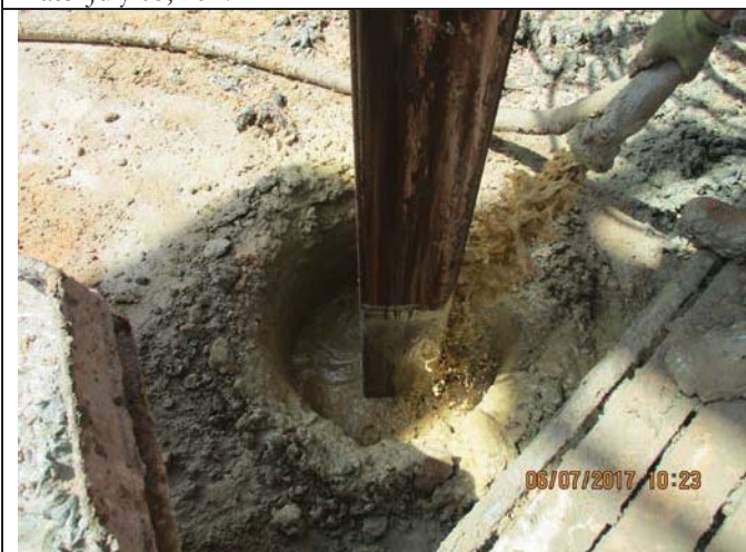
Photo No.11: Drilling piles using Bentonite. Date: July 06, 2017
