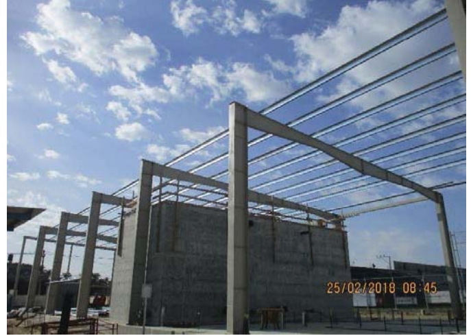
Photo No.34: Continue erection works for pretreatment steel structure Date: February 25, 2018
