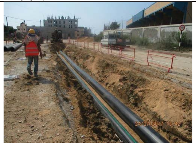
Photo No.36: Installation of 450 mm & 315 mm HDPE pipes. Date: July 24, 2017
