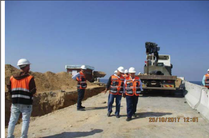
Photo No.47: Outfall pipeline construction activity (crossing Al-Rasheed Road) Date: October 25, 2017
