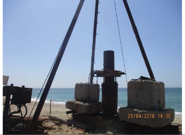
Photo No.40: Start works in beach well No.2 Date: April 29, 2018
