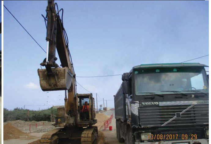
Photo No.32: Pipeline construction activity (trench excavation). Date: August 13, 2017
