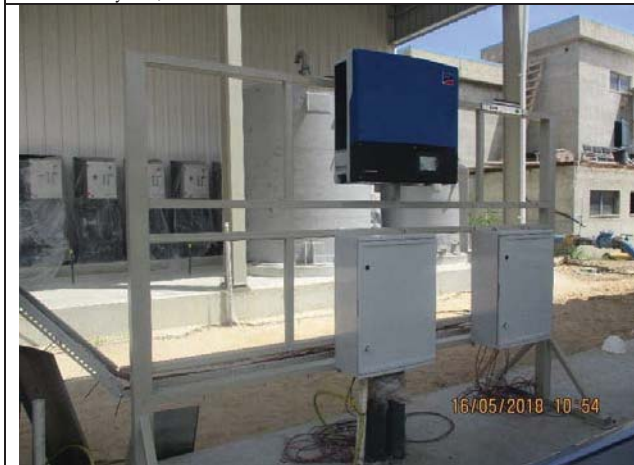
Photo No.17: PVC system installation Date: May 16, 2018
