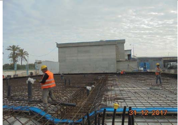
Photo No.52: Water stop installation for RO Building Date: December 31, 2017
