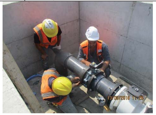
Photo No.16: Manifold installation works for beach wells Date: September 13, 2018
