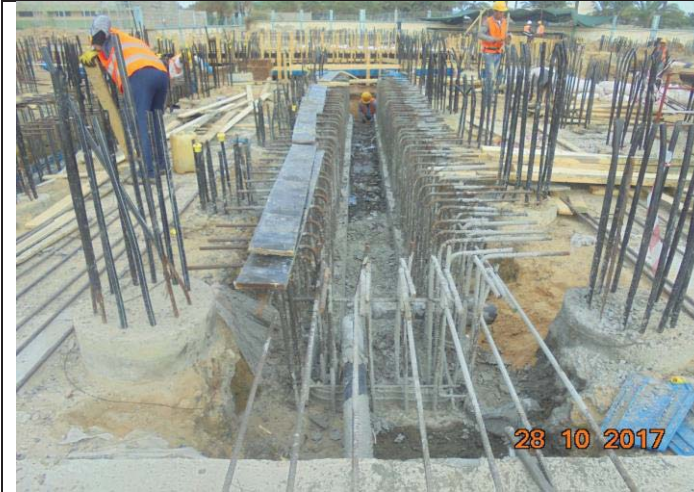
Photo No.55: Pre-treatment building trench formwork and steel reinforcing Date: October 28, 2017
