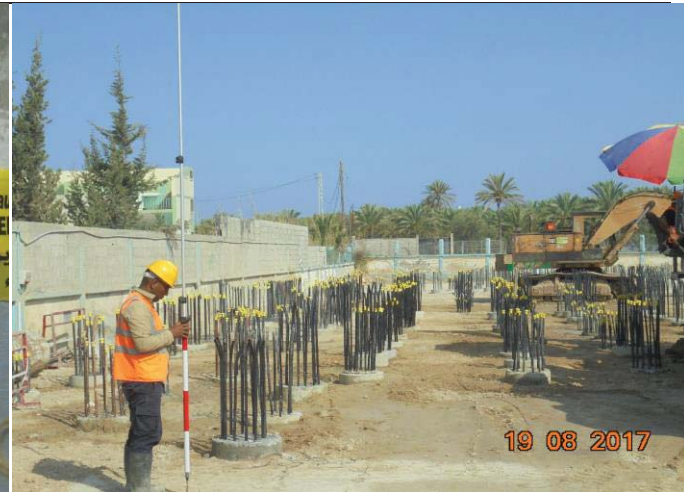
Photo No.38: Pile construction activity (pile locating). Date: August 17, 2017
