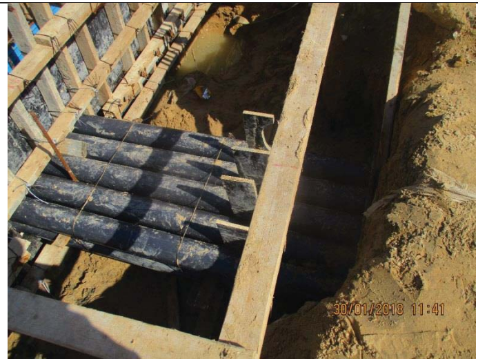
Photo No.40: Electrical conduits installation for generator pad trench.
