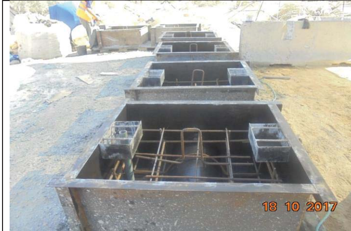
Photo No.37: Construction of weight collars for outfall pipeline. Date: October 18, 2017
