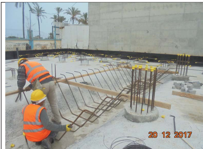
Photo No.41: Steel reinforcement for RO building foundation Date: December 20, 2017
