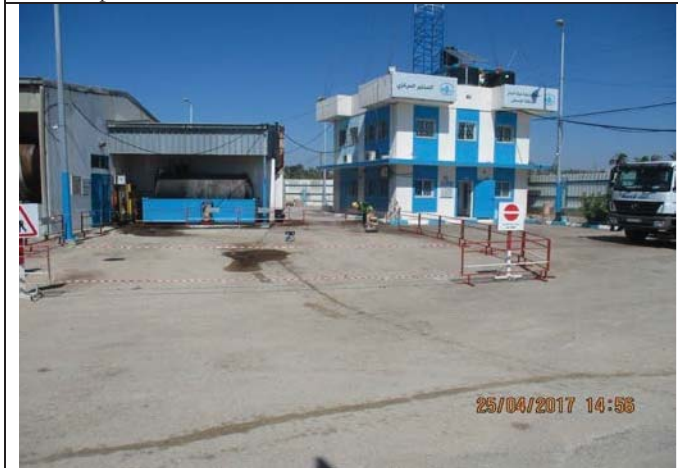
Photo No.19: Start fuel tank relocation activities.
