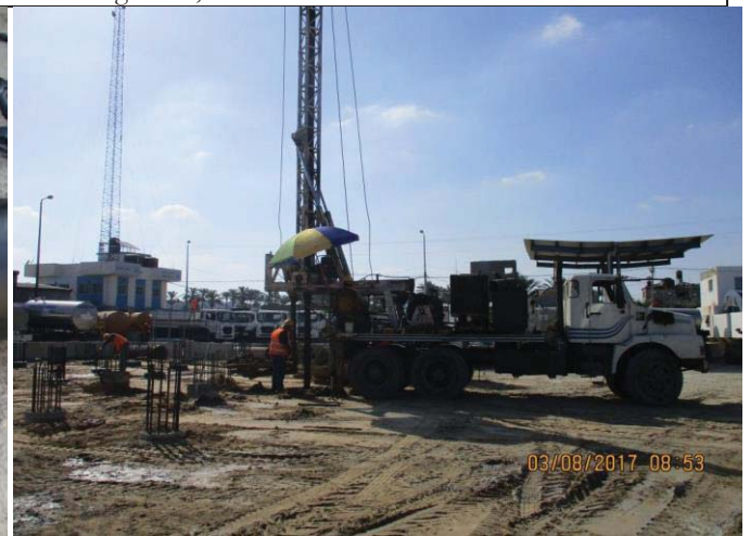
Photo No.12: Pile construction activity (generator pad). Date: August 03, 2017
