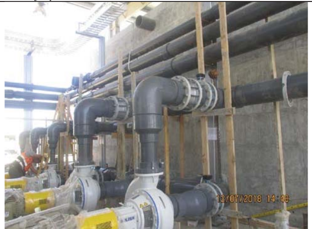
Photo No.18: Manifold installation works for feed pumps. Date: July 12, 2018
