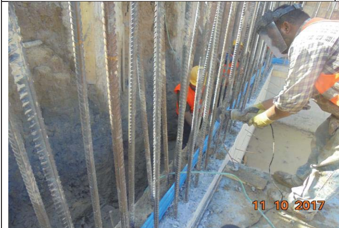
Photo No.17: Brine tank area - cleaning works. Date: October 11, 2017
