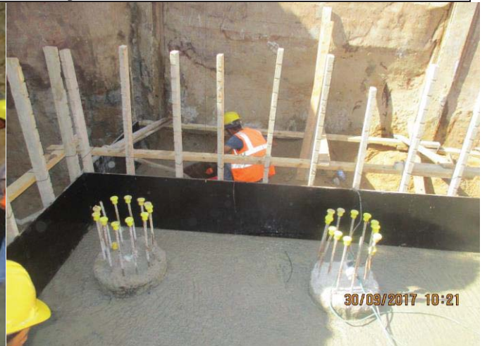
Photo No.40: Brine tank construction activity (Formwork at level -1.60) Date: September 30, 2017
