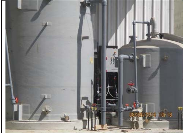
Photo No.13: CPVC pipes installation for chemical tanks Date: August 08, 2018
