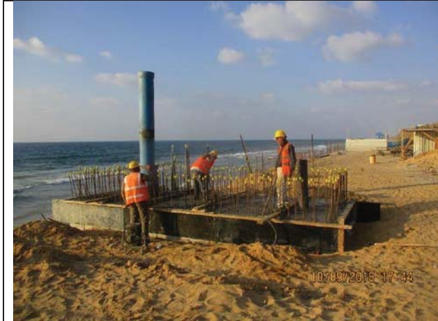
Photo No.13: Casting concrete pad of beach well No. 2 Date: September 10, 2018
