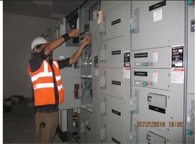
Photo No.09: Electrical works inside electrical room Date: July 07, 2018
