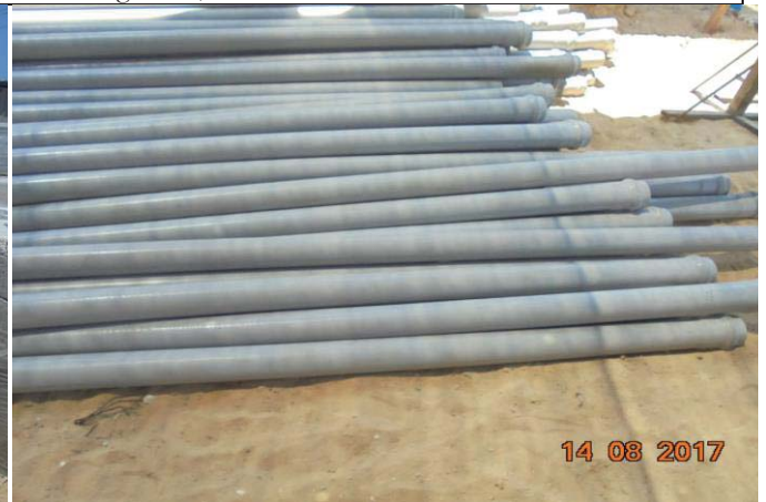
Photo No.36: Pipeline construction activity (electrical conduits) Date: August 15, 2017
