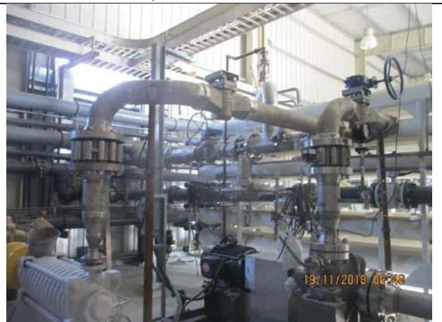
Photo No.10: Assembly works for high pressure pumps Date: November 19, 2018
