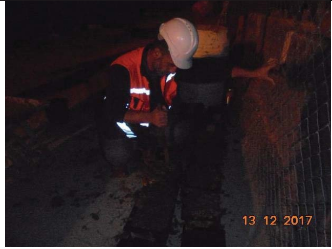
Photo No.30: Concrete quality control field test. Date: December 13, 2017
