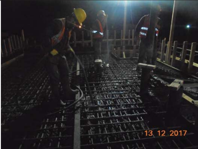
Photo No.29: Raw water & backwash tanks slab concrete casting. Date: December 13, 2017
