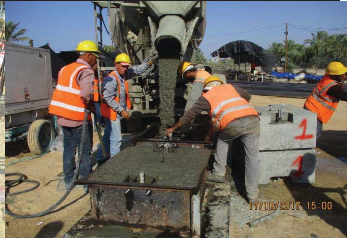
Photo No.34: Construction of weight collars for outfall pipeline. Date: October 17, 2017
