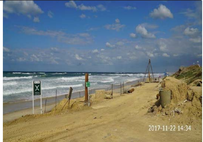
Photo No. 32: Beach well no 01 & 02 securing Date: November 22, 2017
