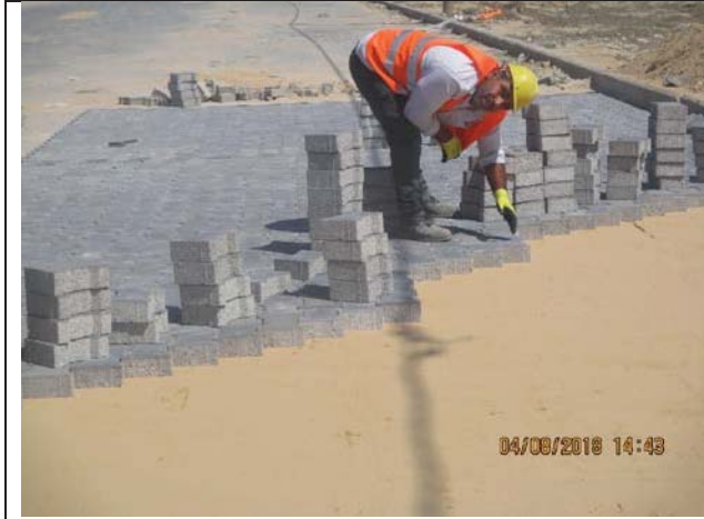
Photo No.07: Reinstatement works from St. 1 +500 to St. 1+550 Date: August 04, 2018
