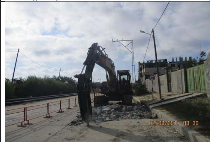
Photo No.09: Continue pipeline preparation – demolish road concrete surface. Date: August 02, 2017
