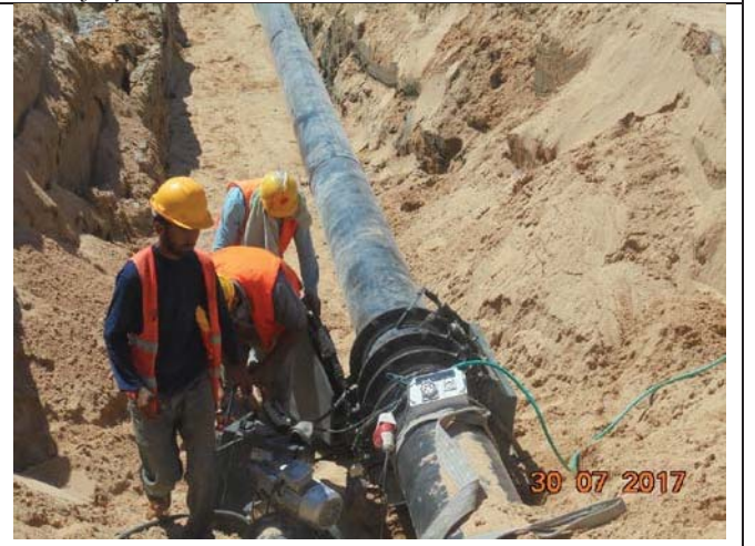
Photo No.40: HDPE pipeline welding. Date: July 30, 2017
