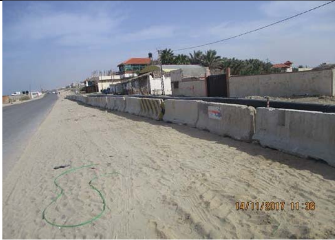
Photo No. 17: Intake pipe line construction activity. Date: November 14, 2017
