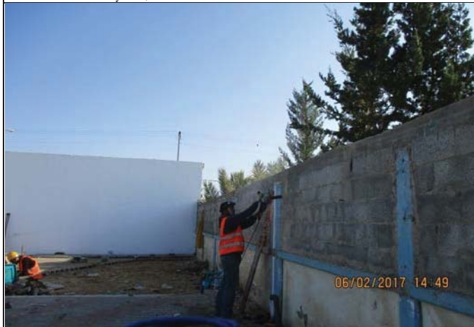
Photo No.07: Continue demolition works of existing steel canopy structure.
