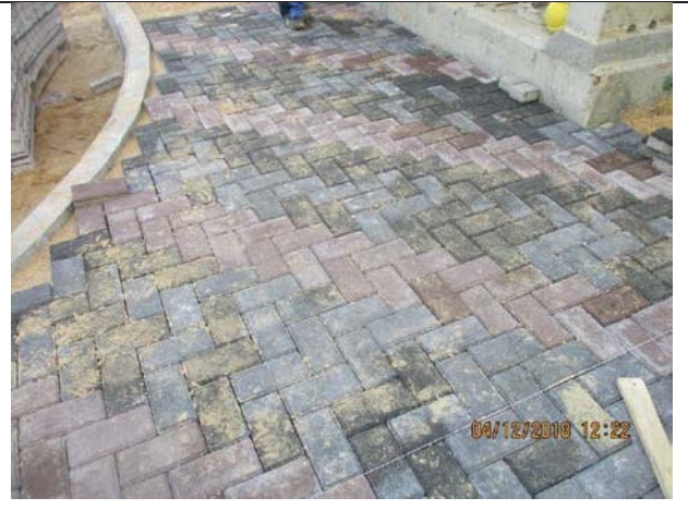
Photo No.04: Start tiling works inside yard Date: December 04, 2018
