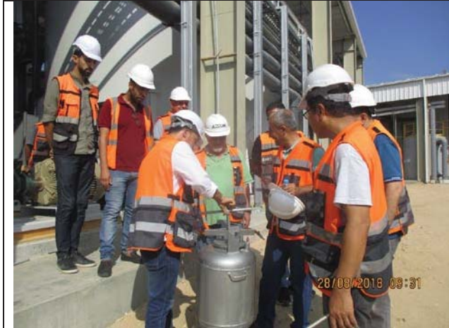
Photo No.25: Grouting injection pump Date: August 28, 2018
