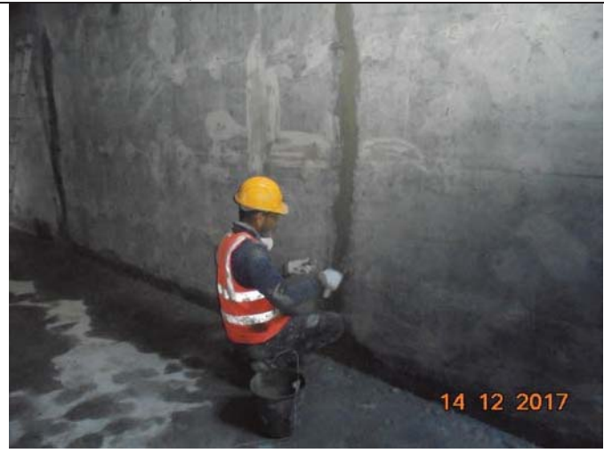
Photo No.32: Brine tank leak points repair works Date: December 14, 2017
