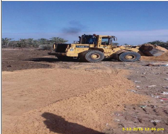
Photo No.03: Storage yard leveling works Date: December 03, 2016
