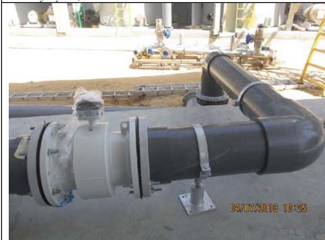
Photo No.05: Fittings installation for brine manifold Date: July 04, 2018
