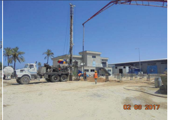
Photo No.08: Pile construction activity (generator pad). Date: August 02, 2017
