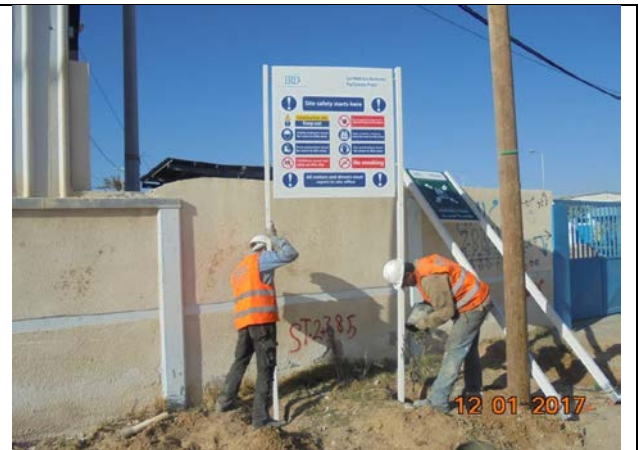
Photo No.02.I: Installation of temporary safety signs. Date: January 12, 2017
