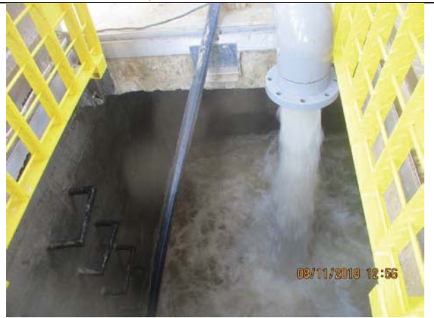
Photo No.04: Start flushing for the intake pipeline Date: November 08, 2018
