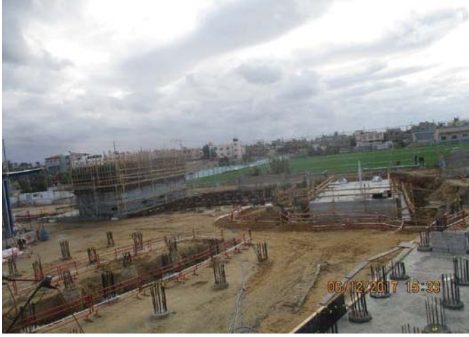
Photo No.13: No site activities – heavy rain Date: December 06, 2017
