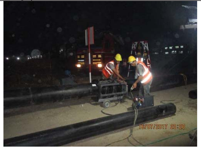
Photo No.22: HDPE pipes welding activity Date: July 16, 2017
