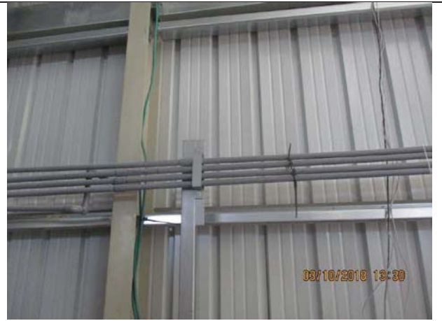
Photo No.02: Piping steel support installation in RO area. Date: October 03, 2018
