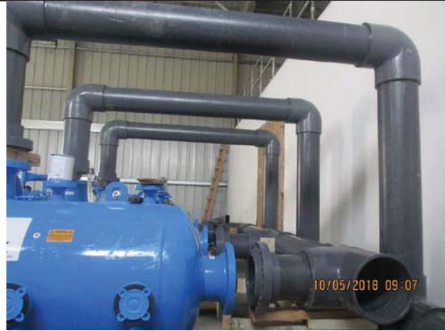
Photo No.11: Mechanical installation inside RO building. Date: May 10, 2018
