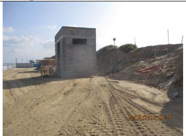
Photo No.28: Block works for beach well electrical room. Date: August 30, 2018
