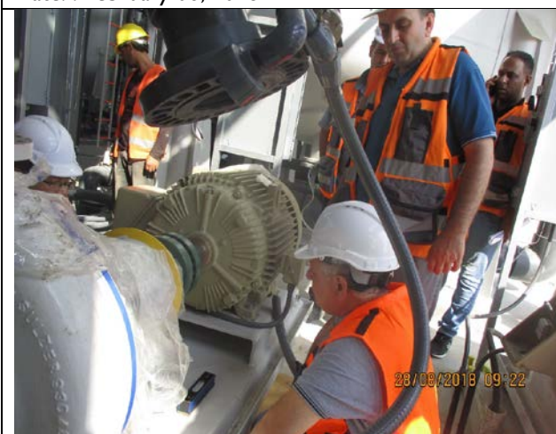
Photo No.15.2: Blumont technical expert inspecting alignment and leveling works. Date: August 28, 2018
