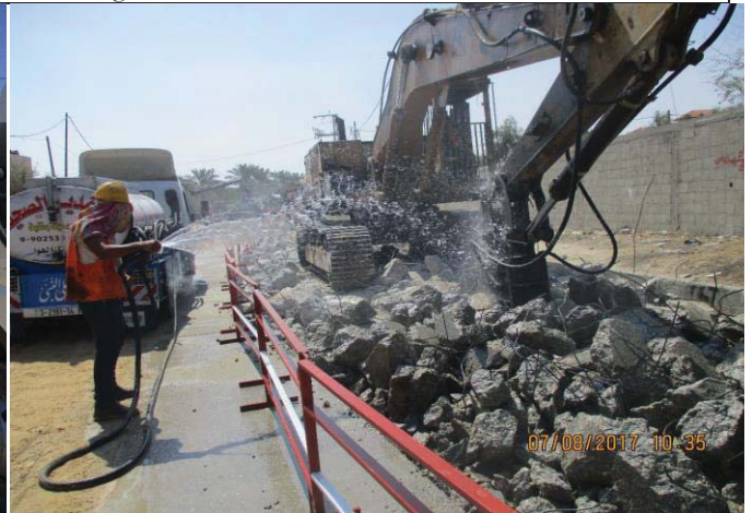
Photo No.22: Continue pipeline preparation – demolish road concrete surface. Date: August 07, 2017
