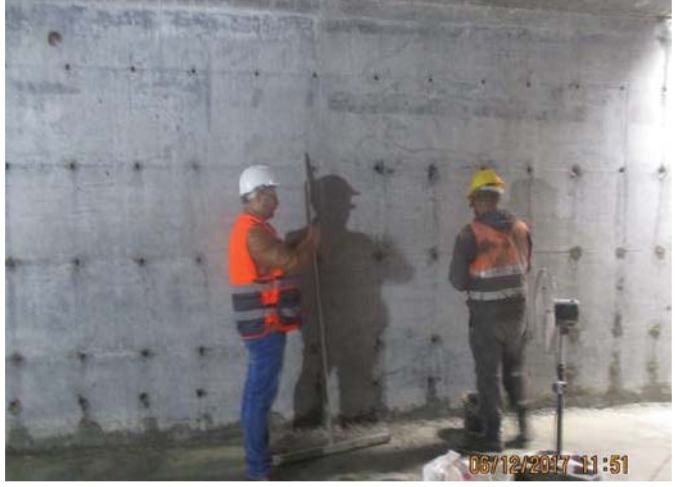
Photo No.14: Brine tank internal repair works progress Date: December 06, 2017
