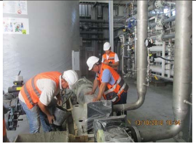
Photo No.08: Grouting for 2 nd pass feed pumps. Date: October 13, 2018
