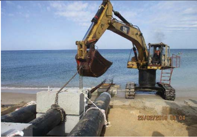
Photo No.35: Experimental works for outfall pipeline installation Date: February 25, 2018
