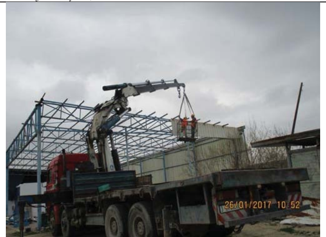
Photo No.08: Demolition of existing steel canopy structure. Date: January 26, 2017
