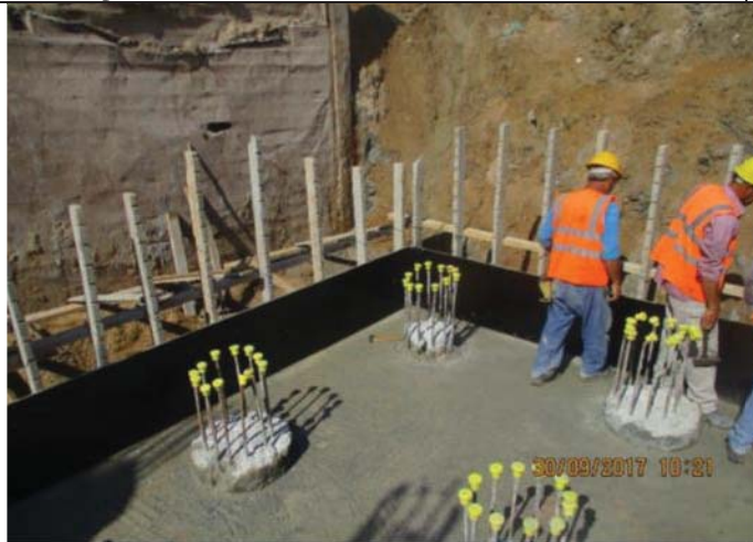
Photo No.39: Brine tank construction activity (formwork at level -1.60) Date: September 30, 2017
