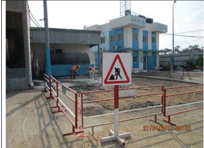
Photo No.23: Continue fuel tank relocation activities Date: April 27, 2017
