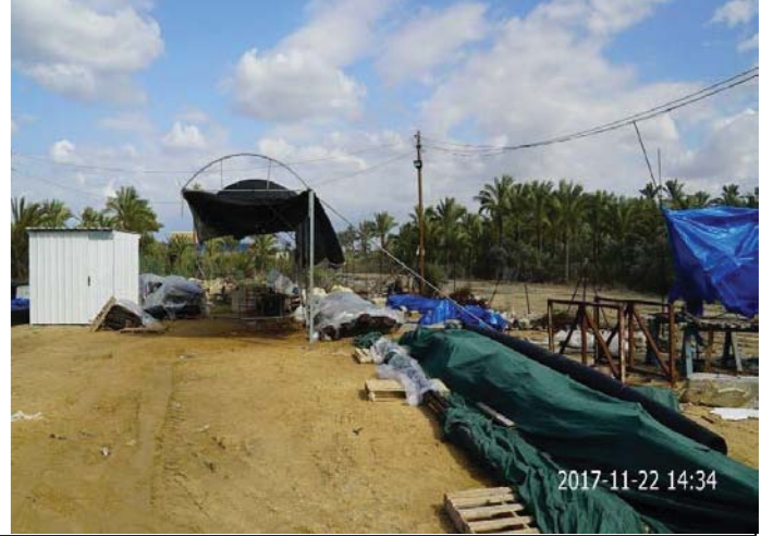
Photo No. 36: Steel rebar storing and securing Date: November 22, 2017
