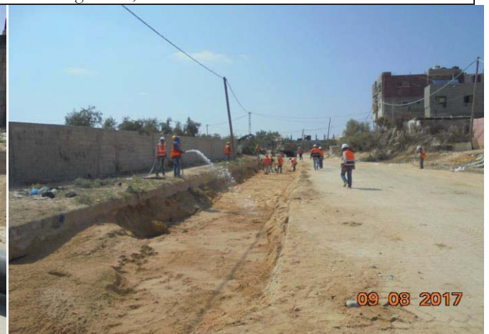
Photo No.28: Pipeline construction activities (backfilling on layers & watering). Date: August 09, 2017
