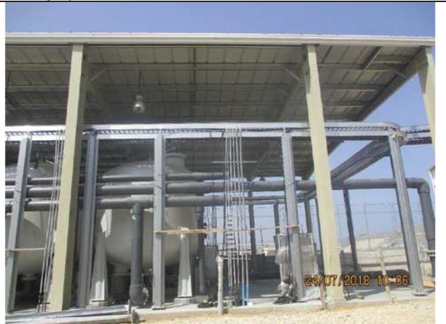
Photo No.28: Extending cables for pretreatment area Date: July 24, 2018
