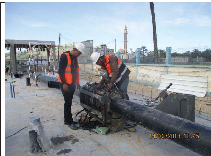
Photo No.21: HDPE pipes welding to install for the existing raw water tank Date: February 14, 2018
