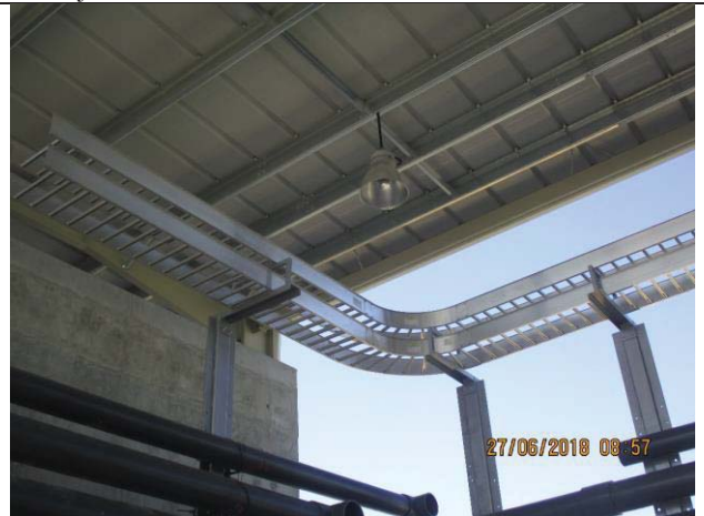
Photo No.30: Installing cable ladder in pretreatment area Date: June 27, 2018
