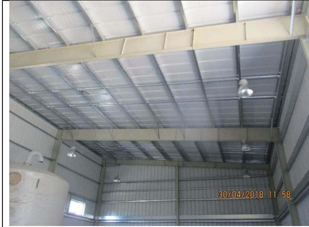
Photo No.43: Start electrical installation inside RO building. Date: April 30, 2018
