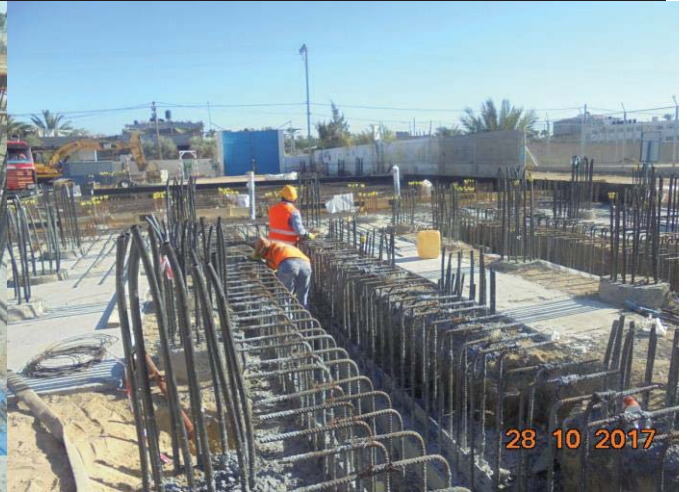
Photo No.56: Pre-treatment building trench formwork and steel reinforcing. Date: October 28, 2017
