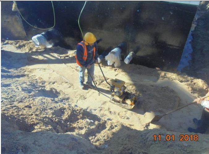
Photo No.13: brine tank backfilling and compaction works. Date: January 11, 2018
