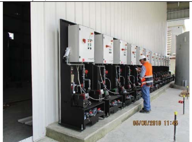
Photo No.06: Chemical dosing skids installation in RO building. Date: May 05, 2018
