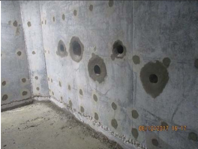
Photo No.15: Brine tank internal repair works. Date: December 06, 2017
