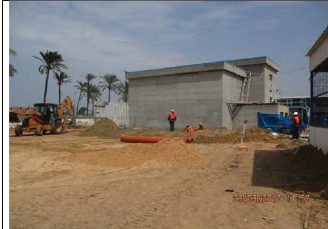
Photo No.23: Brine line relocation activities.
