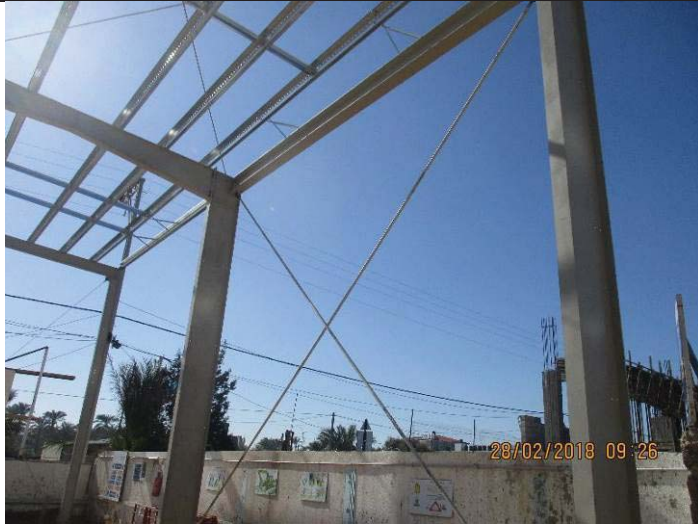
Photo No.41: Continue erection works for pretreatment steel structure Date: February 28, 2018
