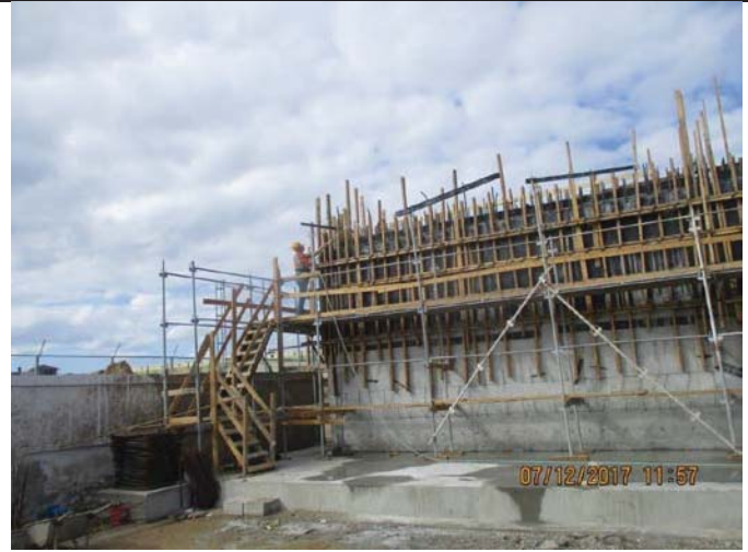
Photo No.16: Curing previously casted walls at raw water and backwash tanks Date: December 07, 2017
