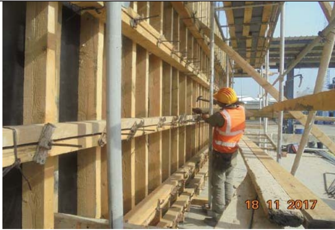
Photo No. 19: Raw water and backwash tanks formwork. Date: November 18, 2017
