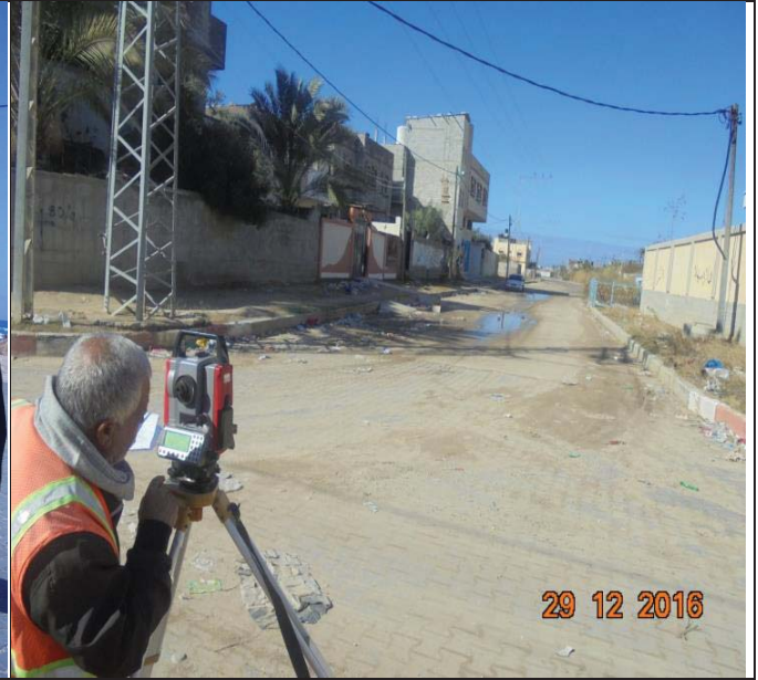
Photo No.18: Locating bench marks Date: December 29, 2016
