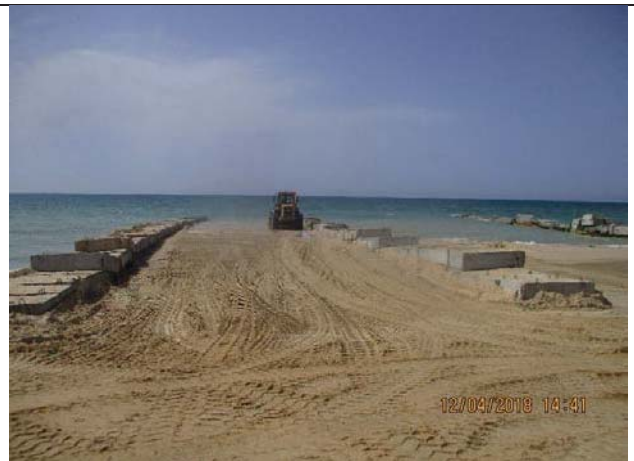
Photo No.18: Preparation works for outfall pipeline installation. Date: April 12, 2018
