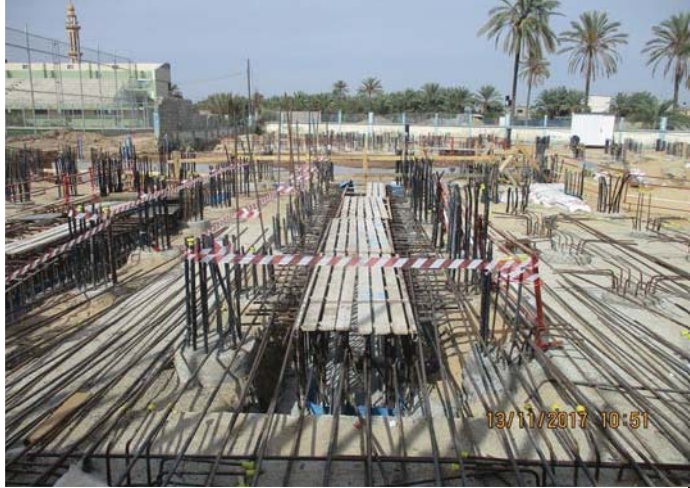
Photo No. 14: brine tank slab (curing casted slab).
