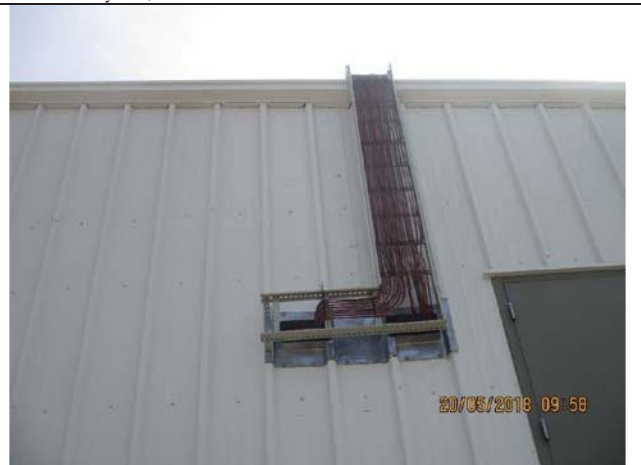
Photo No.18: Electrical cables installation inside RO building Date: May 20, 2018
