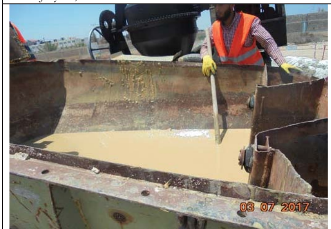
Photo No.05: Bentonite mixing. Date: July 03, 2017
