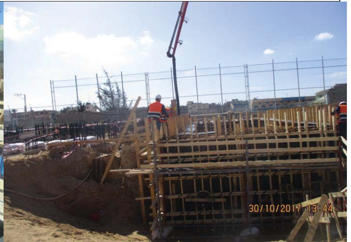
Photo No.58: Tank construction activities - walls casting. Date: October 30, 2017
