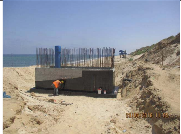
Photo No.32: Insulation works for retaining walls. Date: June 28, 2018
