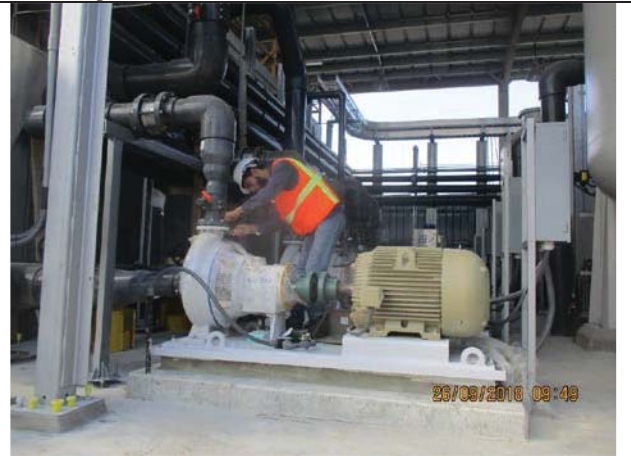
Photo No.28: Piping works for pumps. Date: September 26, 2018
