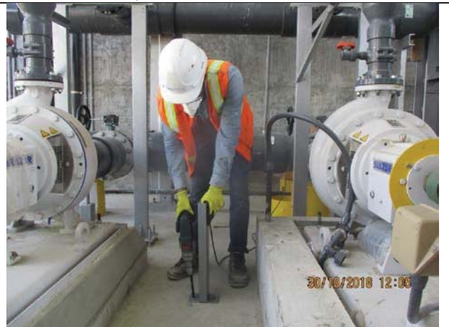
Photo No.18: Pipe support installation in pretreatment area Date: October 30, 2018
