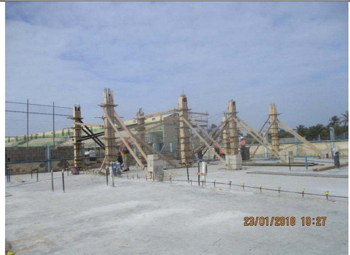
Photo No.30: Steel reinforcement and formwork for electrical room columns.
