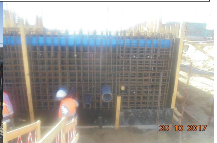
Photo No.54: Continue brine tank construction activities - thimbles installation. Date: October 29, 2017
