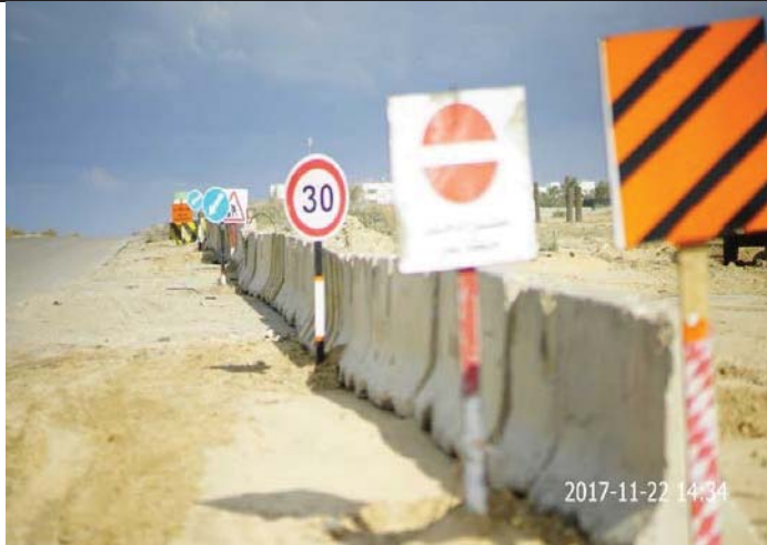
Photo No. 31: Concrete barriers installation & signs installation. Date: November 22, 2017
