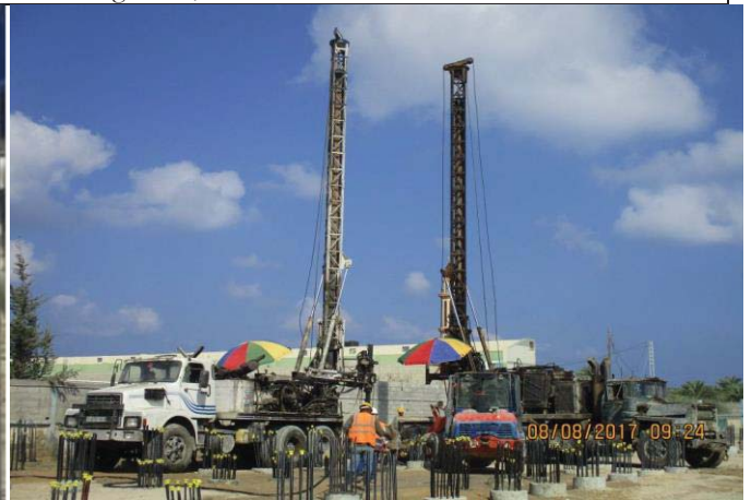
Photo No.24: Pile construction activities (pre-treatment & brine tank). Date: August 08, 2017
