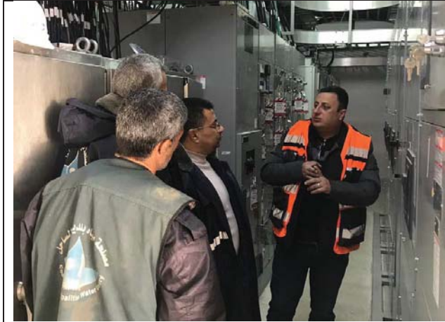
Photo No.07: Onsite training for PWA staff for " VFD" Date: January 09, 2019
