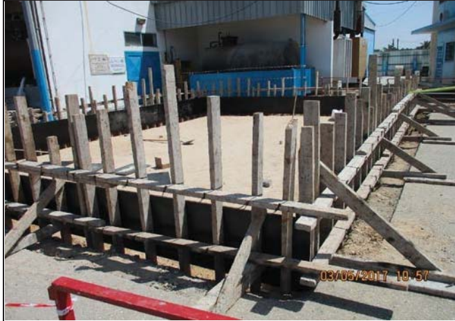
Photo No.01: Fuel tank relocation activities Date: May 03, 2017
