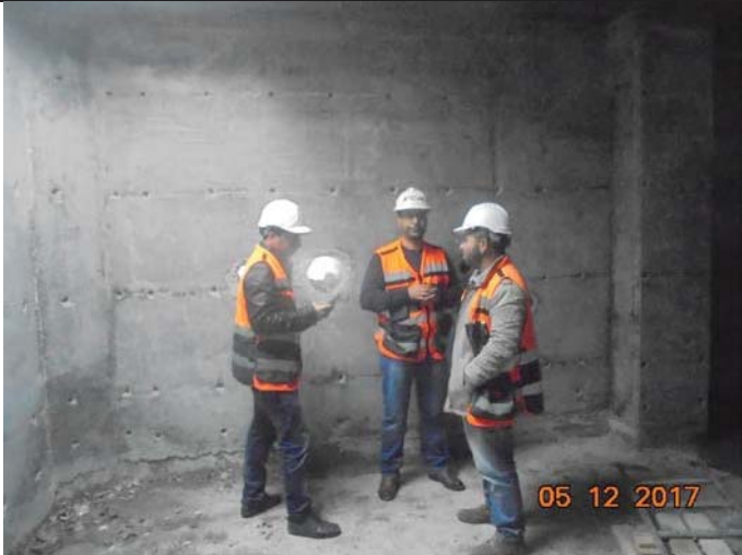
Photo No.11: Brine tank internal preparation works for repair Date: December 05, 2017
