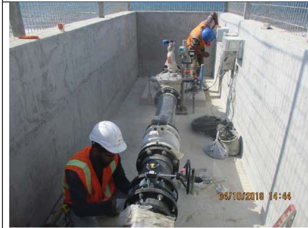
Photo No.03: Mechanical works in beach wells Date: October 04, 2018
