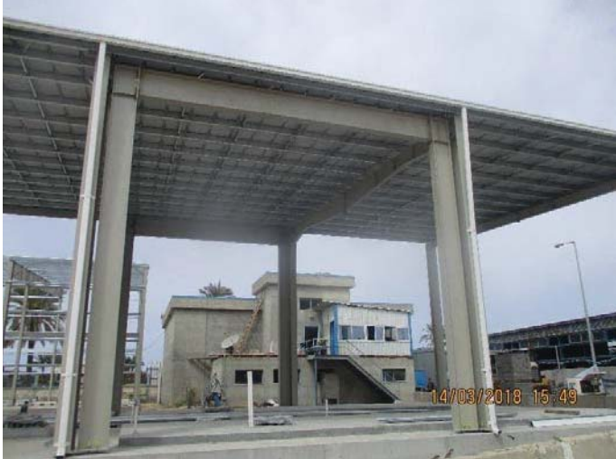
Photo No.11: Generator steel structure Date: March 14, 2018
