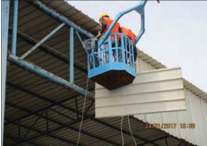
Photo No.05: Start demolition of existing canopy steel structure Date: January 24, 2017
