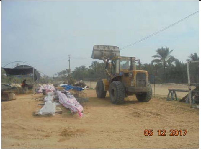
Photo No.12: Idle equipment on site Date: December 05, 2017
