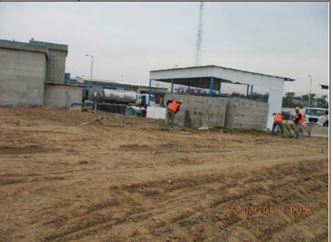
Photo No.20: Site cleaning & housekeeping Date: February 22, 2017
