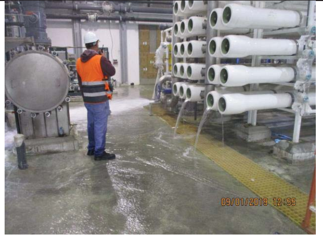
Photo No.08: Flushing of RO vessels Date: January 09, 2019
