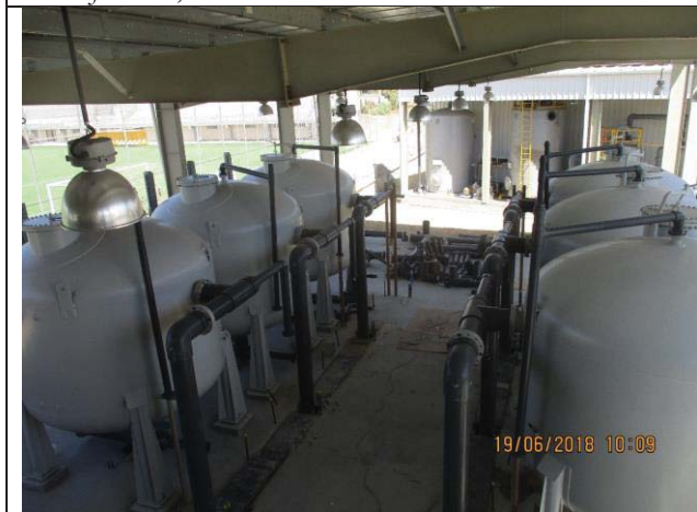
Photo No.17: Pretreatment area Date: June 19, 2018
