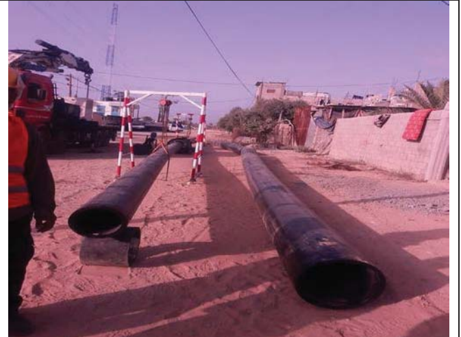
Photo No.16: HDPE pipes welding activity Date: July 13, 2017
