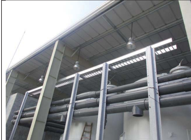
Photo No.25: Installing cable ladder in pretreatment area Date: June 24, 2018
