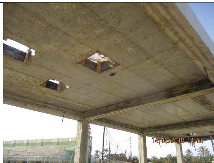
Photo No.22: De-shuttering works for electrical room roof slab Date: February 14, 2018
