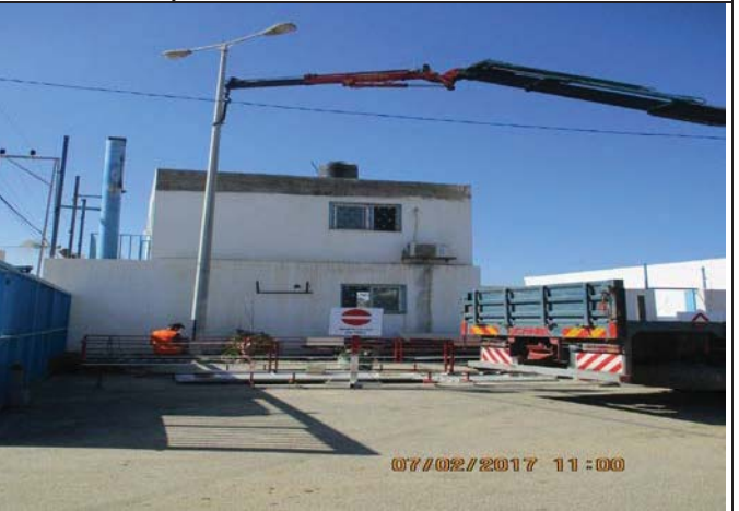
Photo No.10: Demolition of existing electrical lighting poles.
