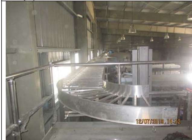
Photo No.17: Cable tray installation in RO building Date: July 12, 2018
