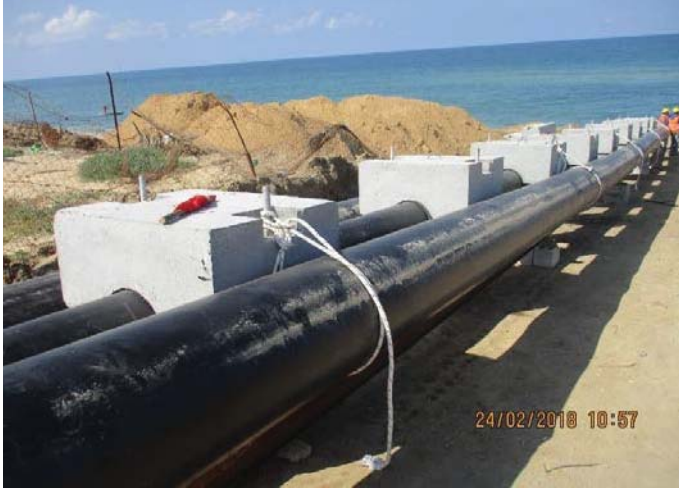
Photo No.33: Preparation works for outfall pipeline installation Date: February 24, 2018
