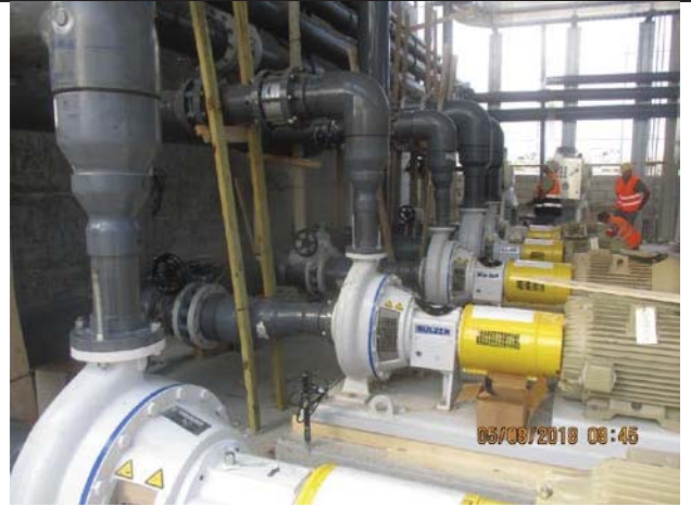
Photo No.08: Leveling works for pumps Date: August 05, 2018
