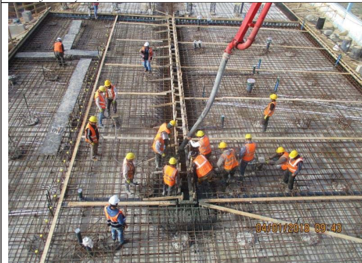
Photo No.03: Casting concrete for RO building foundation (phase 01). Date: January 04, 2018
