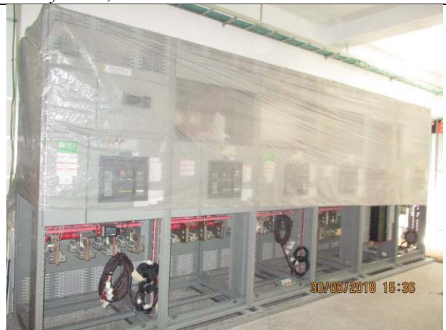
Photo No.36: Finalize the SWBD bus bars Connections Date: June 30, 2018
