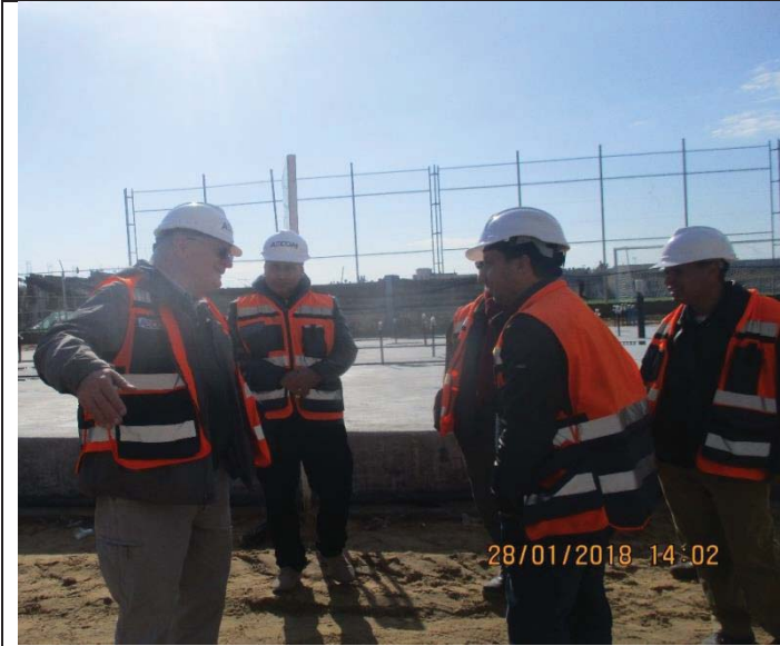
Photo No.37: AECOM visitors at construction site.
