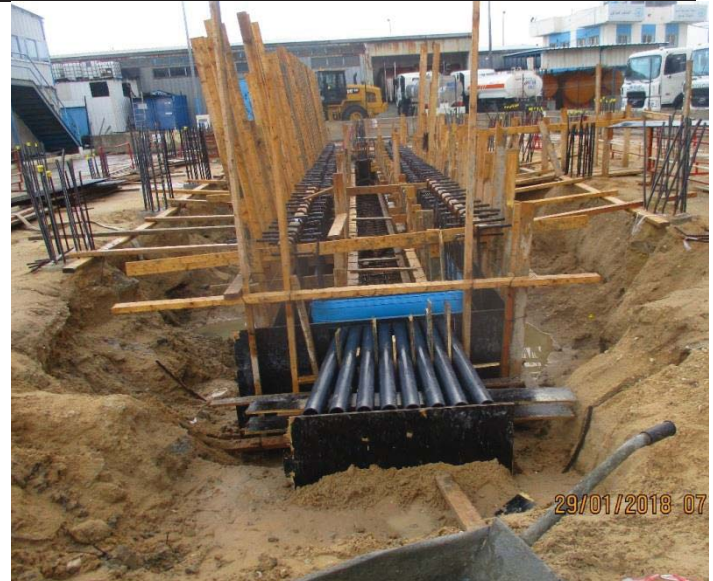
Photo No.38: Electrical conduits installation for generator pad trench.
