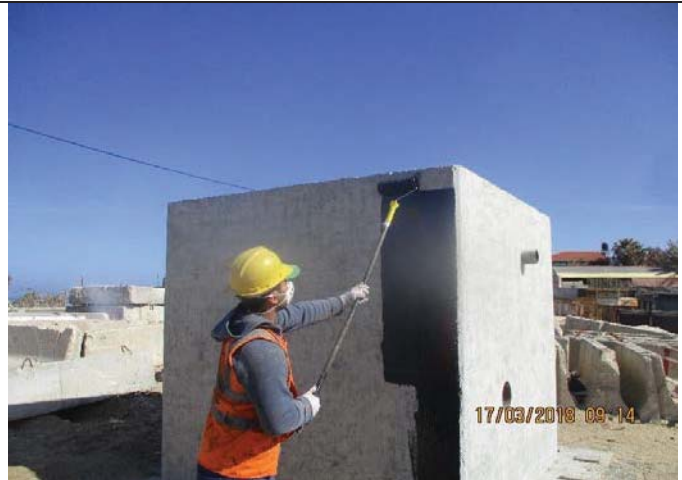
Photo No.14: Epoxy coating for mechanical chambers. Date: March 17, 2018
