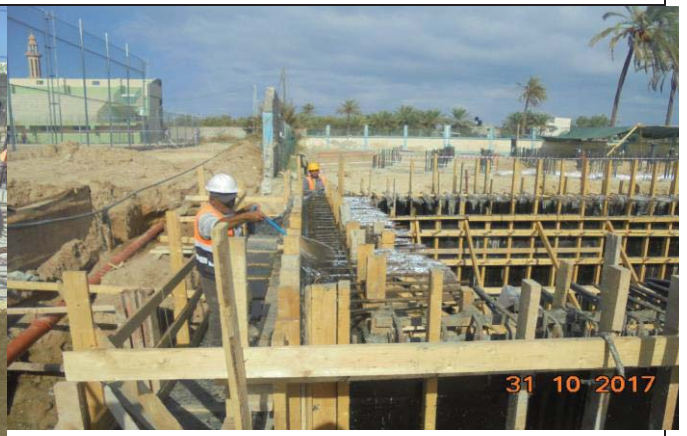
Photo No.60: Brine tank casted walls curing. Date: October 31, 2017
