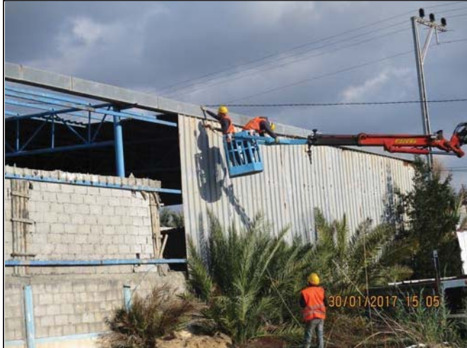
Photo No.11: Demolition of existing steel canopy structure. Date: January 30, 2017
