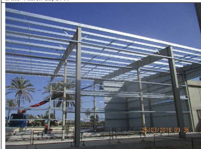
Photo No.25: Continue working on RO building walls. Date: March 26, 2018
