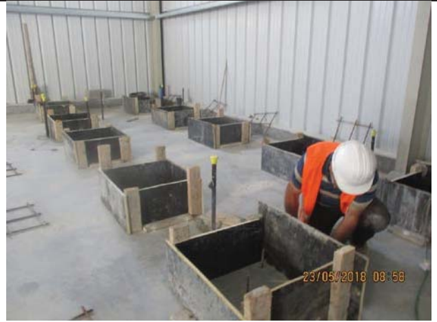
Photo No.20: Formwork for pads inside RO building. Date: May 23, 2018
