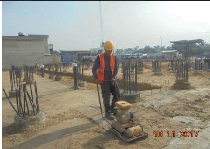
Photo No. 21: Leveling works at R.O building area. Date: November 18, 2017
