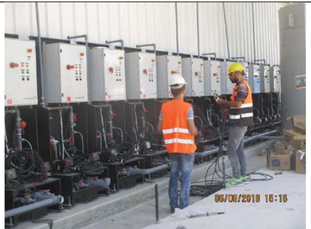
Photo No.10: Electrical works for chemical skids Date: August 06, 2018
