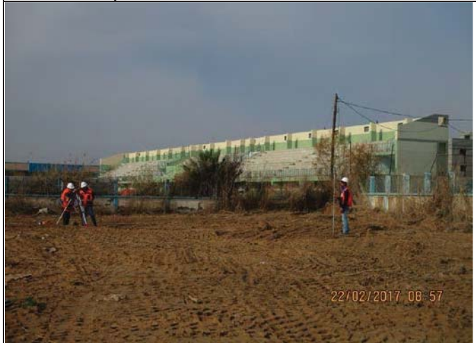
Photo No.19: Grid survey for pretreatment and RO buildings Date: February 22, 2017
