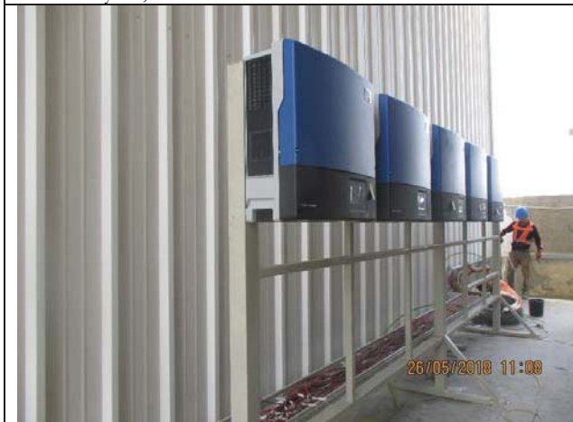
Photo No.23: PV system canopy installation for pretreatment area Date: May 26, 2018
