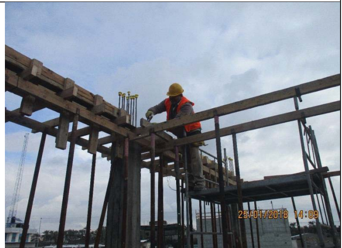
Photo No.34: Start formwork for electrical room roof slab. Date: January 25, 2018
