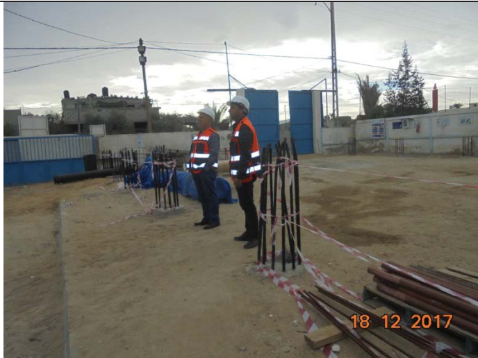
Photo No.37: USAID Representative at construction site. Date: December 18, 2017
