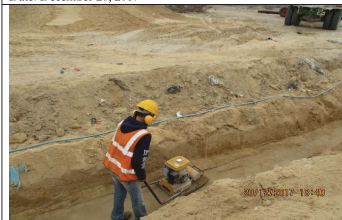
Photo No.43: Backfill and compaction works for intake pipeline Date: December 20, 2017
