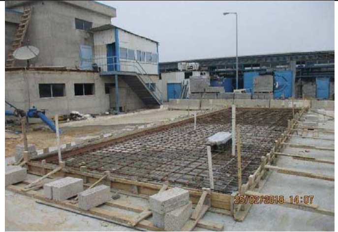
Photo No.36: Formwork for the pads on generator pad. Date: February 25, 2018
