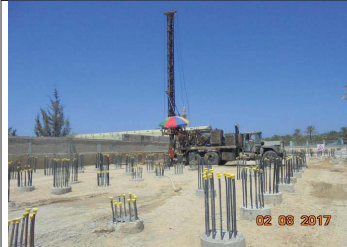
Photo No.07: Pile construction activity (brine tank). Date: August 02, 2017
