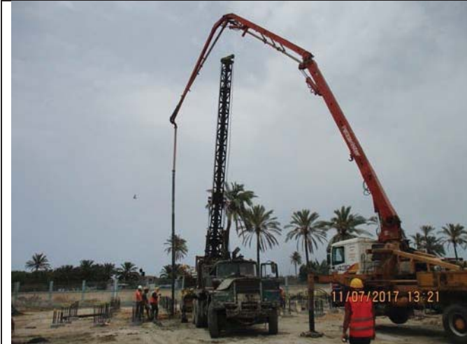
Photo No.13: Pile construction activities-Piles casting Date: July 11, 2017
