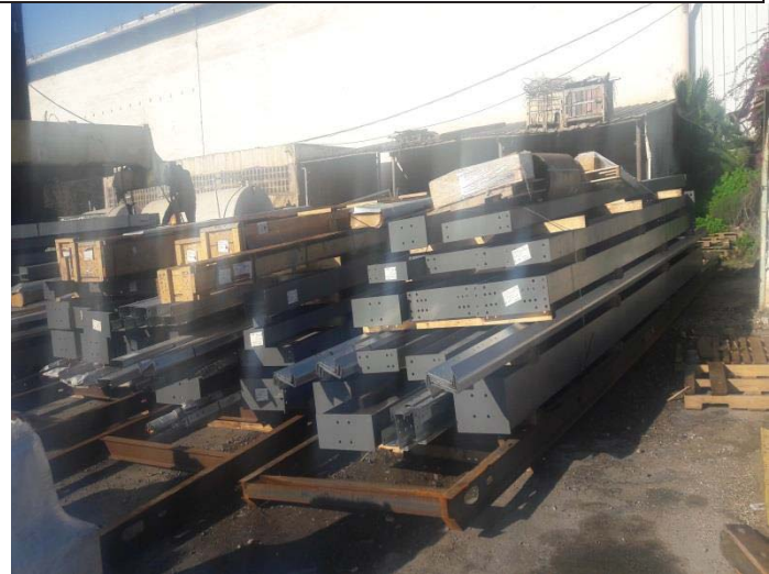
Photo No.44: Delivery of Pre-engineered steel structures. Date: January 30, 2018
