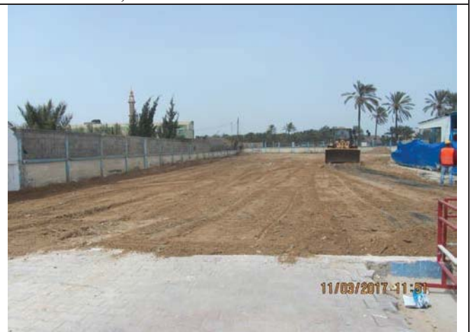
Photo No.04: Site leveling and preparation prior to pile construction works.
