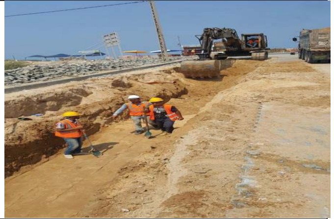
Photo No.44: Pipeline installation -trench excavation, bedding and preparation. Date: August 17, 2017.
