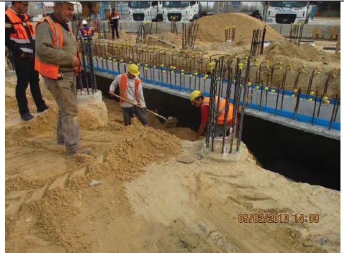
Photo No.08: Backfilling works around the generator pad trench Date: February 05, 2018
