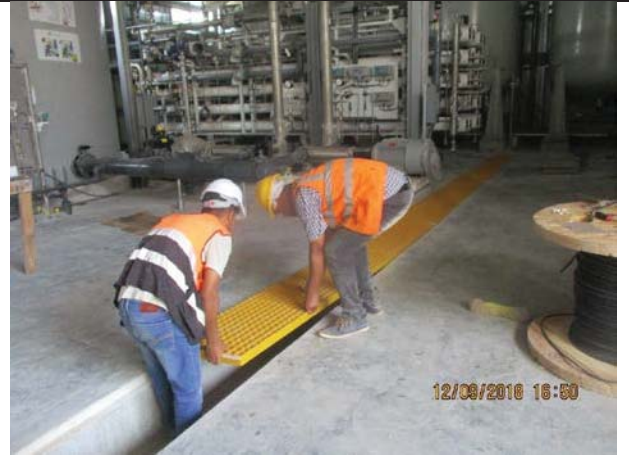
Photo No.14: Grating installation in RO Building (mockup sample) Date: September 12, 2018
