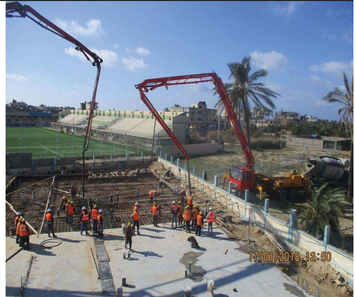
Photo No.22: Casting concrete for RO foundation (phase 2). Date: January 17, 2018
