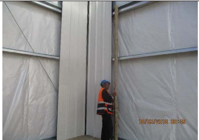
Photo No.16: Installation of walls panels for workshop area Date: March 18, 2018
