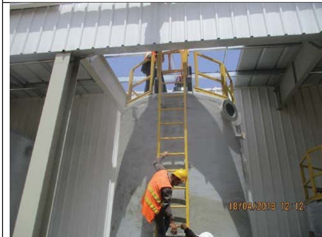
Photo No.23: Mixer installation Date: April 18, 2018
