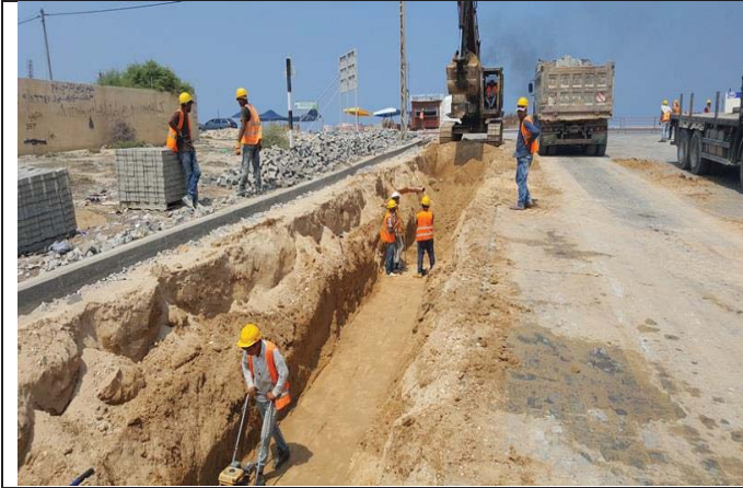
Photo No.43: Pipeline installation -trench excavation, bedding and preparation. Date: August 17, 2017
