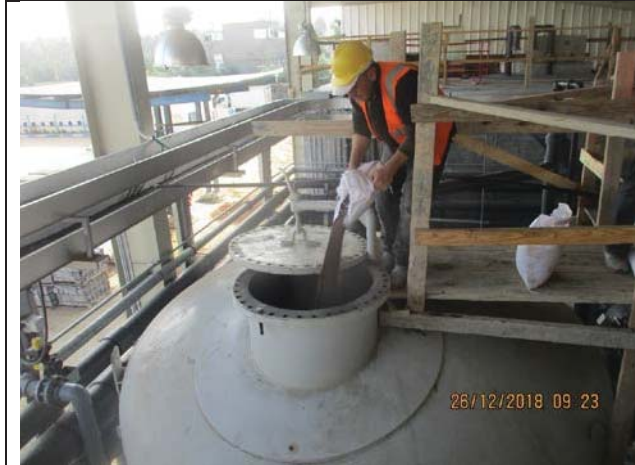
Photo No.25: Filling garnet inside dual media filter #4 Date: December 26, 2018
