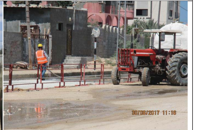
Photo No.72: Curing previously casted panels Date: August 30, 2017
