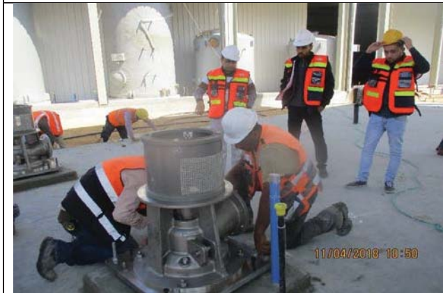
Photo No.15: Excavation works and installation of electrical manhole inside construction site Date: April 11, 2018
