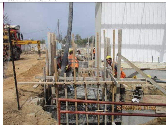
Photo No.28: Casting concrete for two electrical manholes. Date: March 28, 2018
