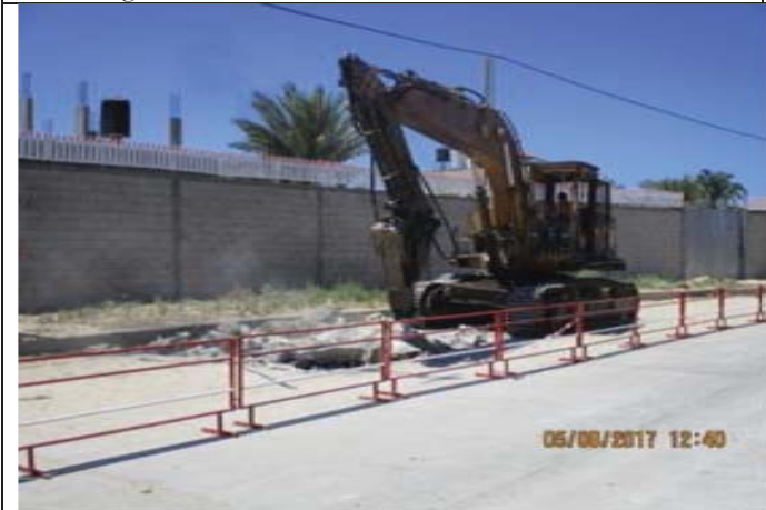
Photo No.15: Pipeline construction activity (demolish road concrete surface). Date: August 05, 2017
