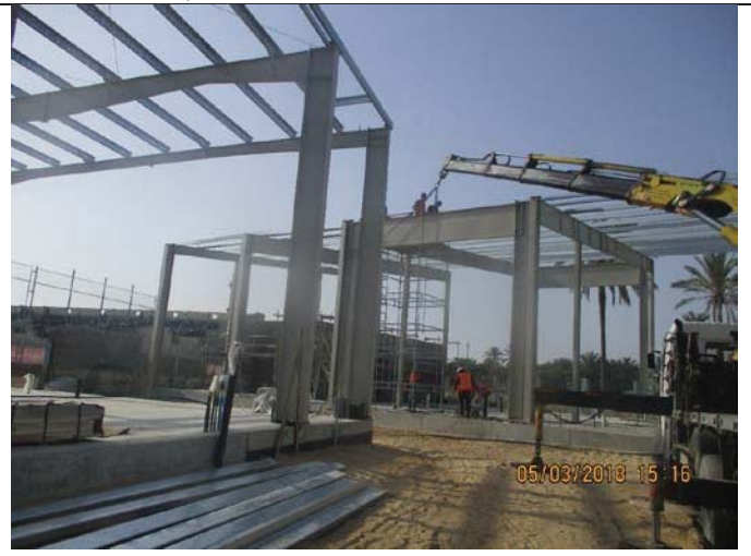
Photo No.04: Erection works for RO steel structure
