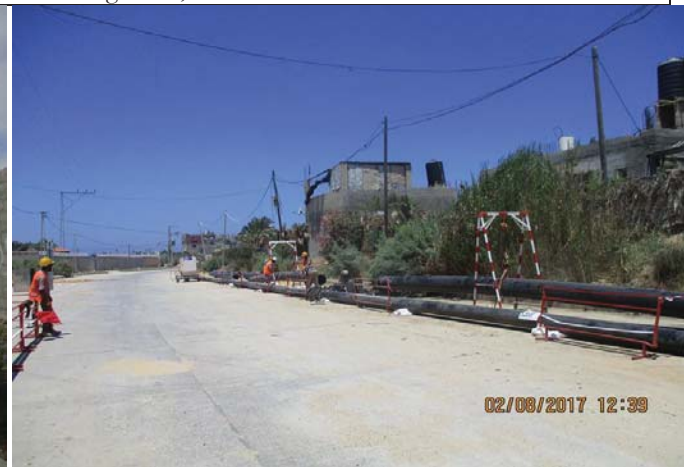
Photo No.10: Continue pipeline preparation – welding pipes (450 mm & 315 mm). Date: August 02, 2017
