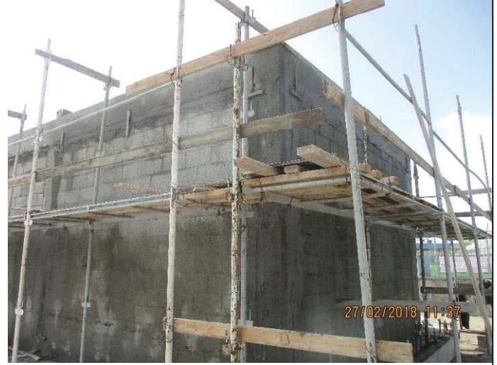
Photo No.40: Start plastering works for electrical room Date: February 27, 2018.
