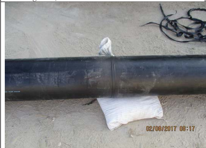
Photo No.11: HDPE pipe loading on sandy bags. Date: August 02, 2017
