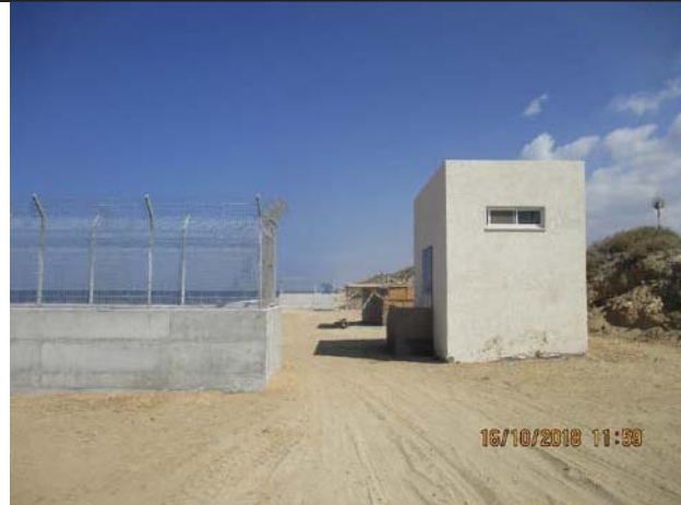
Photo No.09: Leveling works around beach pumps Date: October 16, 2018
