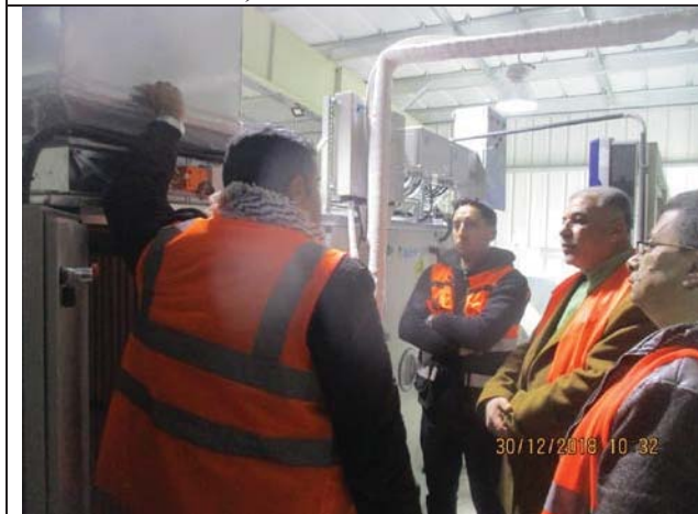
Photo No.29: Onsite training for PWA staff "HVAC system" Date: December 30, 2018
