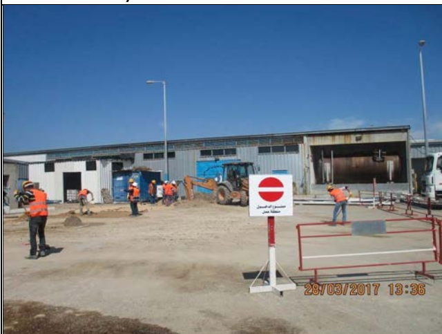
Photo No. 05.I: Housekeeping during brine line relocation activities. Date: March 28, 2017
