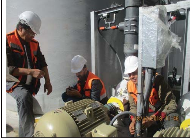
Photo No.19: Final alignment for pumps Date: December 18, 2018
