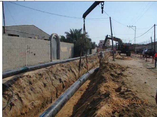
Photo No.29: Pipeline (outfall and intake) installation. Date: July 20, 2017
