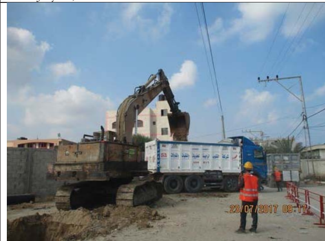
Photo No.35: Transfer excavation material to dumping site. Date: July 23, 2017
