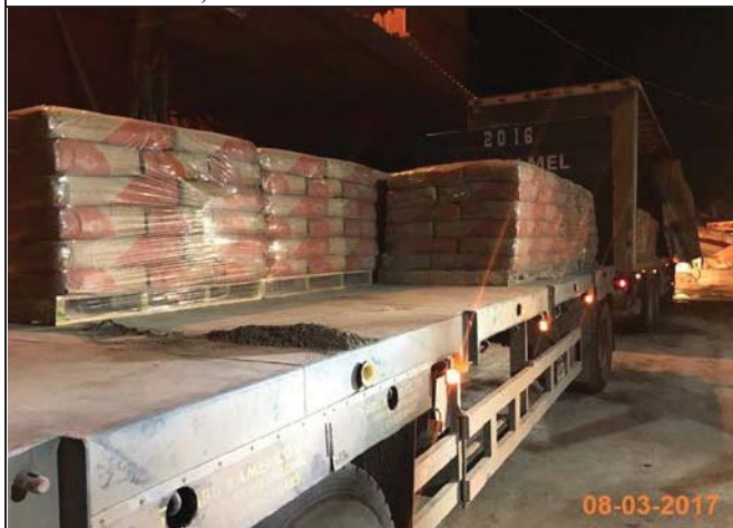
Photo No.03: Delivery of sulfate resistant cement (CEM I, 42.5N SR3) to AL Ta'awon batch plant /Gaza Strip through Tarqumia crossing point.
