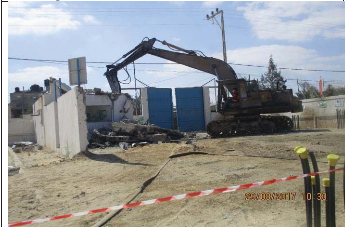
Photo No.71: Existing ICRC store demolition works. August 29, 2017
