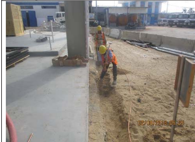
Photo No.03: Excavation works for grounding system Date: August 02, 2018
