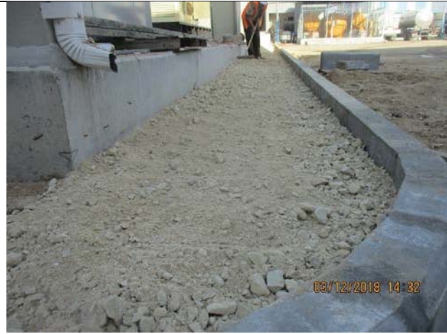
Photo No.03: Base course furnishing for tiles sidewalk. Date: December 03, 2018
