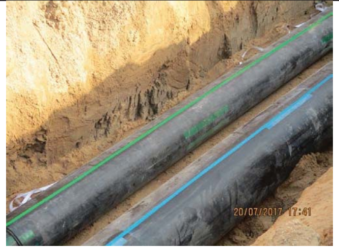
Photo No.32: Pipeline (outfall and intake) marking. Date: July 20, 2017
