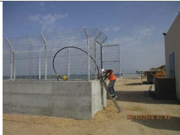
Photo No.17: Chlorination works for beach wells Date: October 25, 2018
