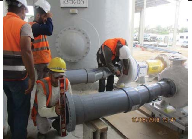
Photo No.14: Fabrication and installation works for PVC manifold. Date: May 12, 2018
