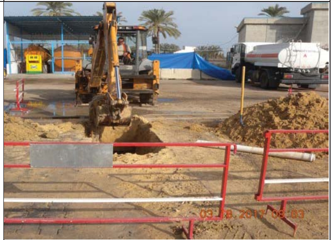
Photo No.14: Storm water catchment relocation. Date: March 18, 2017
