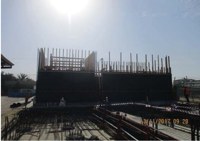
Photo No. 13: Raw water and backwash tanks formwork and steel formation.
