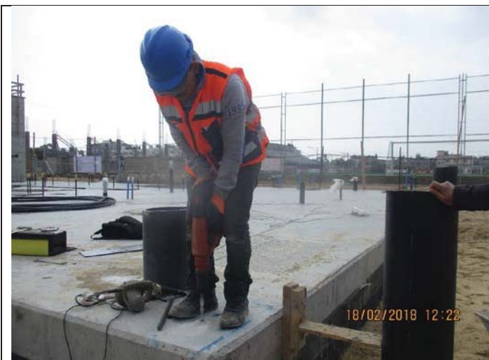
Photo No.25: Start drilling works to install anchor bolts for pretreatment steel structure Date: February 18, 2018
