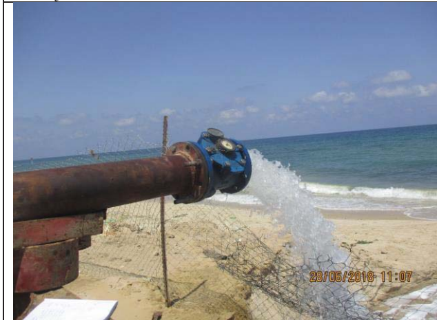
Photo No.33: Pumping test for beach well No. 3. Date: June 28, 2018
