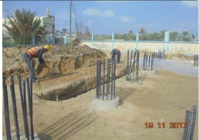
Photo No. 24: R.O building – excavation for electrical trench. Date: November 19, 2017
