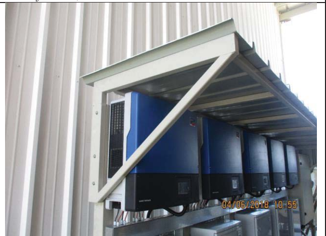
Photo No.06: Shed installation in pretreatment area Date: June 04, 2018
