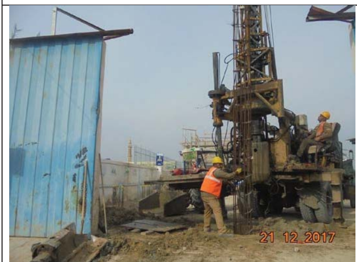
Photo No.45: Excavation works and steel reinforcement for piles Date: December 21, 2017
