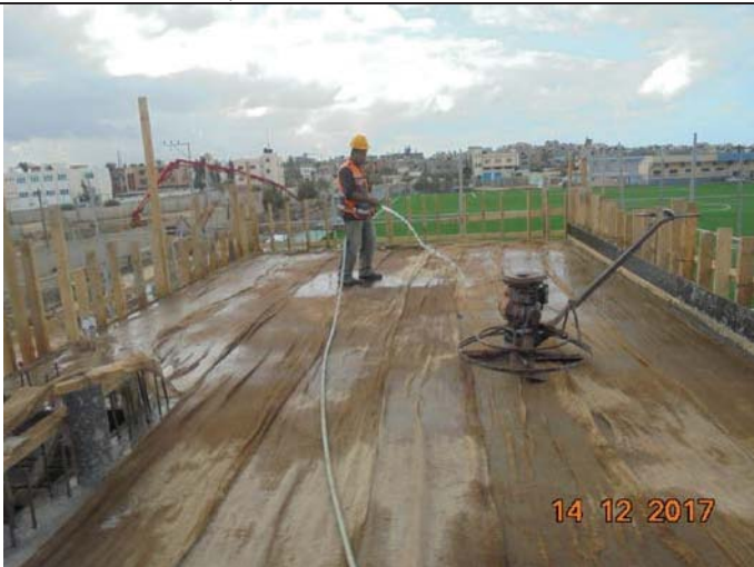
Photo No.31: Raw water and backwash water tanks curing. Date: December 14, 2017
