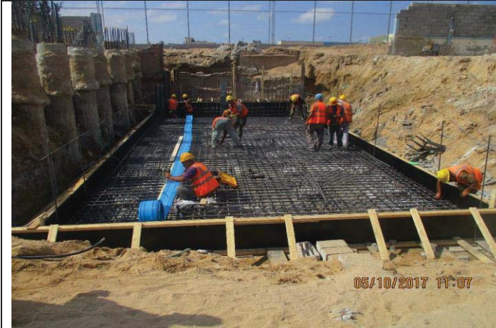
Photo No.07: Brine tank construction activity (reinforcement works) Date: October 5, 2017
