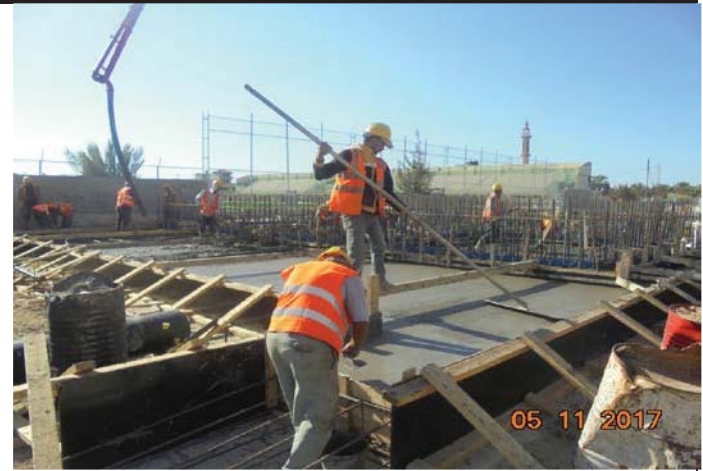
Photo No. 08: Raw water and backwash tanks concrete casting.
