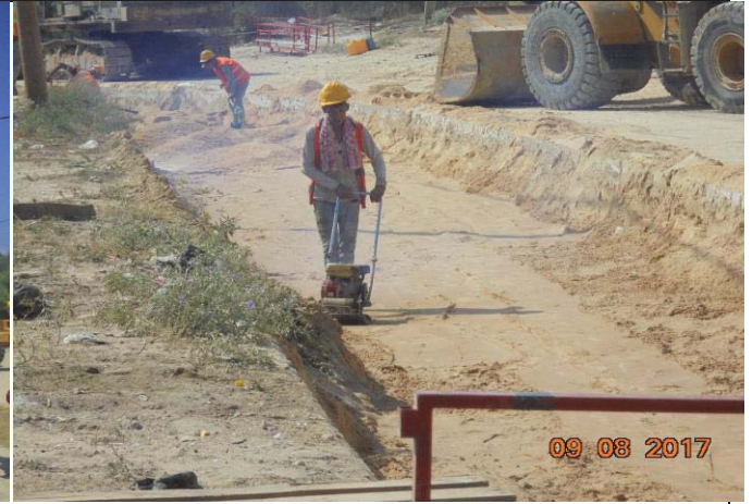
Photo No.26: Pipeline construction activities (compaction backfilling layers). Date: August 09, 2017
