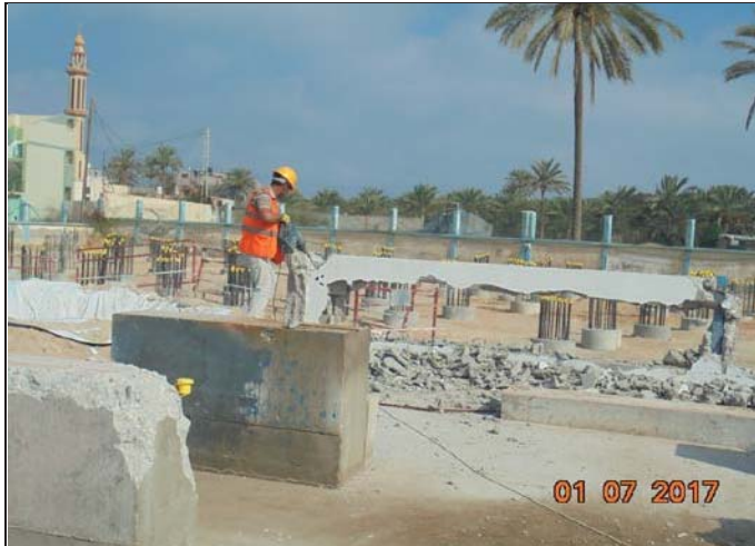
Photo No.01: Continue demolition of existing fuel tank pads. Date: July 01, 2017
