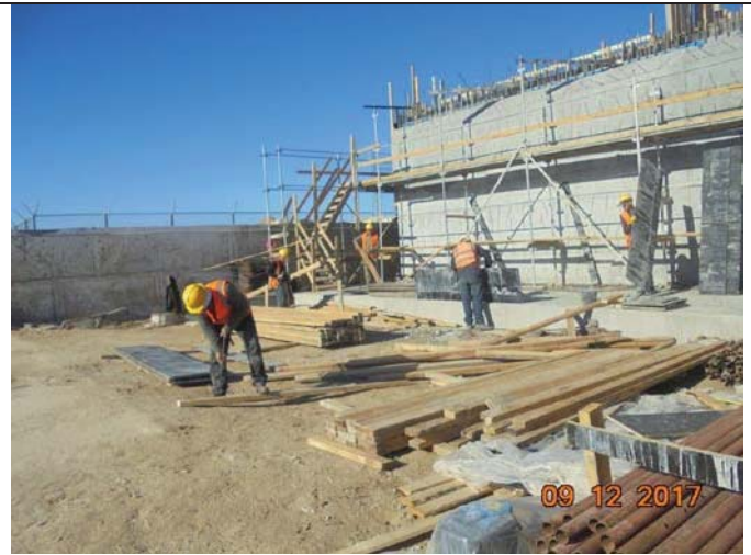
Photo No.16: Curing previously casted walls at raw water and backwash tanks Date: December 07, 2017
