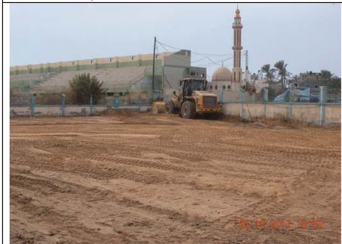
Photo No.15: Site leveling for new proposed RO building. Date: March 18, 2017
