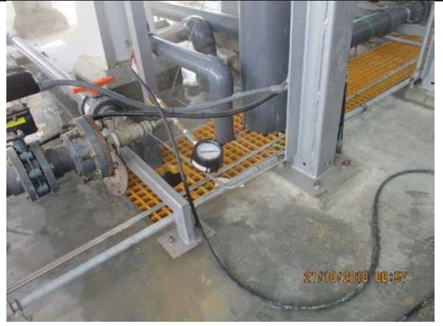
Photo No.12: Hydrostatic testing for DMF tanks Date: October 21, 2018
