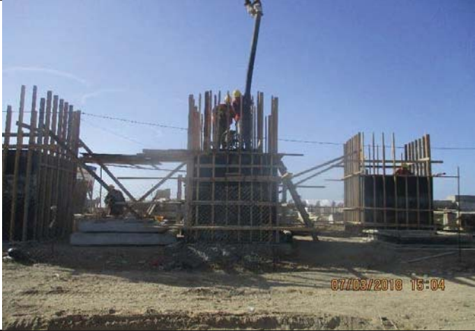
Photo No.07: Casting concrete for mechanical chamber Date: March 07, 2018
