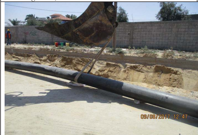
Photo No.27: Pipeline construction activities (pipe laying). Date: August 09, 2017
