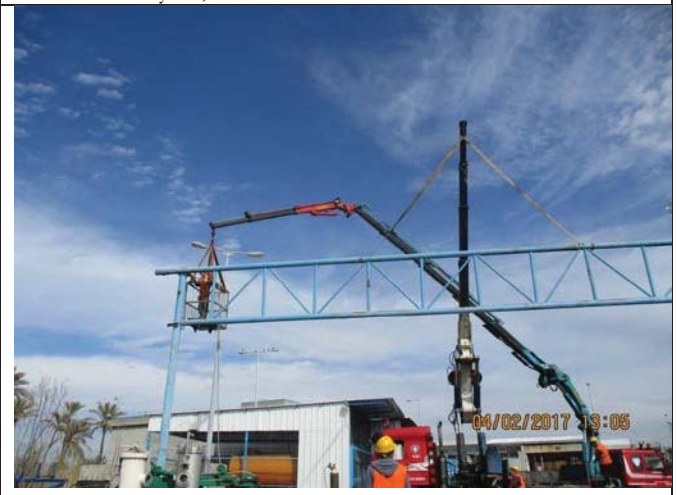
Photo No.04: Continue demolition of existing steel canopy structure Date: February 04, 2017
