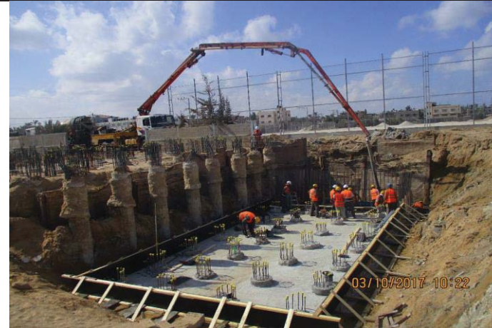
Photo No.05: Brine tank construction activity (concrete casting) Date: October 3, 2017
