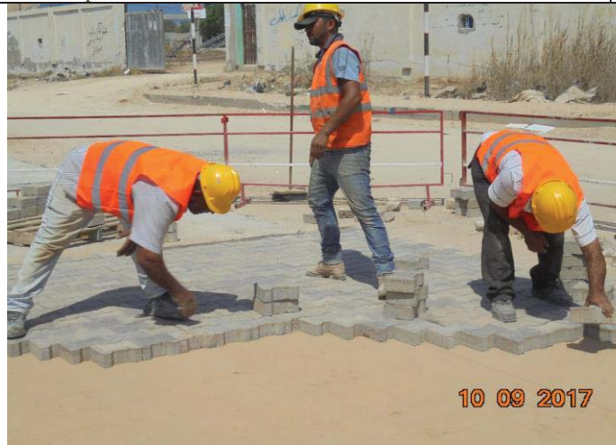
Photo No.15: Surface restoration work ( interlock works ) Date: September 10, 2017
