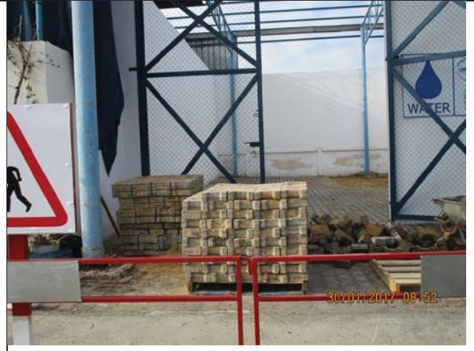
Photo No.12: Removing interlocks. Date: January 30, 2017
