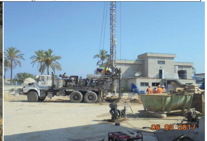
Photo No.18: Pile construction activity (generator pad). Date: August 06, 2017
