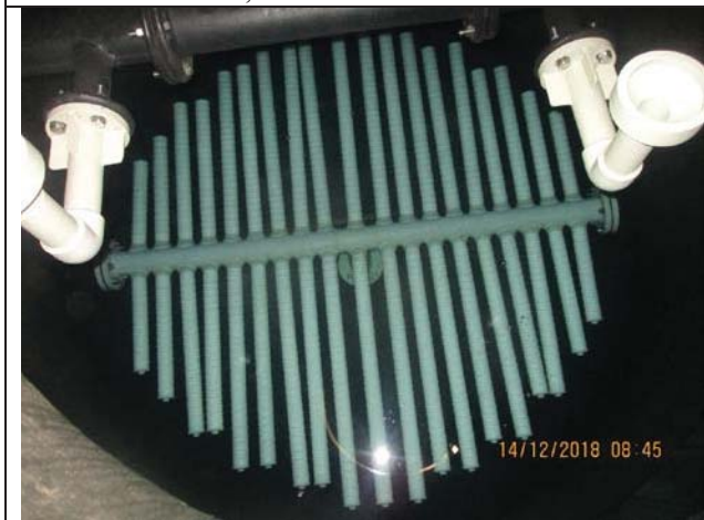
Photo No.15: Filling calcite contactors tanks with water Date: December 14, 2018
