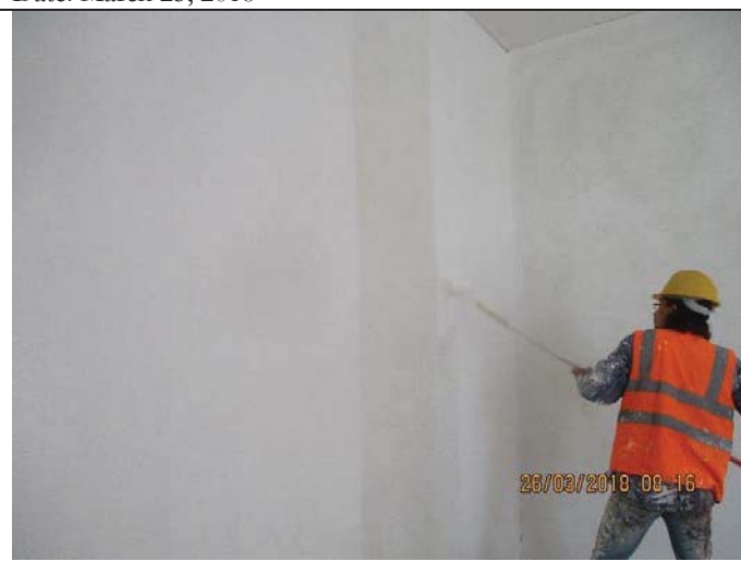
Photo No.26: Painting works for electrical room walls. Date: March 26, 2018
