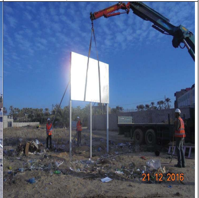
Photo No.16: Temporary sign No.2 installation Date: December 21, 2016
