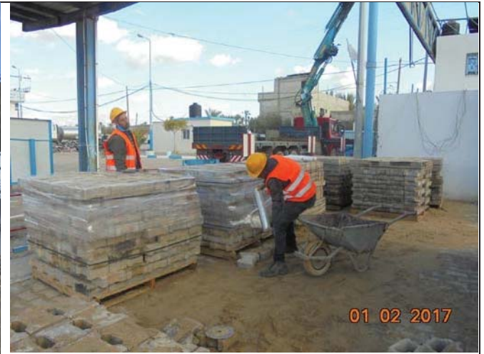
Photo No.02: Continue interlocks demolition. Date: February 01, 2017
