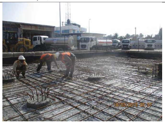
Photo No.24: Continue formwork & steel reinforcement for generator pad Date: February 18, 2018
