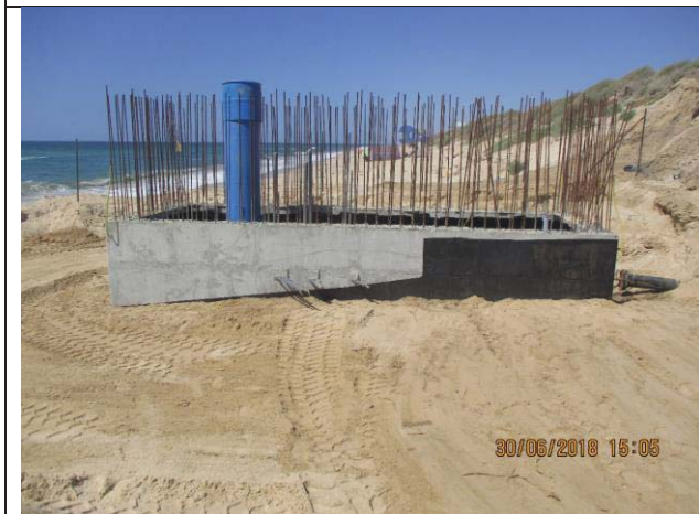
Photo No.35: Backfilling works around beach well No. 1 Date: June 30, 2018
