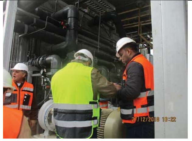
Photo No.26: Functional test for pretreatment Date: December 27, 2018
