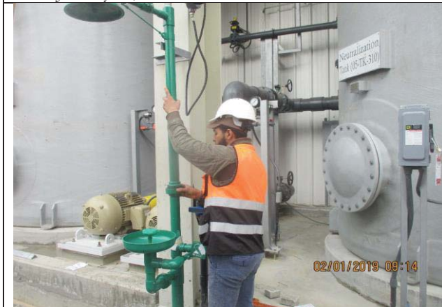
Photo No.03: Functional works for emergency eyewash Date: January 02, 2019
