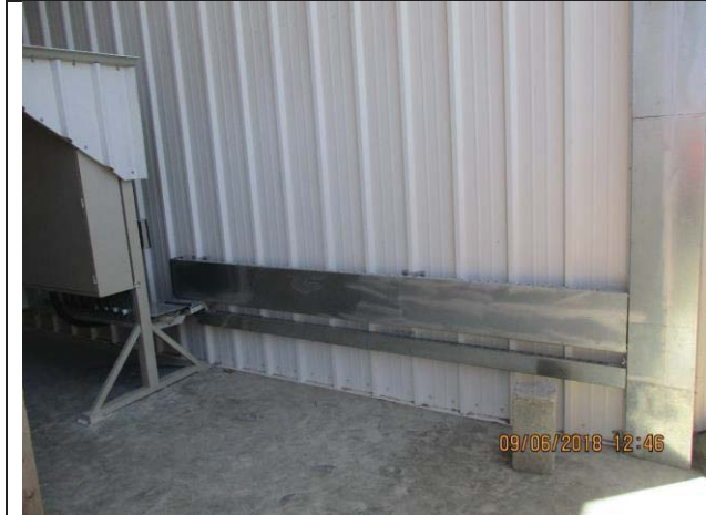
Photo No.13: Installation works for PV system Date: June 09, 2018
