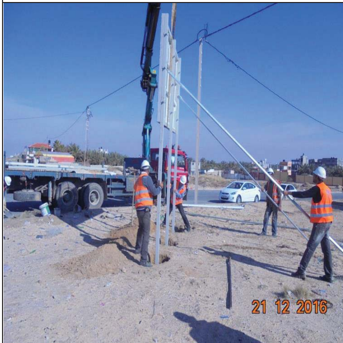
Photo No.15: Temporary sign No.1 installation Date: December 21, 2016
