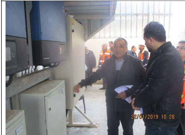
Photo No.15: Initial punch list walkthrough Date: January 22, 2019
