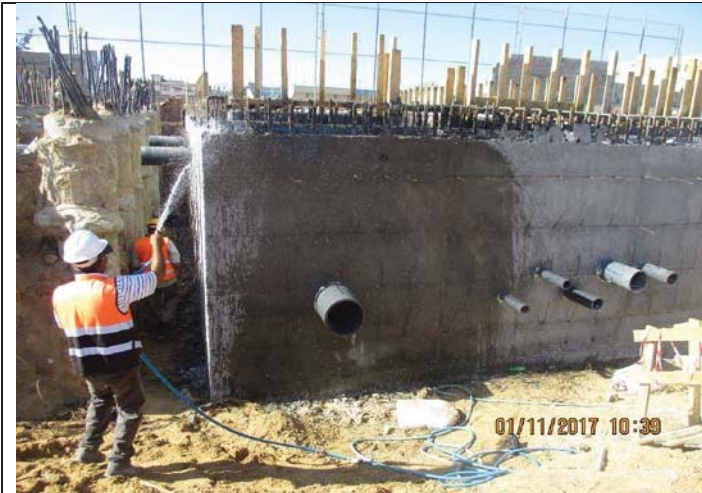
Photo No. 01: Brine tank walls curing
