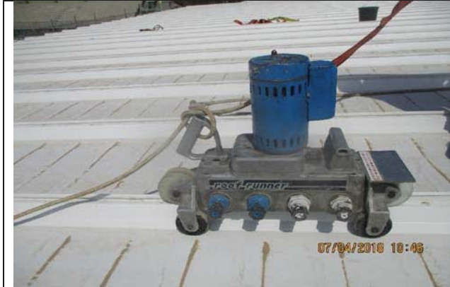
Photo No.13: Closing the joints between roof panels Date: April 07, 2018
