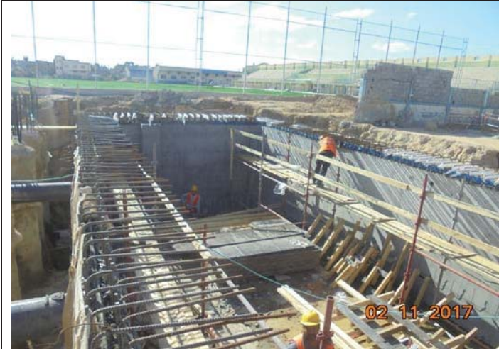
Photo No. 05: Brine tank formwork and tie rod removal.
