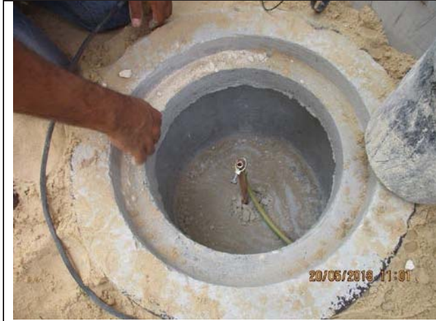
Photo No.19: Grounding manhole installation Date: May 20, 2018
