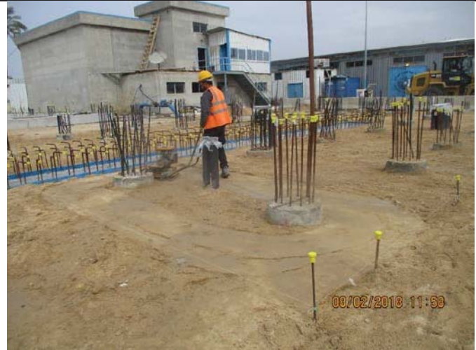
Photo No.14: compaction works for backfilling layers for generator pad
