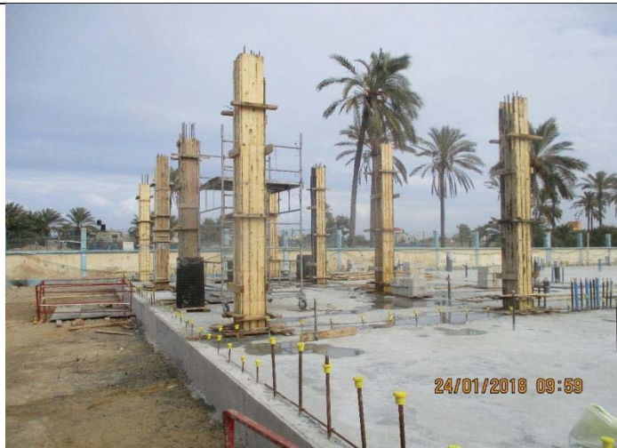
Photo No.33: Curing for casted columns of electrical room. Date: January 24, 2018
