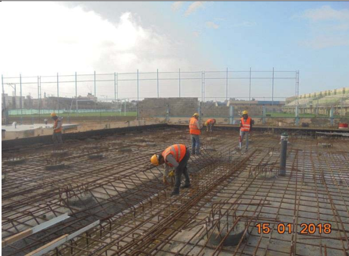
Photo No.15: Steel reinforcement works for RO foundation (phase 2). Date: January 13, 2018
