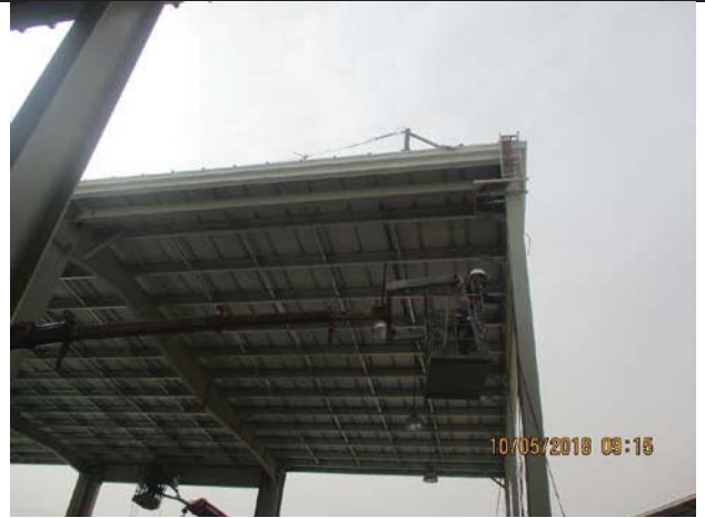
Photo No.12: Start cable tray installation for generator canopy Date: May 10, 2018
