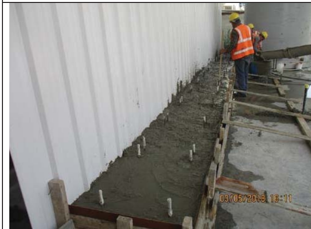
Photo No.05: Casting concrete for chemical skid area pad. Date: May 03, 2018
