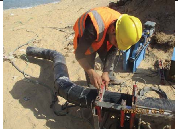
Photo No.20: Connection works for beach wells pipes Date: September 16, 2018
