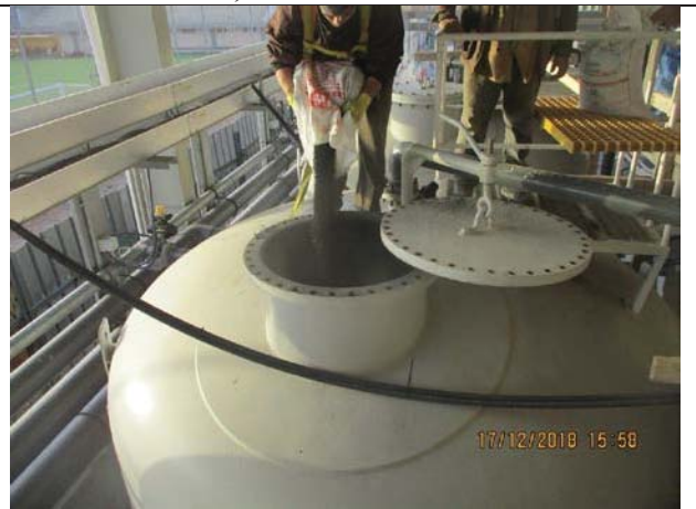
Photo No.18: Filling Anthracite inside DMF tanks Date: December 17, 2018
