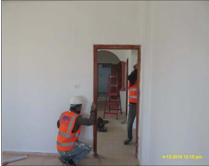
Photo No.05: Primary field office painting works Date: December 04, 2016
