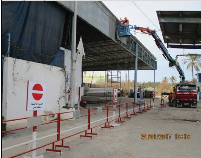
Photo No.03: Demolition of existing canopy steel structure Date: January 24, 2017
