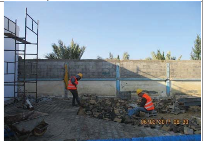
Photo No.08: Continue interlocks demolition
