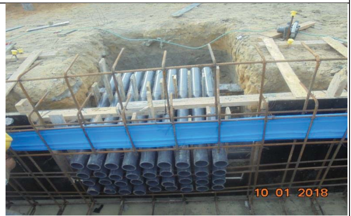
Photo No.10: Electrical conduits installation for electrical room trench. Date: January 10, 2018
