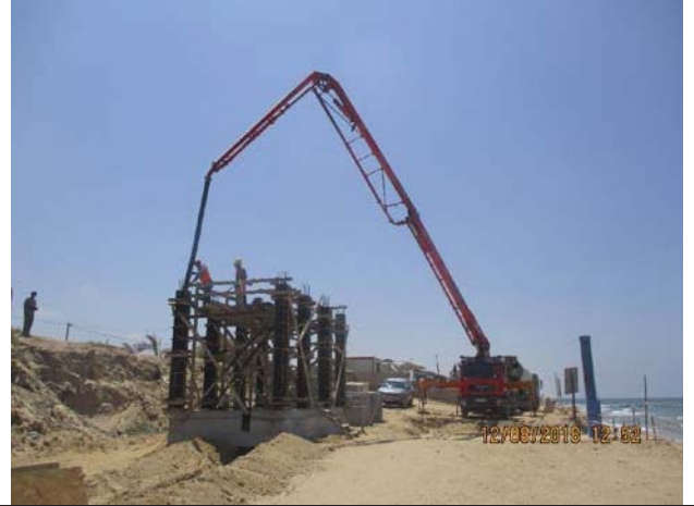
Photo No.16: Casting concrete for electrical room columns Date: August 12, 2018
