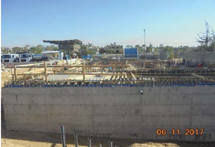
Photo No. 11: Brine tank formwork removal and slab formwork preparation works
