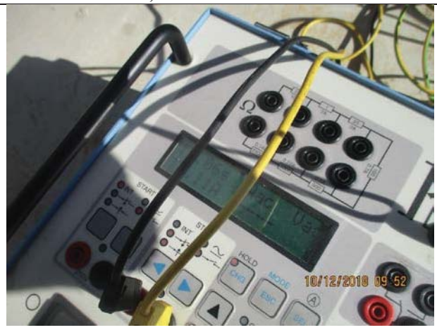
Photo No.12: Schneider representative working on current injection test Date: December 10, 2018
