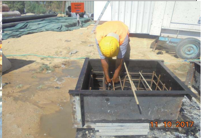
Photo No.18: Concrete encasement (collar) for outfall pipeline. Date: October 11, 2017
