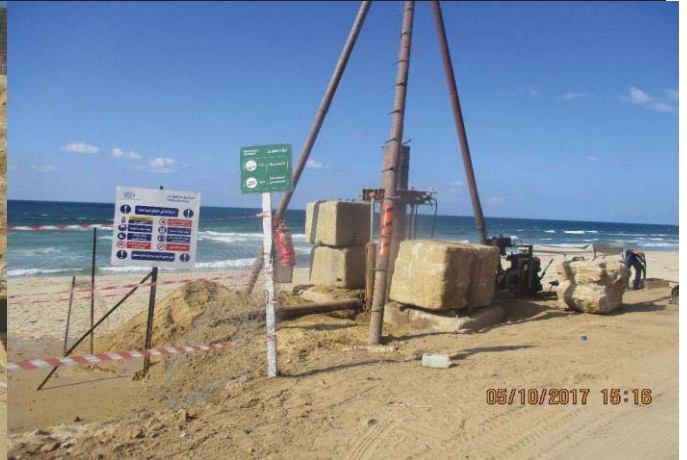
Photo No.08: Beach well drilling activity (beach well No. 02) Date: October 5, 2017
