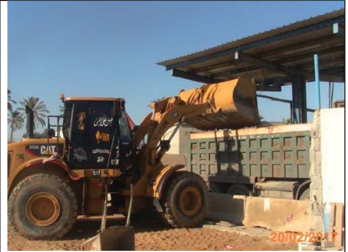
Photo No.18: Transferring debris to dumping site Date: February 20, 2017
