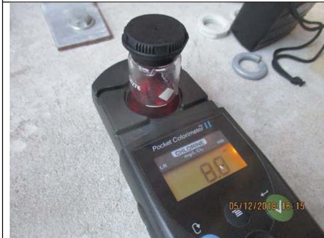
Photo No.09: Disinfection and flushing works for all pipes. Date: December 05, 2018
