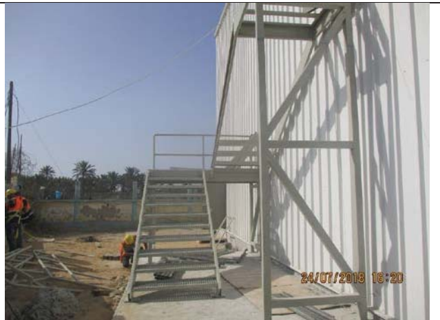
Photo No.30: Staircase installation for RO building Date: July 24, 2018
