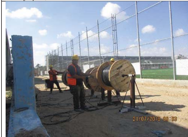
Photo No.23: Extending cables for Pretreatment Area Date: July 21, 2018
