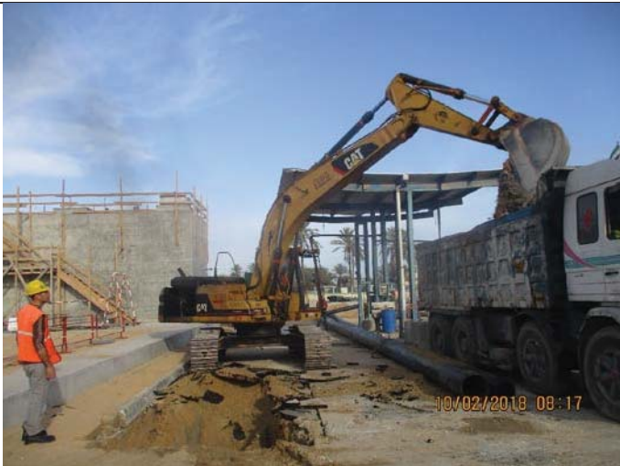
Photo No.15: start excavation works to install pipes inside construction site
