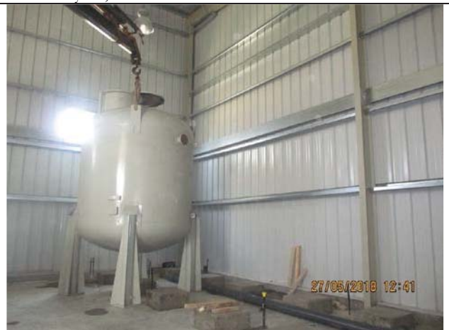
Photo No.24: Installation works for calcite contactors (3 units) Date: May 27, 2018
