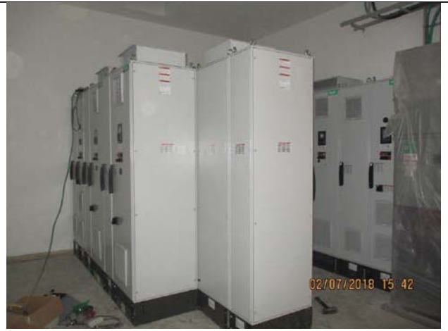
Photo No.02: Installation of VFD panels (6 panels) Date: July 02 2018
