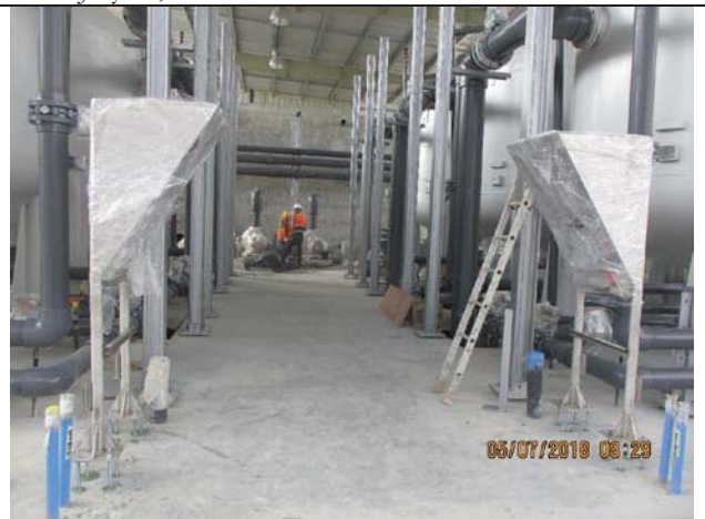
Photo No.06: Local control panel installation Date: July 05, 2018
