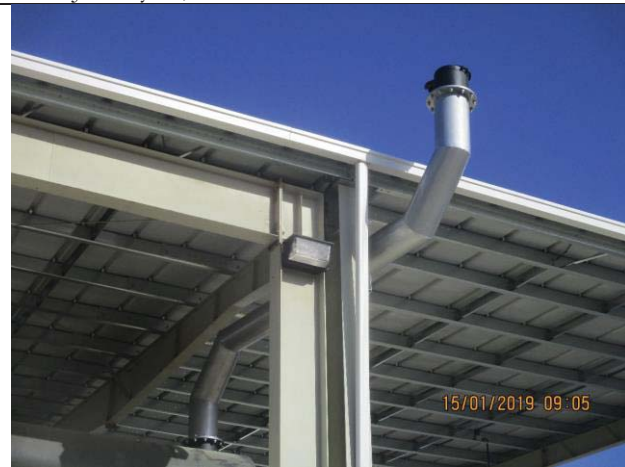
Photo No.09: Closing punch list items "painting generator exhaust" Date: January 15, 2019
