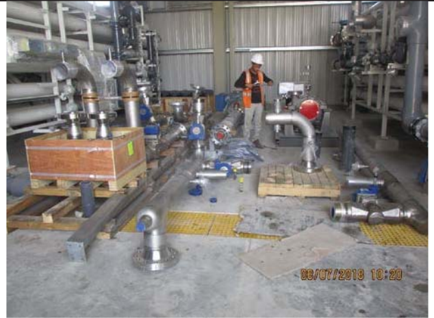
Photo No.10: Continue assembly of 1 st pass RO skid Date: July 08, 2018
