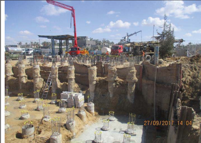
Photo No.37: Brine tank construction activity (mat foundation preparation works) Date: September 27, 2017
