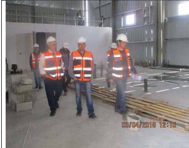
Photo No.07: USAID visit Date: April 03, 2018
