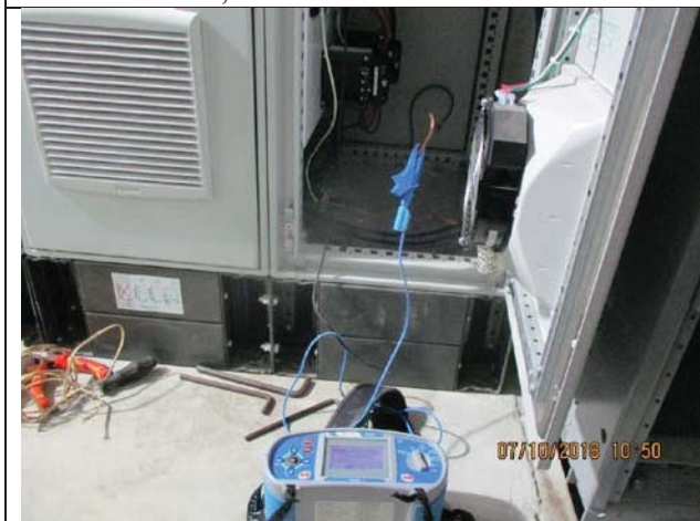
Photo No.05: Megger testing Date: October 07, 2018
