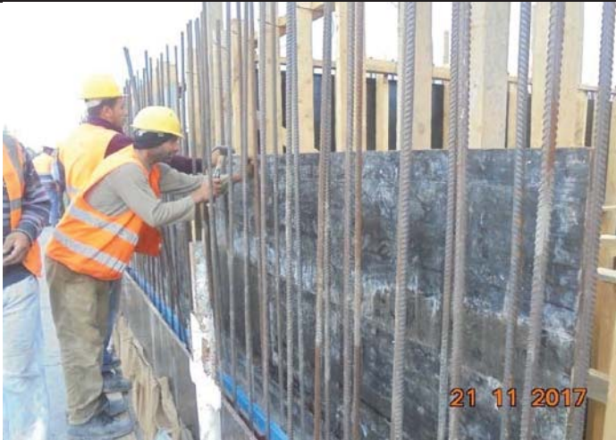
Photo No. 25: Raw water and backwash tank formwork Date: November 21, 2017
