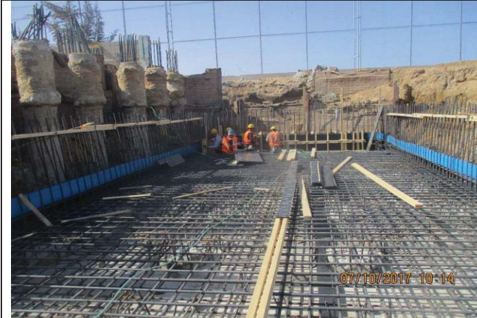
Photo No.09: Brine tank construction activity (reinforcement works) Date: October 7, 2017
