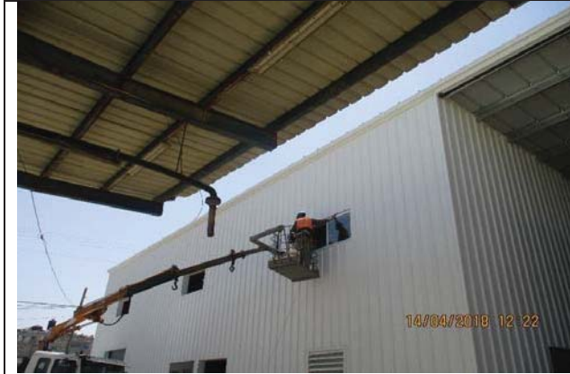
Photo No.19: Accessories installation for steel structures (doors, louvers...etc.) Date: April 14, 2018
