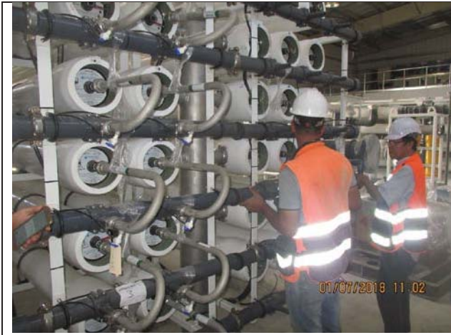
Photo No.01: Start assembly of 1 st pass RO skid Date: July 01, 2018
