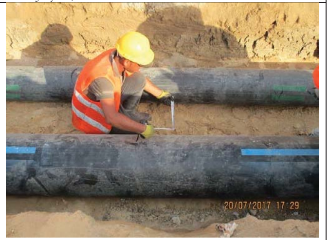
Photo No.30: Pipeline (outfall and intake) laying and fixation. Date: July 20, 2017
