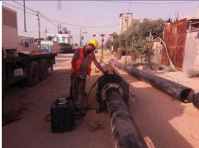
Photo No.17: HDPE pipes welding activity. Date: July 13, 2017
