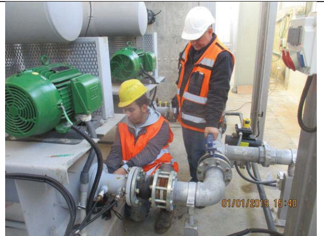
Photo No.02: Functional works for blowers inside Pretreatment Building Date: January 01, 2019
