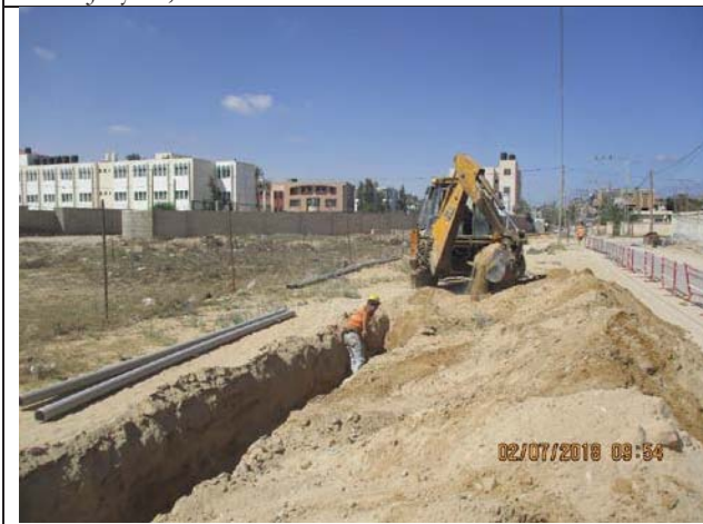
Photo No.03: Installing the MV cables (final phase) Date: July 02, 2018
