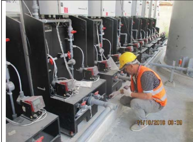
Photo No.07: Mechanical works for chemical skids Date: October 11, 2018
