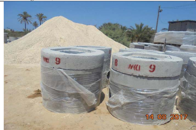
Photo No.35: Pipeline construction activity (electrical manholes) Date: August 15, 2017
