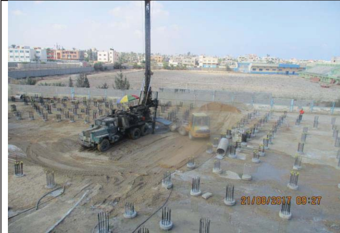
Photo 49: Pile construction activity (pile drilling). Date: August 21, 2017
