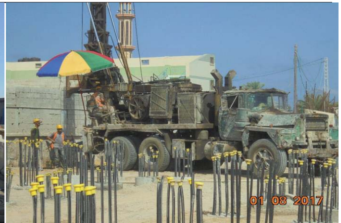
Photo No.02: Pile construction activity (brine tank). Date: August 01, 2017
