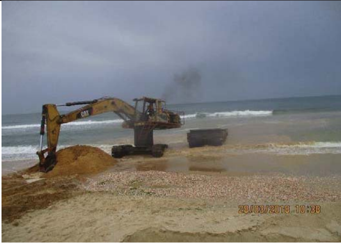
Photo No.31: Preparation works for outfall pipeline installation Date: March 28, 2018
