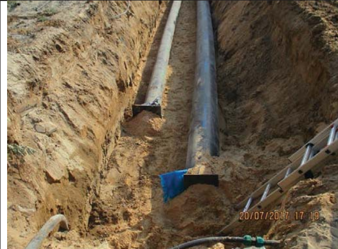
Photo No.31: Pipeline (outfall and intake) end protection. Date: July 20, 2017
