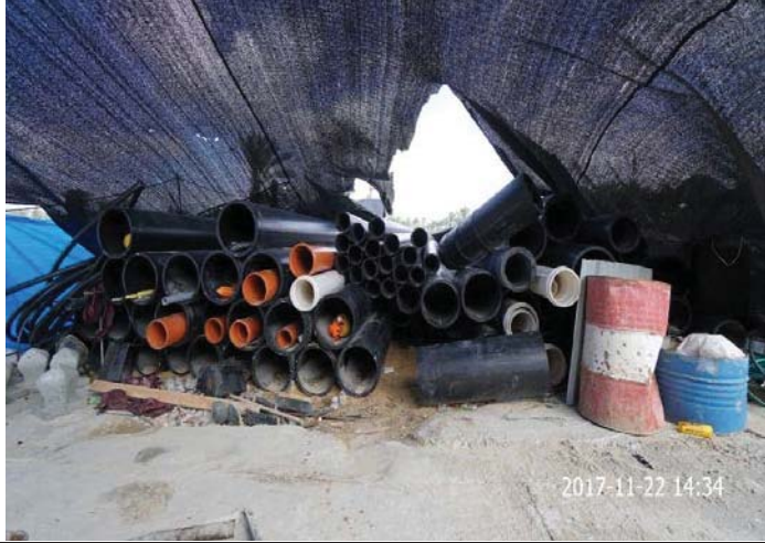
Photo No. 35: HDPE pipes stored at storage yard Date: November 22, 2017
