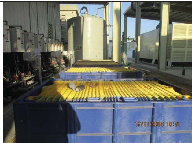
Photo No.09: IBC containments tanks installation Date: November 17, 2018
