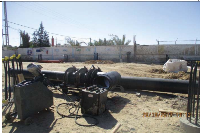
Photo No.53: HDPE pipes welding works prior to intake and outfall pipeline. Date: October 26, 2017
