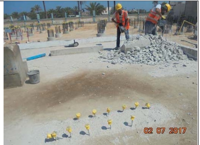
Photo No.02: Continue demolition of existing fuel tank pads. Date: July 02, 2017
