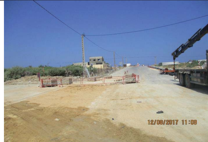
Photo No.31: Pipeline construction activity (interlock dismantling activity). Date: August 12, 2017
