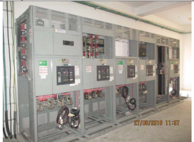
Photo No.28: VFD panels installation inside electrical room Date: June 27, 2018
