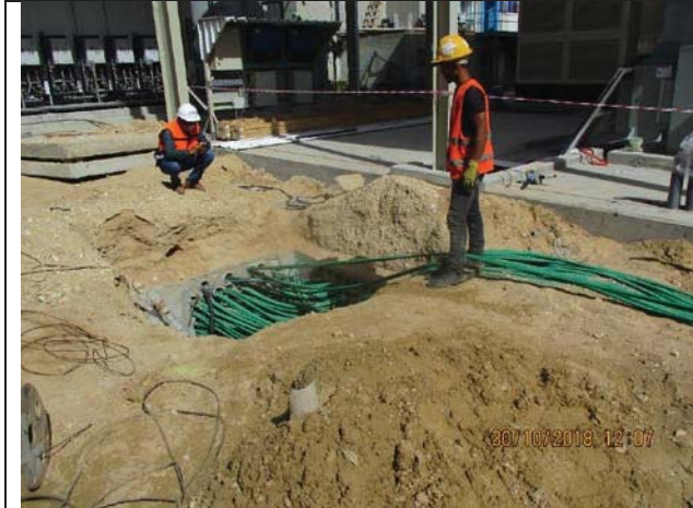
Photo No.19: Extending cables in construction site Date: October 30, 2018
