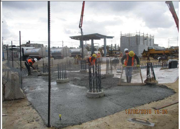
Photo No.20: Casting concrete for generator pad blinding Date: February 13, 2018
