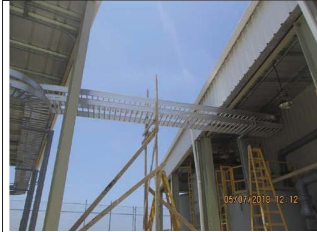
Photo No.07: Cable ladder installation in pretreatment area Date: July 05, 2018
