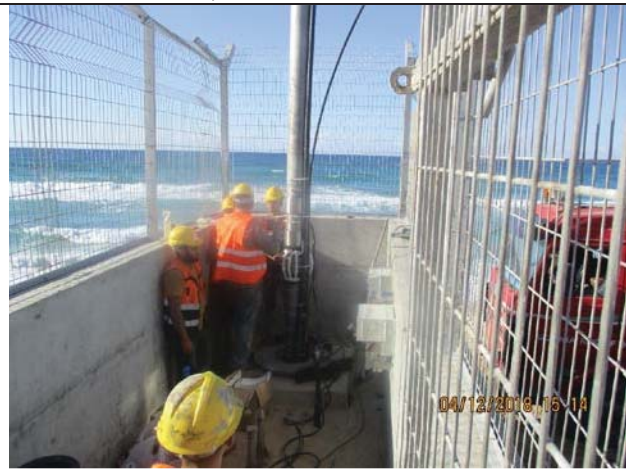
Photo No.05: Installation works for beach well No. 1 pump Date: December 04, 2018
