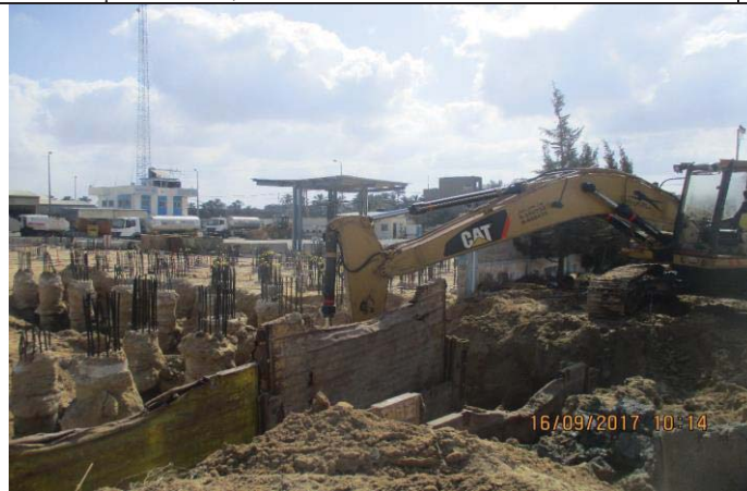
Photo No.29: Structural excavation (brine tank excavation side protection) Date: September 16, 2017
