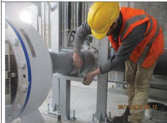
Photo No.17: Finishing pipes support works Date: November 30, 2018
