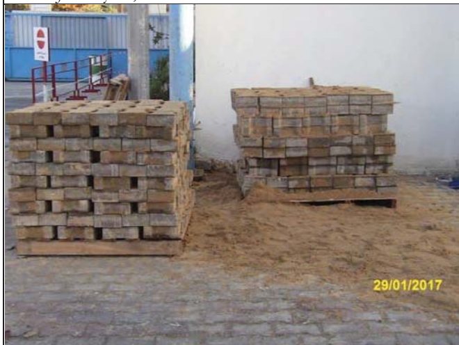
Photo No.09: Removing interlocks. Date: January 29, 2017
