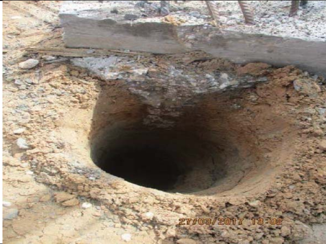
Photo No.29: Drilling investigation boreholes near R06 & R08 piles. Date: March 27, 2017
