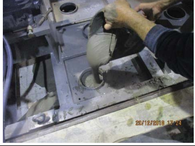
Photo No.20: Grouting works for pumps inside RO Building. Date: December 20, 2018
