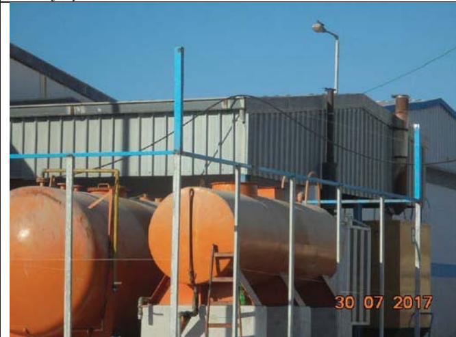
Photo No.39: Continue works at fuel tank area Date: July 30, 2017
