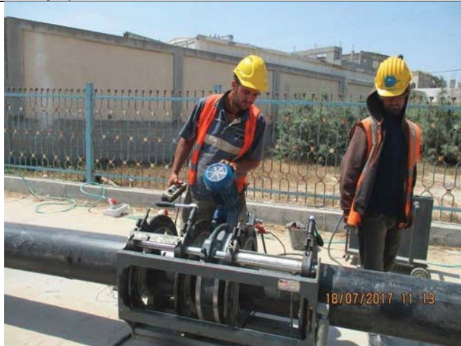
Photo No.23: HDPE pipes welding activity. Date: July 18, 2017
