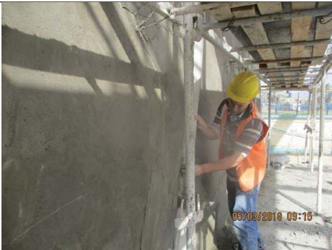
Photo No.03: Continue plastering works for electrical room
