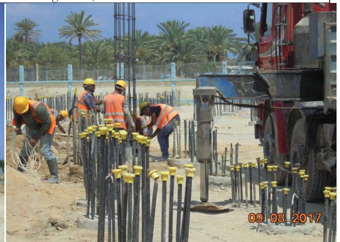
Photo No.30: Pile construction activities. Date: August 09, 2017
