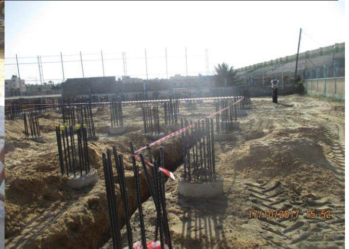
Photo No.32: Continue steel fabrication for outfall pipeline weight collars. Date: October 17, 2017
