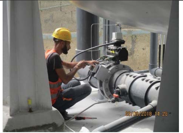
Photo No.32: Connection works for instruments Date: September 29, 2018
