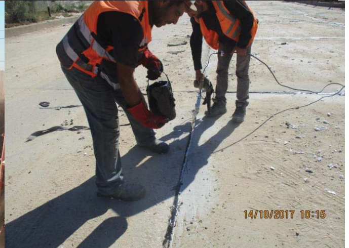
Photo No.26: Continue joints filling between concrete panels. Date: October 14, 2017
