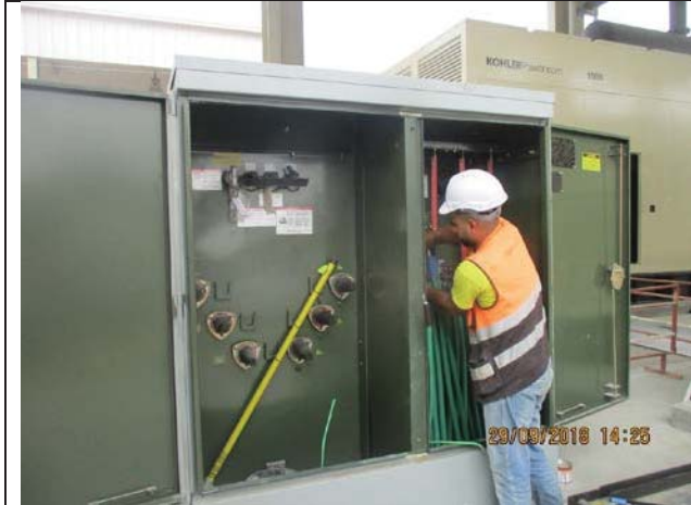
Photo No.31: Electrical works in generator canopy Date: September 29, 2018
