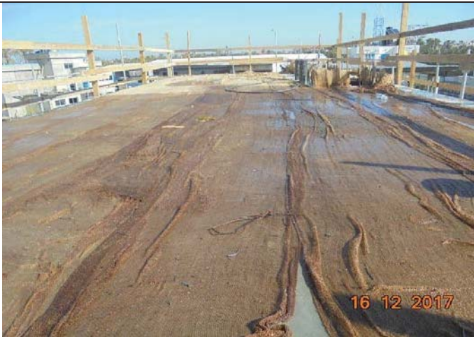
Photo No.33: Raw water and backwash tanks slab curing Date: December 16, 2017
