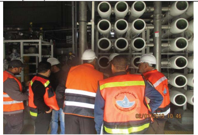
Photo No.04: Onsite training for PWA staff "ERI System" Date: January 02, 2019
