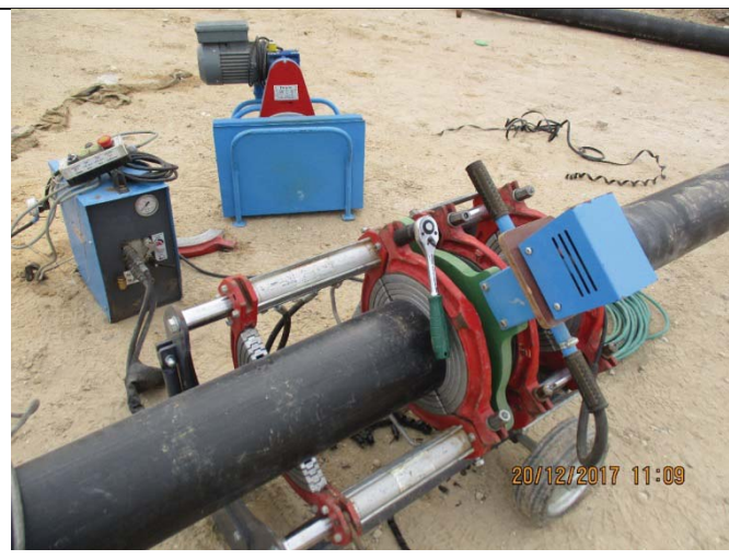
Photo No.42: HDPE intake pipeline welding work Date: December 20, 2017
