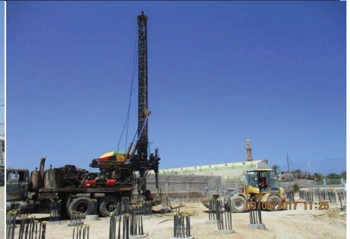
Photo No. 14: Pile construction activity (brine tank). Date: August 03, 2017
