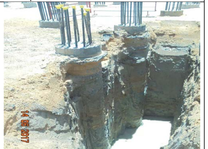
Photo No.08.2: Piles integrity test at RO building. Date: June 14, 2017
