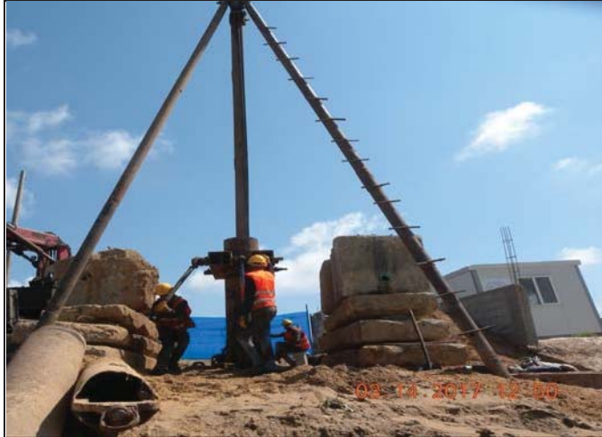
Photo No.11: Hydrogeology investigation by drilling one beach well borehole. Date: March 14, 2017
