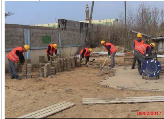
Photo No.13: Continue interlocks demolition Date: February 09, 2017
