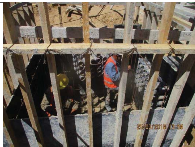
Photo No.24: Shuttering works for electrical manhole Date: March 25, 2018
