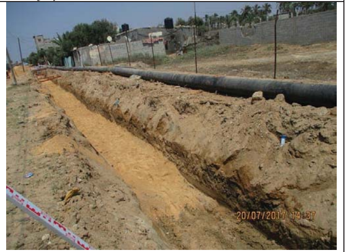
Photo No.28: Pipeline bedding using clean sand. Date: July 20, 2017
