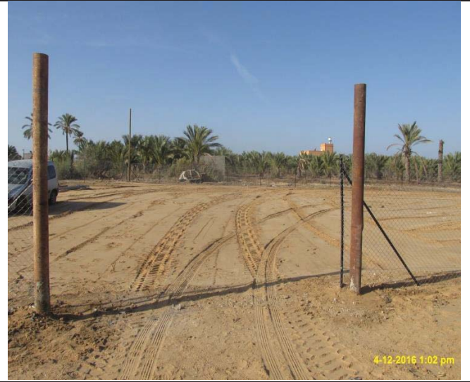
Photo No.06: Storage yard fence erection Date: December 04, 2016
