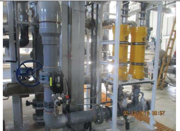
Photo No.02: Assembly works for RO system Date: December 02, 2018
