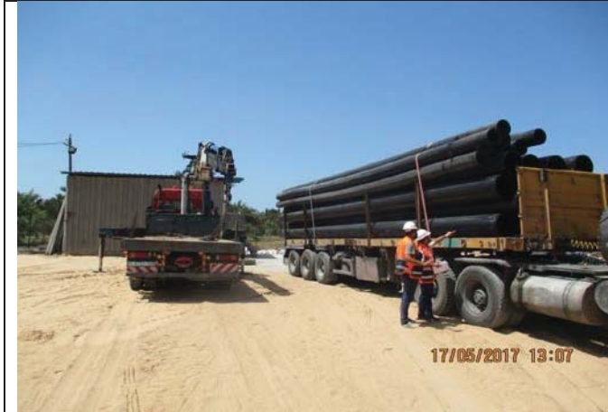
Photo No.07: Delivery and storage of Plassim HDPE pipes at storage yard. Date: May 17, 2017
