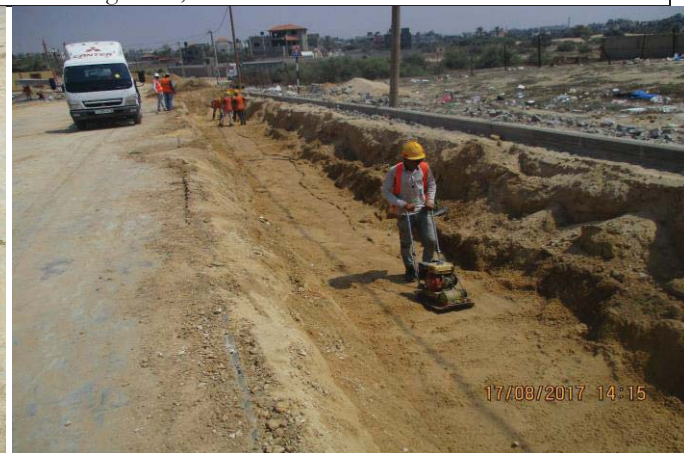
Photo No.42: Pipeline construction activity (compacting layers). Date: August 17, 2017
