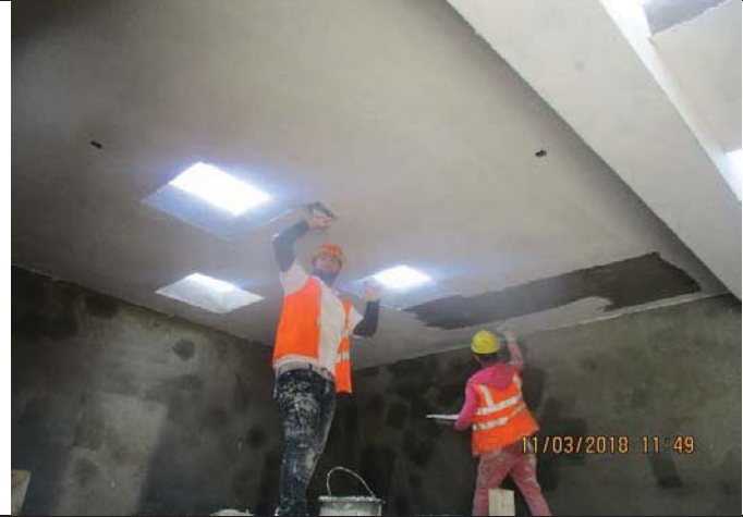
Photo No.08: Continue plastering works for electrical room Date: March 11, 2018
