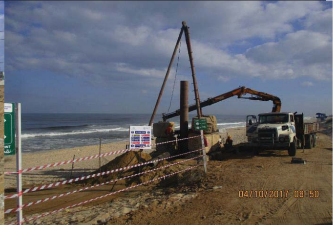
Photo No.06: Beach well construction activity (drilling works) Date: October 4, 2017
