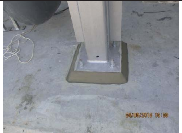
Photo No.04: Grouting works for steel support Date: August 04, 2018
