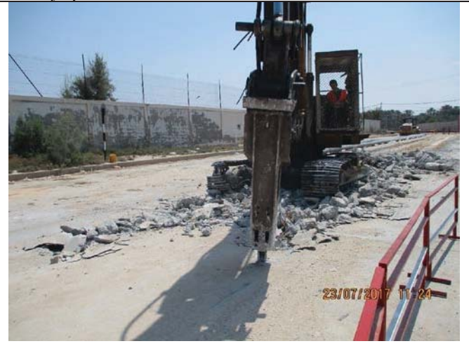
Photo No.34: Pipeline preparation activities-Demolishing concrete road. Date: July 23, 2017
