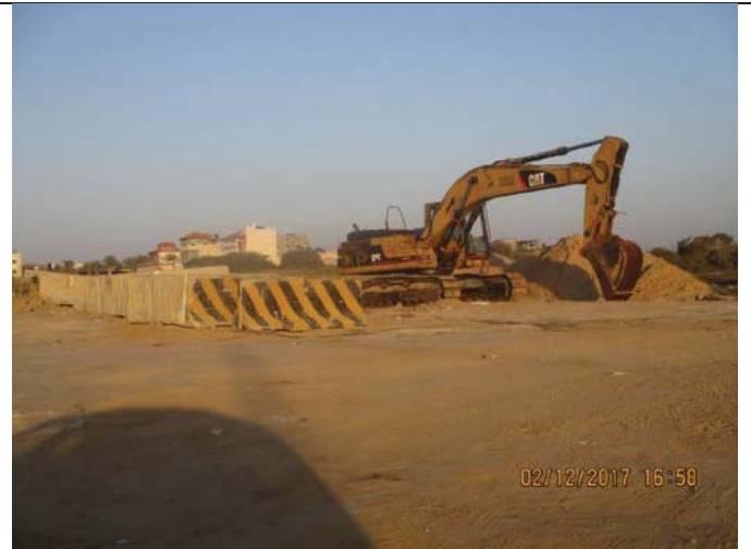
Photo No.02: Idle Equipment.
