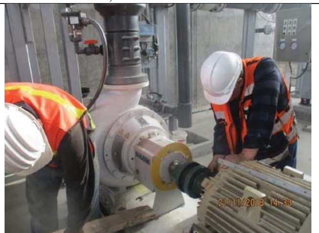
Photo No.12: Alignment for shaft coupling for pretreatment pumps Date: November 21, 2018
