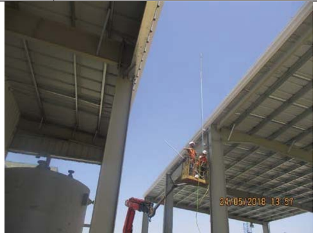
Photo No.22: Lightening protection system installation Date: May 24, 2018
