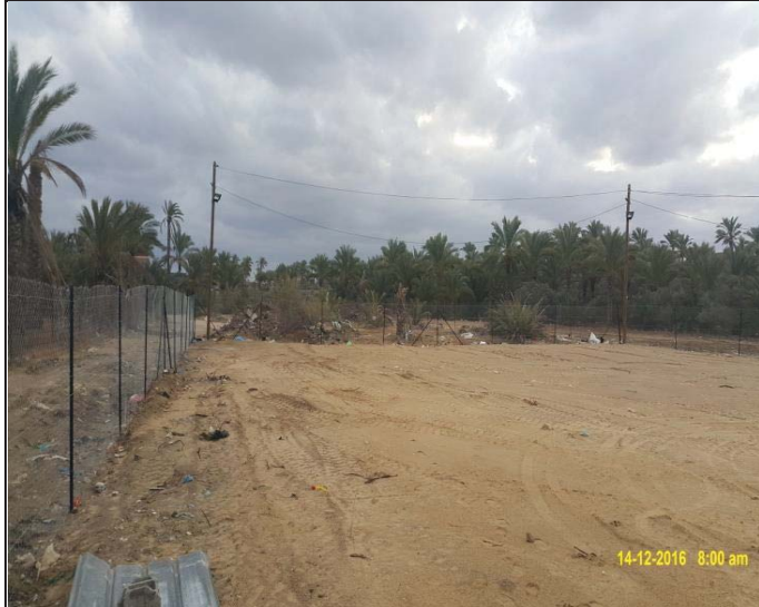
Photo No.09: Storage yard fencing and civil works
