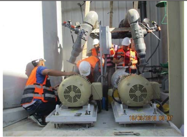
Photo No.22: Leveling works and alignment for CIP pumps. Date: September 18, 2018
