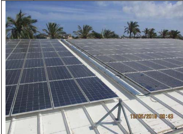
Photo No.15: Cable tray installation for RO canopy Date: May 13, 2018
