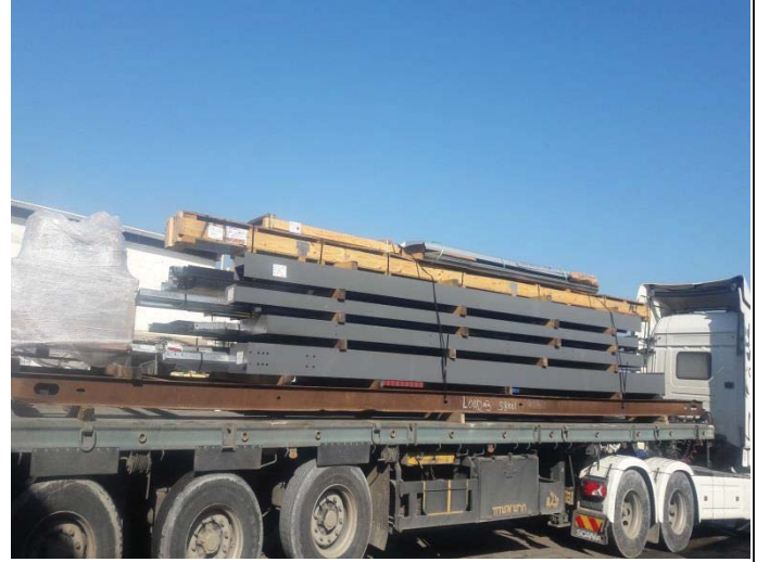
Photo No.46: Delivery of pre-engineered steel structures. Date: January 30, 2018
