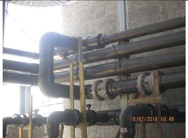
Photo No.20: Installation of PVC manifolds Date: July 18, 2018
