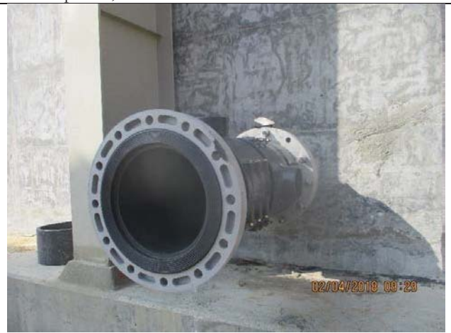
Photo No.04: fittings installation for raw water tank. Date: April 02, 2018
