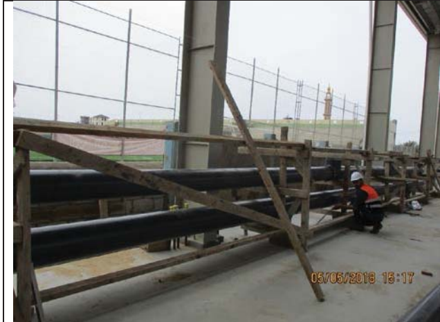
Photo No.07: Fabrication and installation works for PVC manifold Date: May 05, 2018
