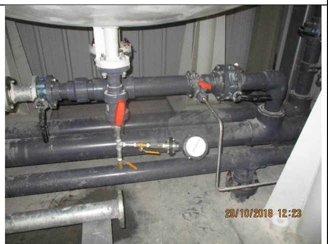
Photo No.16.2: Hydrostatic test for calcite contactors Date: October 29, 2018
