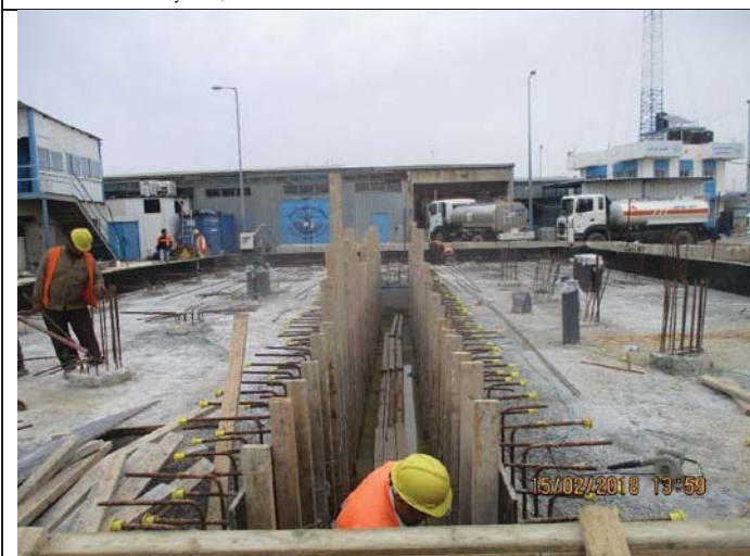
Photo No.23: Formwork for generator pad Date: February 15, 2018
