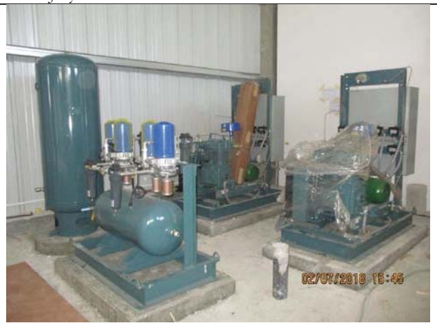
Photo No.04: Air compressor installation Date: July 02, 2018
