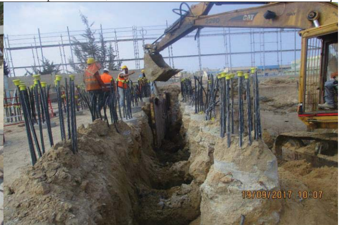
Photo No.24: Structural excavation (brine tank excavation). Date: September 19, 2017
