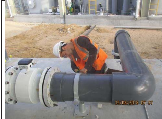
Photo No.19: Connection works for brine tank Date: August 15, 2018
