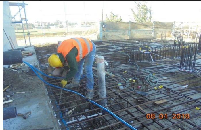
Photo No.07: De-shuttering works for RO foundation. Date: January 08, 2018
