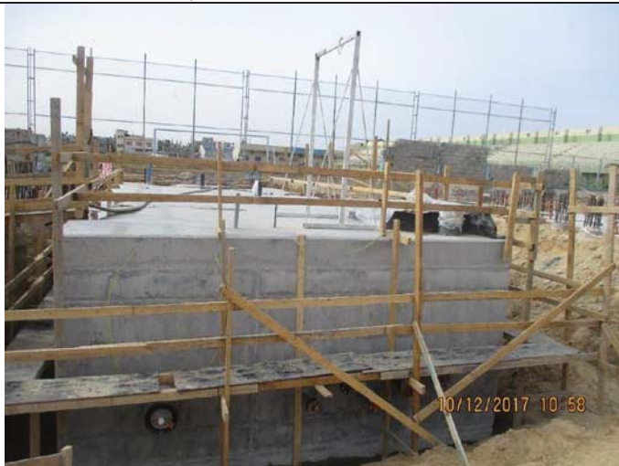
Photo No.21: Brine tank water filling progress Date: December 10, 2017
