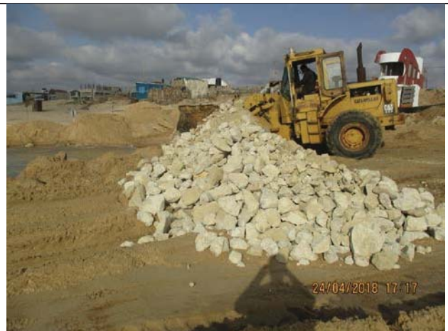
Photo No.36: start rock gravel backfilling above outfall pipeline Date: April 24, 2018
