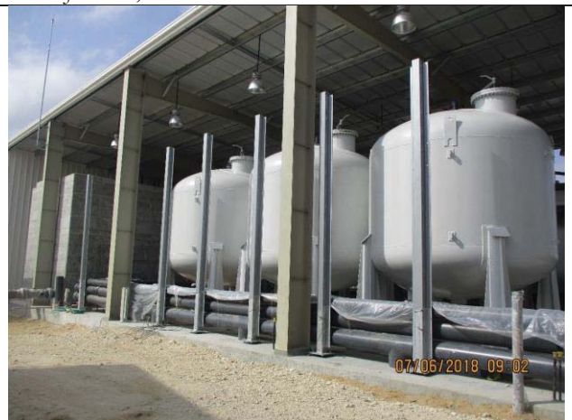
Photo No.12: Steel support installation Date: June 07, 2018
