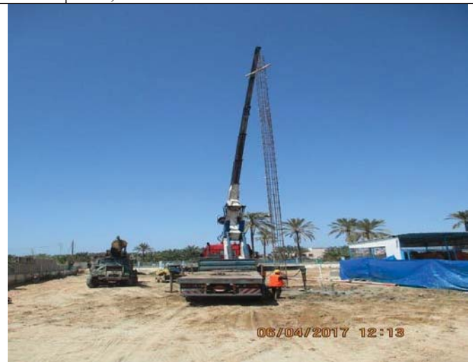
Photo No.09: Installation of reinforcement steel case. Date: April 06, 2017
