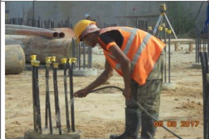
Photo No.23: Pile construction activity (curing previously casted piles). Date: August 08, 2017
