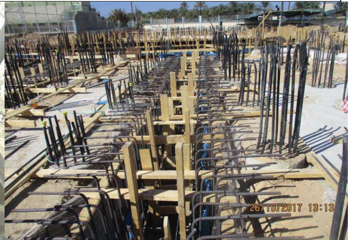
Photo No.52: Pre-treatment building trench formwork and steel reinforcing. Date: October 26, 2017
