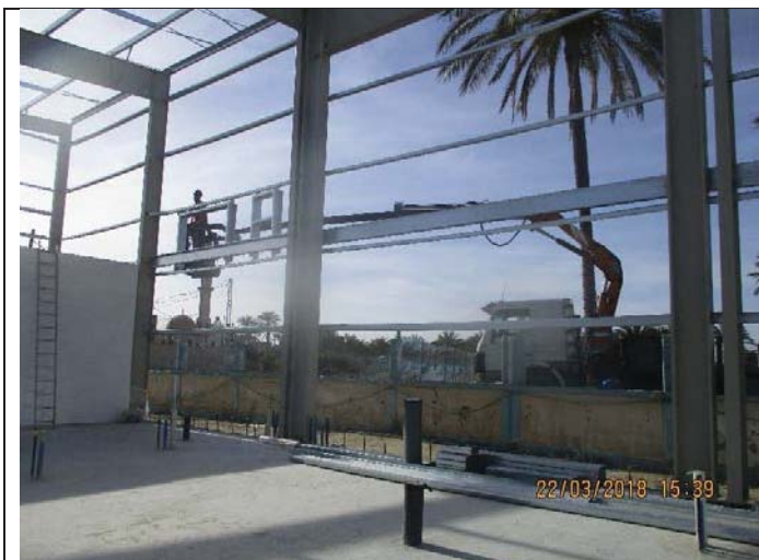
Photo No.23: Start works in walls of RO building. Date: March 22, 2018
