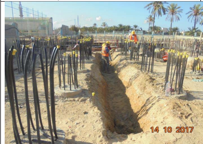
Photo No.23: Trench excavation in pretreatment building. Date: October 14, 2017
