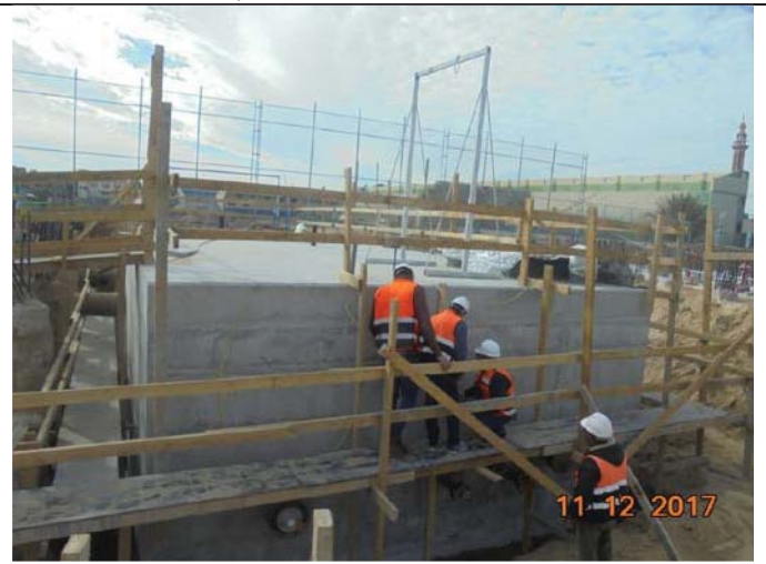
Photo No.24: Brine tank water filling completion. Date: December 11, 2017
