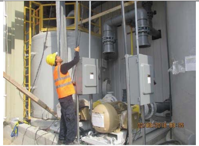
Photo No.02: Extending cables for pumps in RO Building. Date: August 02, 2018
