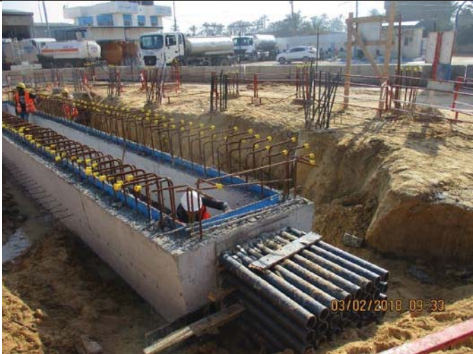
Photo No.03: De-shuttering works for generator pad trench
