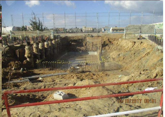
Photo No.14: Cleaning brine tank. Date: October 10, 2017
