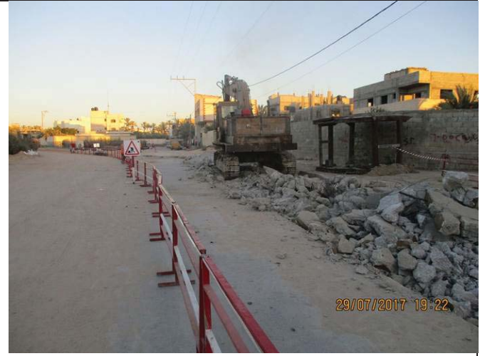
Photo No.38: Pipeline preparation activities-Demolishing concrete road. Date: July 29, 2017
