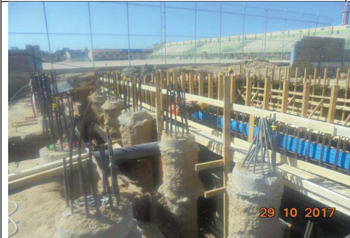
Photo No.57: Continue brine tank construction activities - thimbles installation. Date: October 29, 2017
