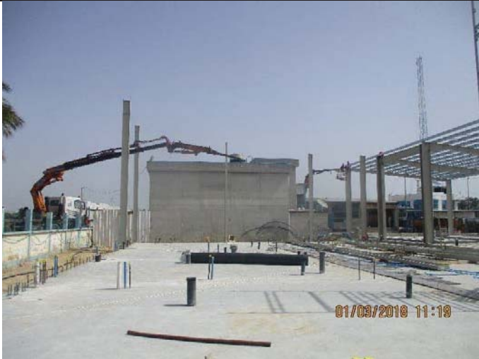
Photo No.01: Erection works for RO steel structure
