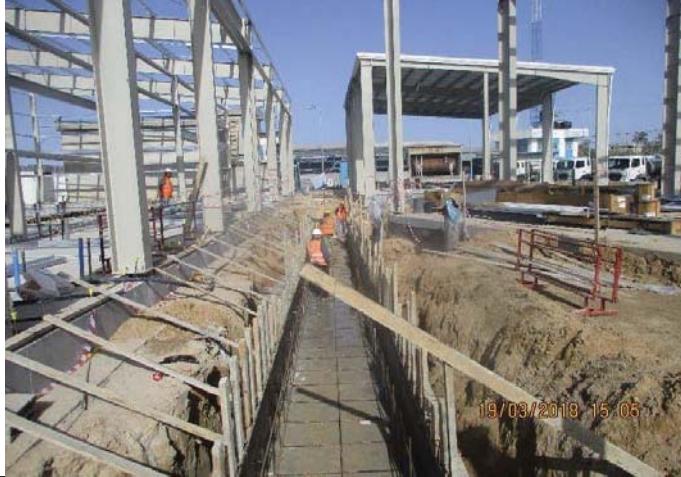
Photo No.19: Shuttering works for duct bank. Date: March 19, 2018
