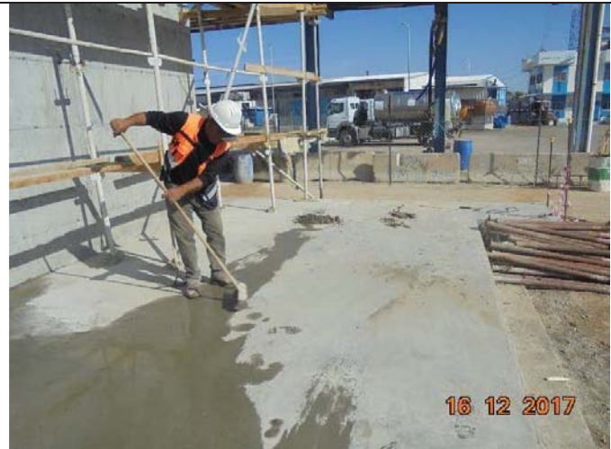
Photo No.34: Housekeeping works for construction site Date: December 16, 2017
