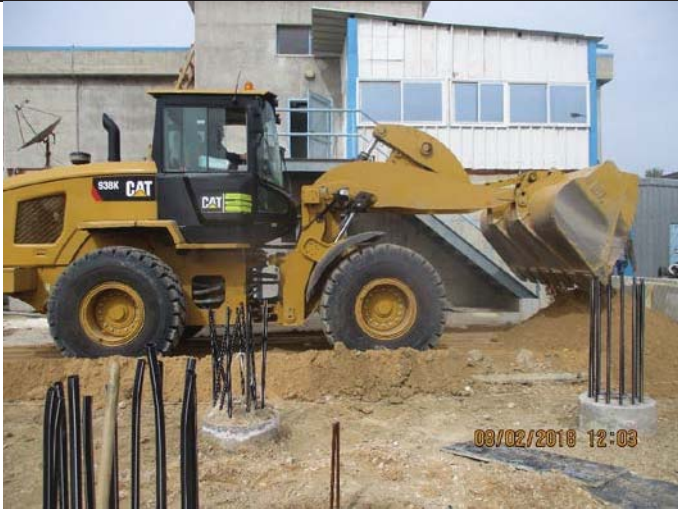
Photo No.13: Leveling works for generator pad
