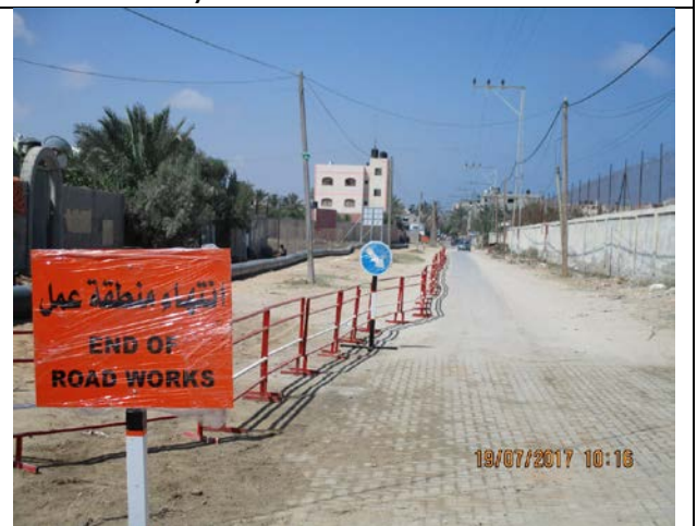
Photo No. 06.I: Housekeeping & safety arrangements during construction works. Date: July 19, 2017
