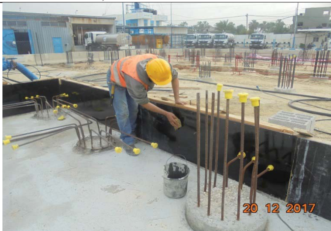
Photo No.40: Start formwork for RO building foundation Date: December 20, 2017
