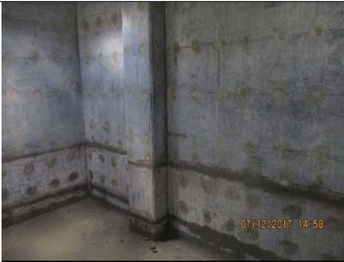
Photo No.17: Brine tank internal walls repair works completion Date: December 07, 2017
