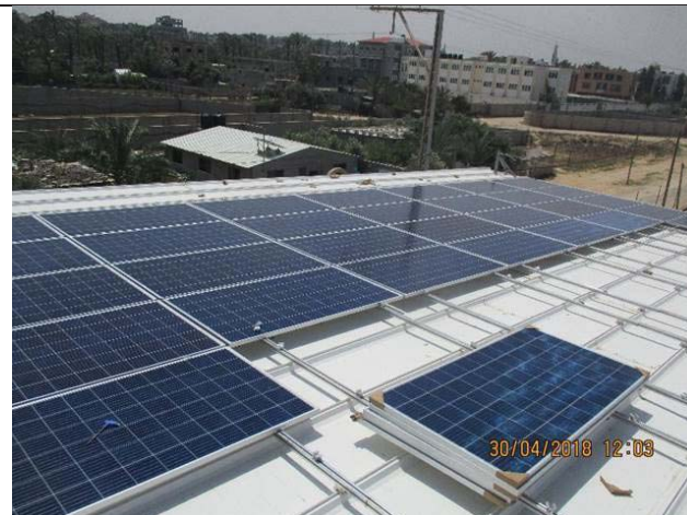
Photo No.41: PV panels installation for generator canopy Date: April 30, 2018
