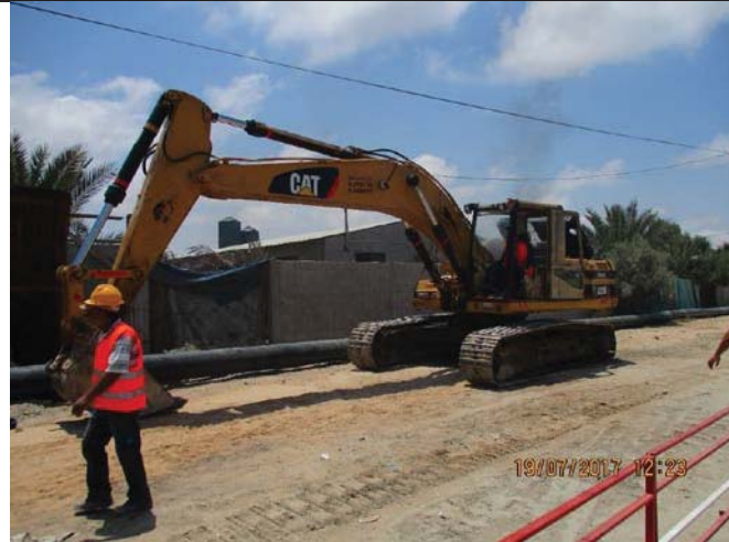
Photo No.25: Preparation for pipeline trench excavation. Date: July 19, 2017
