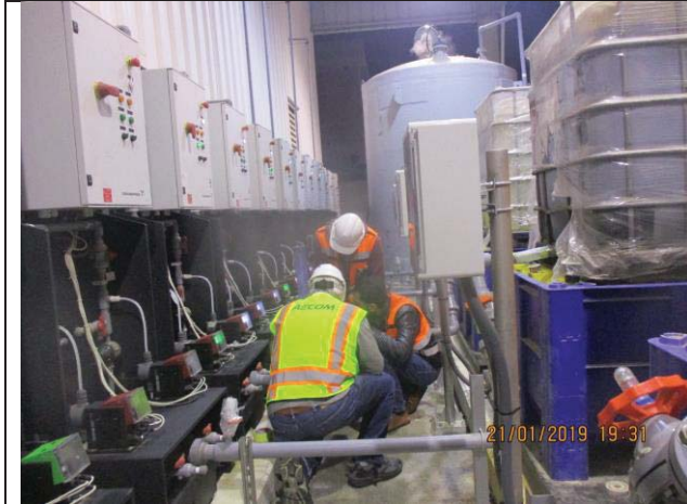
Photo No.13: Chemical skid preparation before running Date: January 21, 2019
