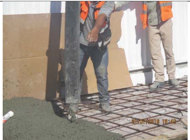
Photo No.24: Casting concrete for stair case pad. Date: July 21, 2018
