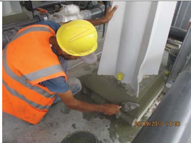
Photo No.11: Grouting works for DMF tanks Date: September 09, 2018
