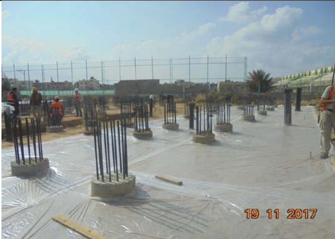
Photo No. 23: Preparing for casting concrete Date: November 19, 2017
