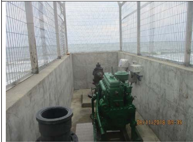
Photo No.03: Preparation for flushing and disinfection Date: November 06, 2018
