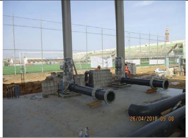
Photo No.38: Mechanical installation inside construction site Date: April 26, 2018
