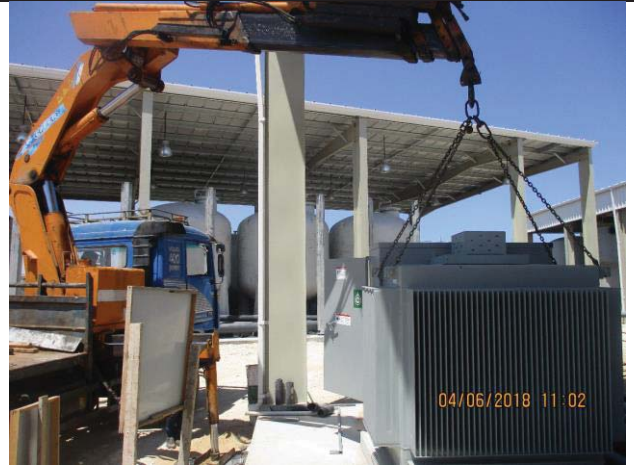
Photo No.08: Transformer installation in place Date: June 04, 2018
