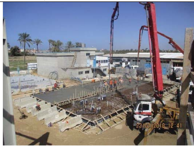
Photo No.32: Casting concrete for generator pad Date: February 22, 2018
