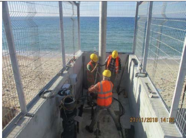
Photo No.16: Well pump installation for beach well No. 1 Date: November 27, 2018
