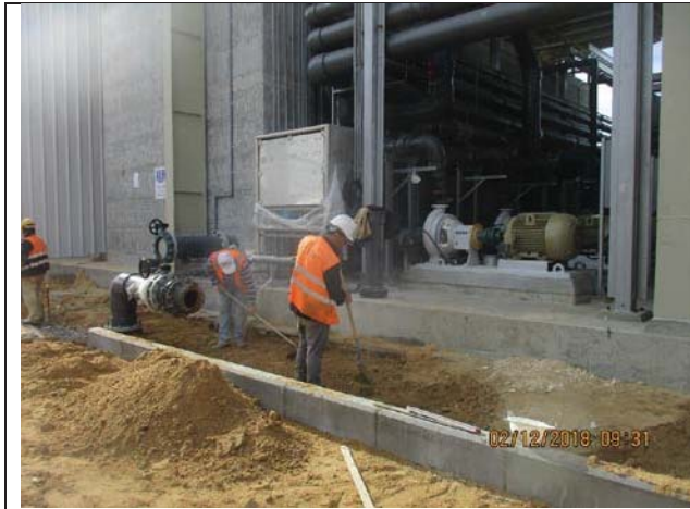
Photo No.01: Curbstone installation for site yard Date: December 02, 2018
