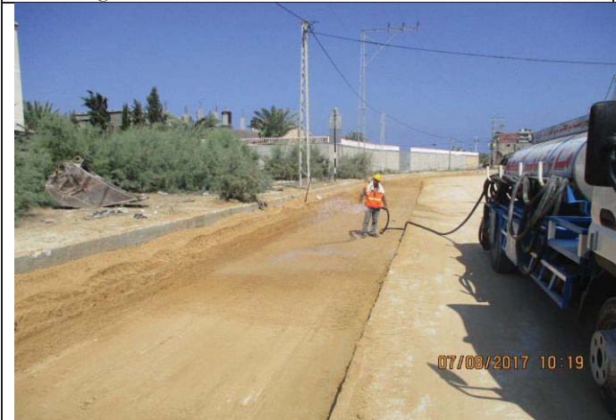
Photo No.21: Pipeline construction activities (watering prior to compaction). Date: August 07, 2017
