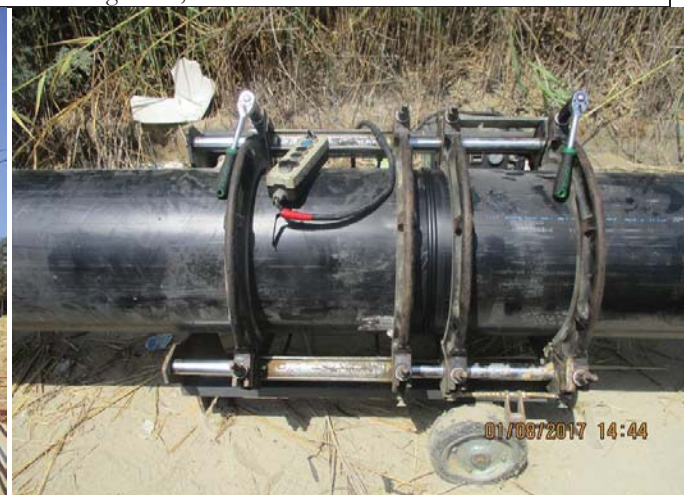
Photo No.06: Pipeline preparation activities (HDPE pipe welding). Date: August 01, 2017
