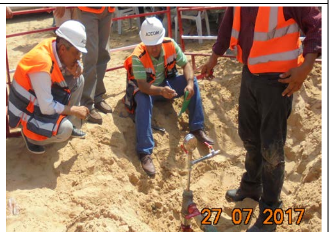
Photo No.10.2: Pipelines field leakage test. Date: July 27, 2017
