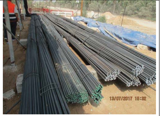
Photo No.18: Delivery of steel reinforcement at storage yard. Date: July 13, 2017
