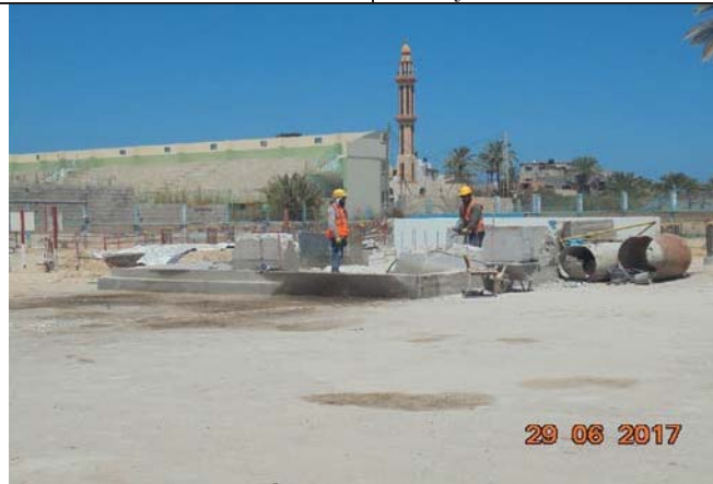
Photo No.17: Continue demolition of existing fuel tank pads. Date: June 29, 2017
