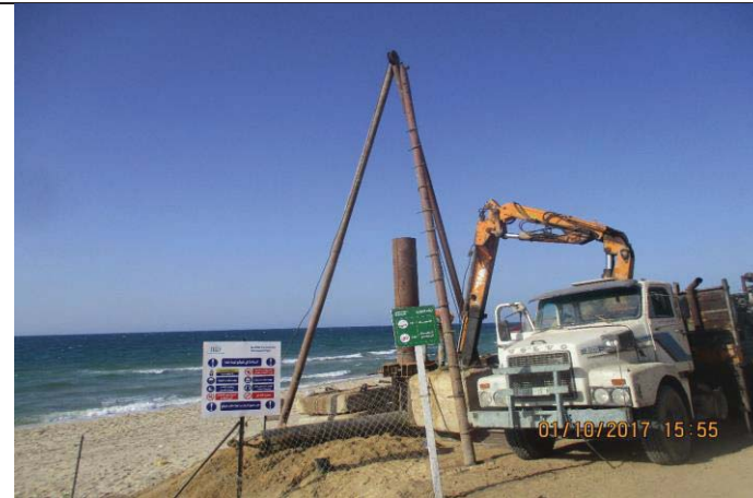
Photo No.01: Beach well construction activity (beach well No. 02) Date: October 1, 2017
