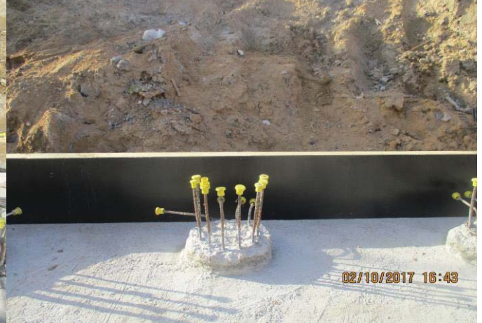
Photo No.04: Brine tank construction activity (internal formwork) Date: October 2, 2017
