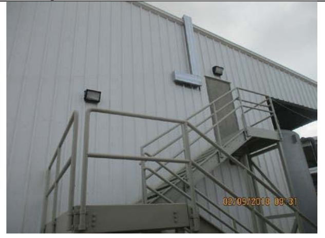
Photo No.04: Lighting fixtures installation for RO Building Date: September 02, 2018
