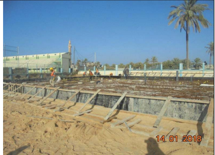
Photo No.16: Shuttering works and steel reinforcement for RO foundation (phase 2). Date: January 14, 2018
