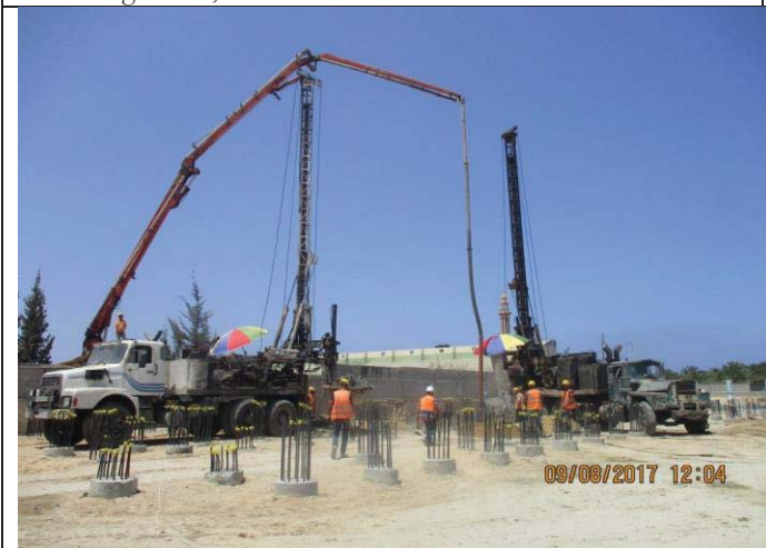
Photo No.29: Pile construction activities (drilling & casting). Date: August 09, 2017
