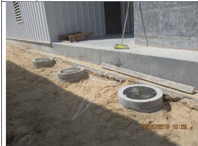
Photo No.29: Grounding manholes installation for pretreatment area. Date: May 29, 2018
