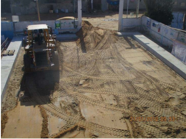
Photo No.27: Backfilling works for workshop area.
