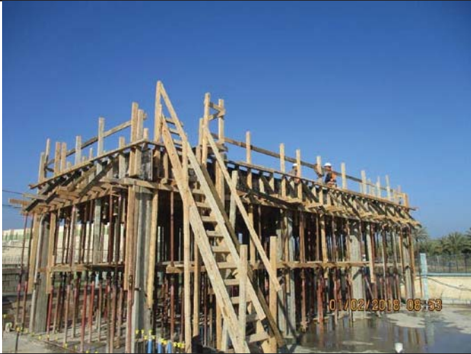
Photo No.01: Electrical room at RO building
