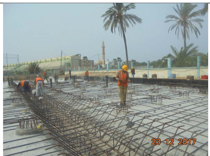
Photo No.46: Excavation works and steel reinforcement for piles Date: December 23, 2017
