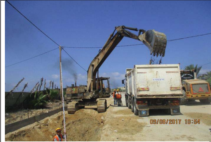
Photo No.25: Pipeline construction activities (trench excavation works). Date: August 09, 2017
