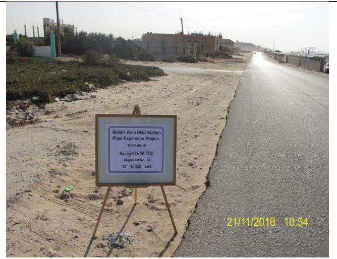
Photo No.02: Dilapidation survey Date: November 21, 2016
