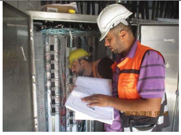
Photo No.10: Electrical works inside electrical room Date: September 08, 2018
