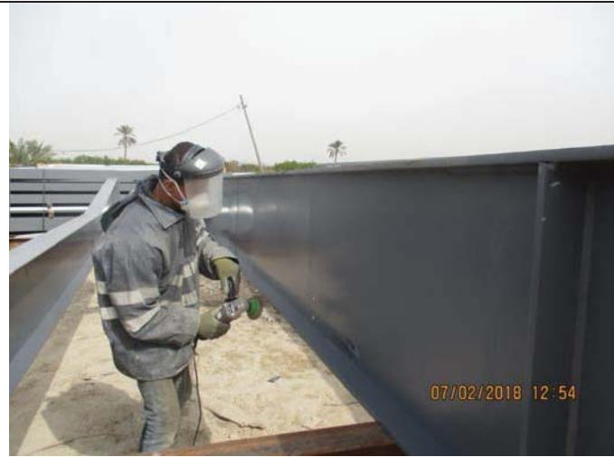
Photo No.12: Preparation works for steel structure before coating Date: February 07, 2018
