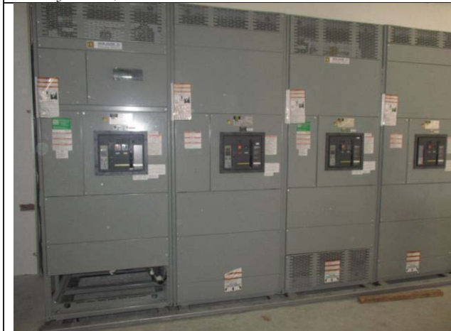
Photo No.23: Installing the SWBD panels Date: June 23, 2018
