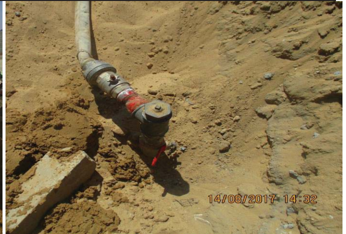
Photo No.34: Pipeline construction activity (pressure test preparation works) Date: August 14, 2017
