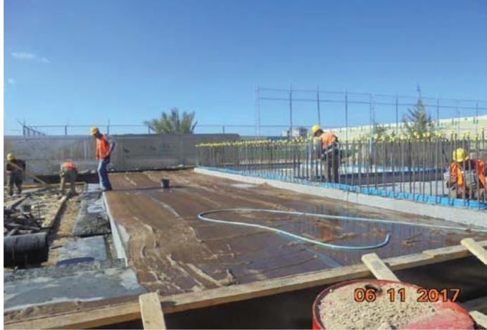
Photo No. 10: Raw water and backwash tanks foundation, curing.
