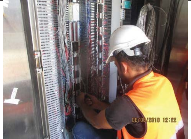
Photo No.14: Electrical works in electrical room Date: August 08, 2018
