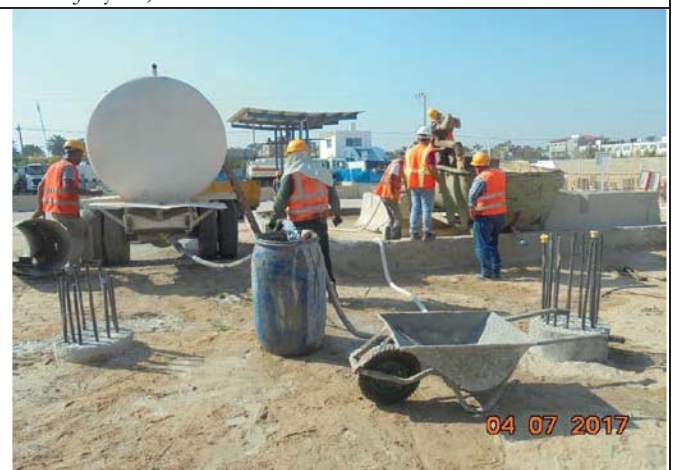
Photo No.06: Mixing Bentonite with water. Date: July 04, 2017
