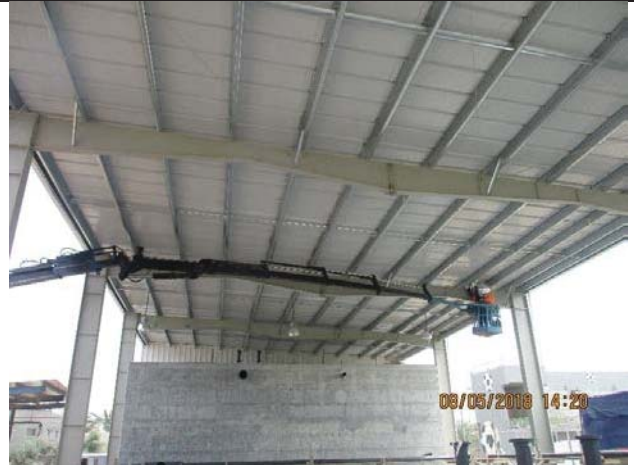
Photo No.10: Electrical installation inside pretreatment building Date: May 08, 2018
