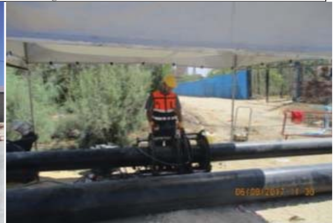
Photo No.16: Continue pipeline preparation – welding pipes (450 mm & 315 mm). Date: August 06, 2017
