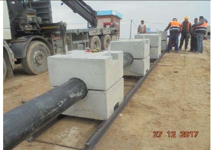
Photo No.50: Trial run for outfall pipeline installation Date: December 27, 2017
