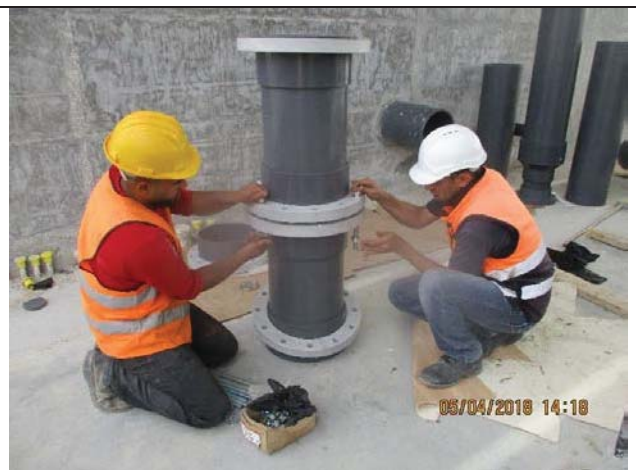
Photo No.12: Preparation for mechanical works Date: April 05, 2018
