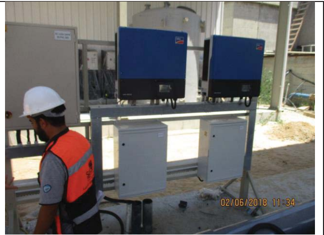
Photo No.02: Inverter installation in generator. Date: June 02, 2018
