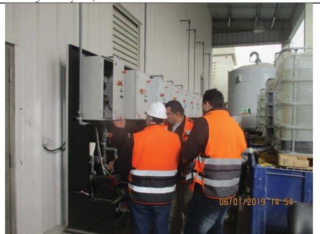
Photo No.06: Functional test for the chemical feed system Date: January 06, 2019
