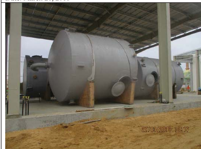
Photo No.27: Chemical tanks delivered to site Date: March 27, 2018
