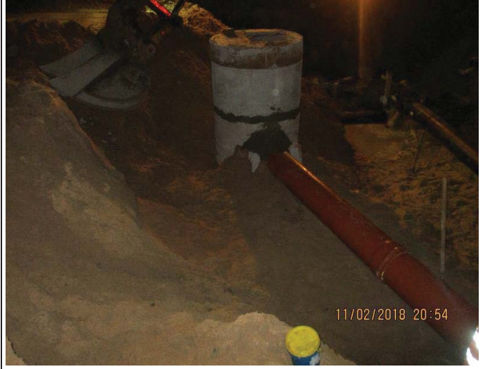
Photo No.18: PVC pipes installation for brine discharge line Date: February 11, 2018
