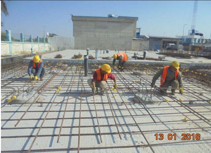
Photo No.15: Steel reinforcement works for RO foundation (phase 2). Date: January 13, 2018
