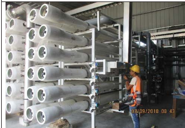
Photo No.05: Connection works for instrumentation Date: September 03, 2018
