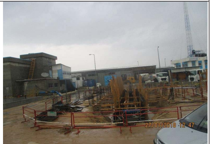
Photo No.36: No site activities due to heavy rain. Date: January 27, 2018
