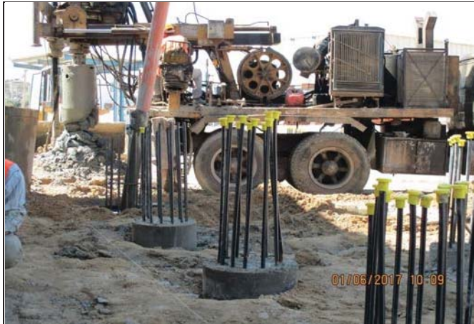
Photo No.01: Pile casting at the new RO building area.
