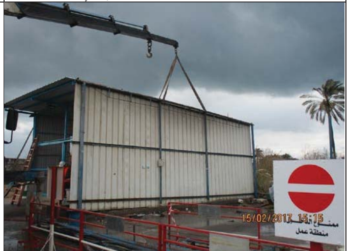
Photo No.14: Demolition of steel canopy structure Date: February 15, 2017
