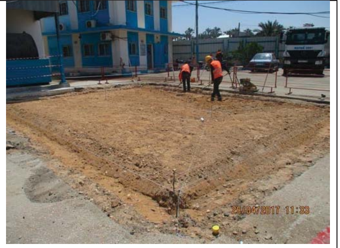
Photo No.24: Continue fuel tank relocation activities Date: April 29, 2017
