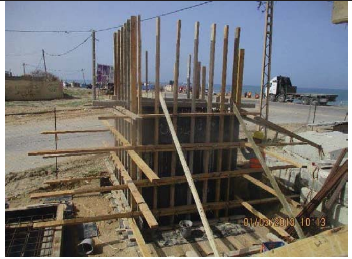
Photo No.02: Shuttering and reinforcement works for mechanical chambers
