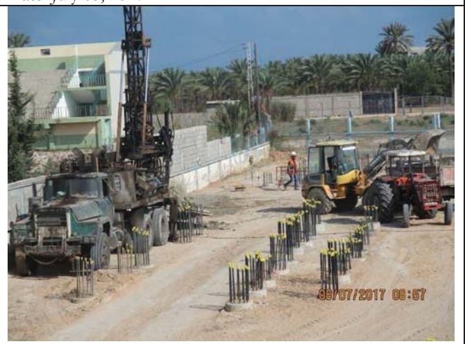
Photo No.12: Pile construction activities using Bentonite. Date: July 08, 2017
