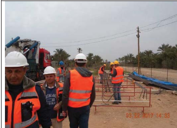
Photo No.21: Fabricating reinforcement steel case at storage yard. Date: March 22, 2017
