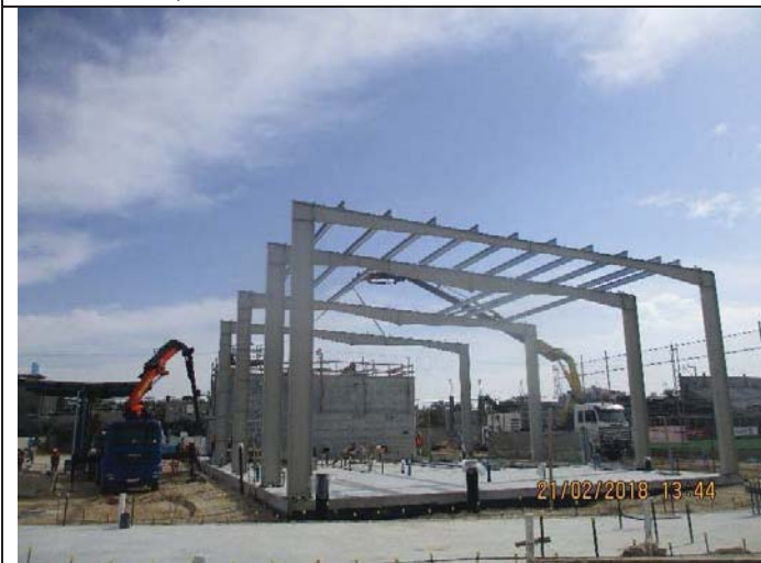
Photo No.31: Continue erection works for pretreatment steel structure Date: February 21, 2018
