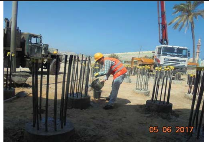
Photo No.04: Curing previously casted piles.
