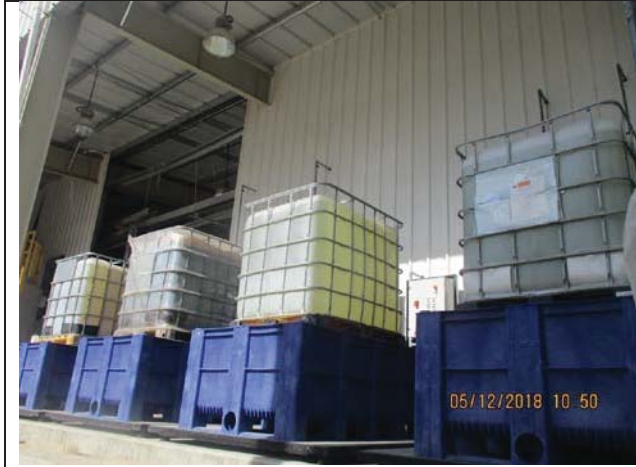
Photo No.07: Chemical tanks installation on chemical area Date: December 05, 2018
