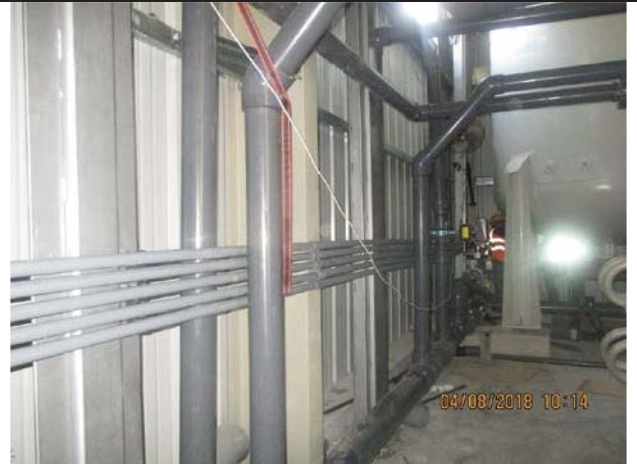
Photo No.06: Chemical pipes installation Date: August 04, 2018
