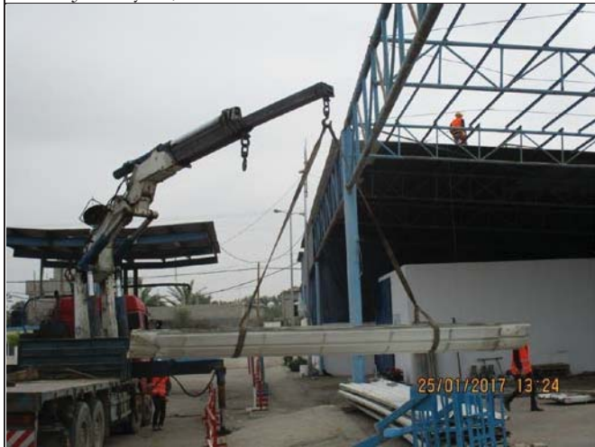
Photo No.07: Demolition of existing steel canopy structure. Date: January 25, 2017
