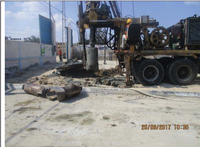
Photo No.31: Pile construction activity (workshop area) Date: September 20, 2017
