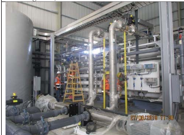
Photo No.23: Mechanical works in 2 nd pass. Date: August 27, 2018
