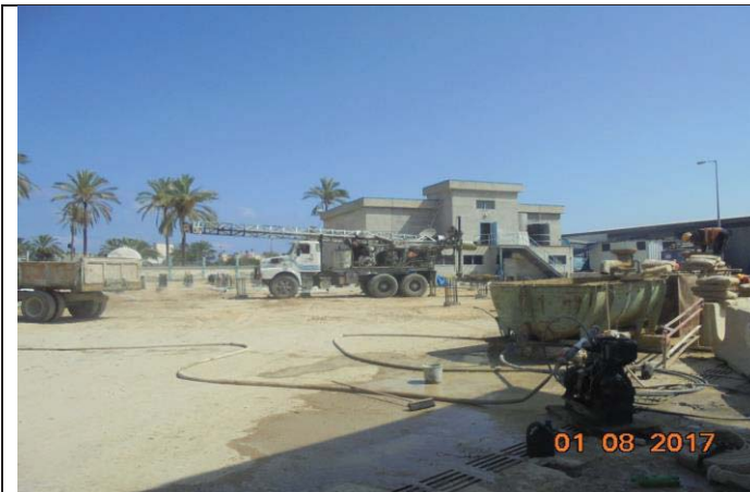
Photo No.01: Pile construction activity (generator pad). Date: August 01, 2017
