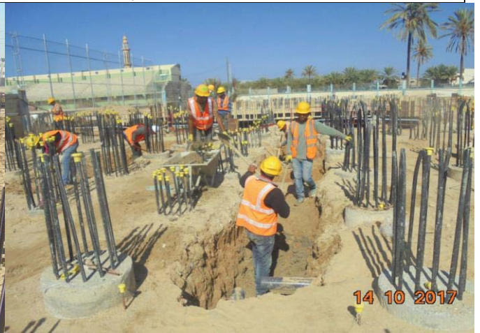
Photo No.22: Trench excavation in pre-treatment building. Date: October 14, 2017
