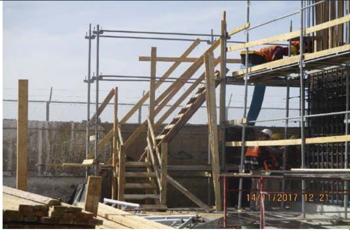
Photo No. 16: Raw water and backwash tanks formwork and steel formation.
