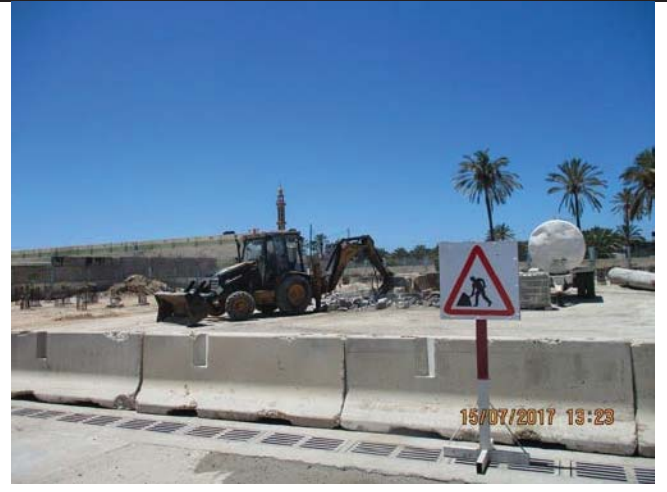
Photo No.20: Demolition of existing diesel fuel tank pads. Date: July 15, 2017
