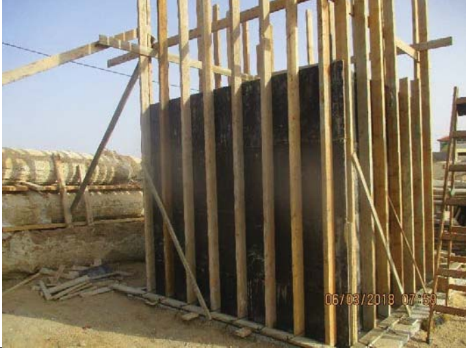
Photo No.05: Shuttering and reinforcement works for mechanical chambers Date: March 06, 2018
