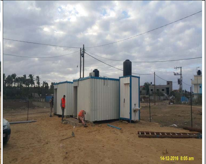
Photo No.10: Containers installation for contractor site office, guardroom & portable WC
