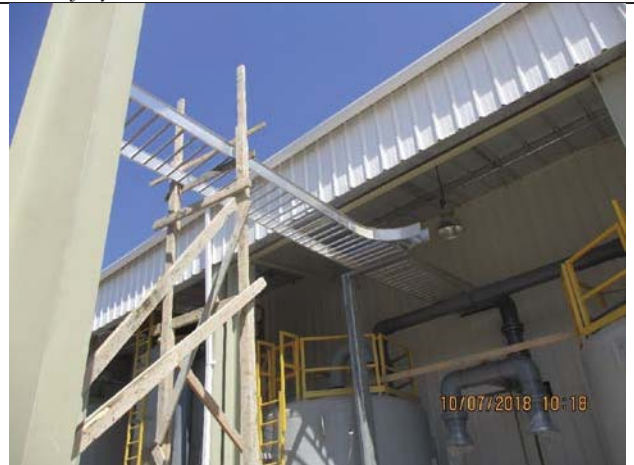
Photo No.12: Cable tray installation Date: July 10, 2018
