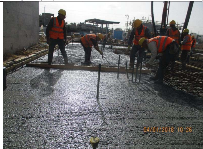
Photo No.04: Casting concrete for RO building foundation (phase 01). Date: January 04, 2018
