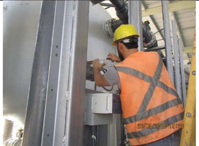
Photo No.26: Connection works for instruments Date: August 28, 2018
