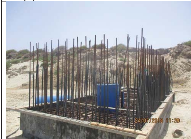
Photo No.29: Concrete pad for beach well No.1
