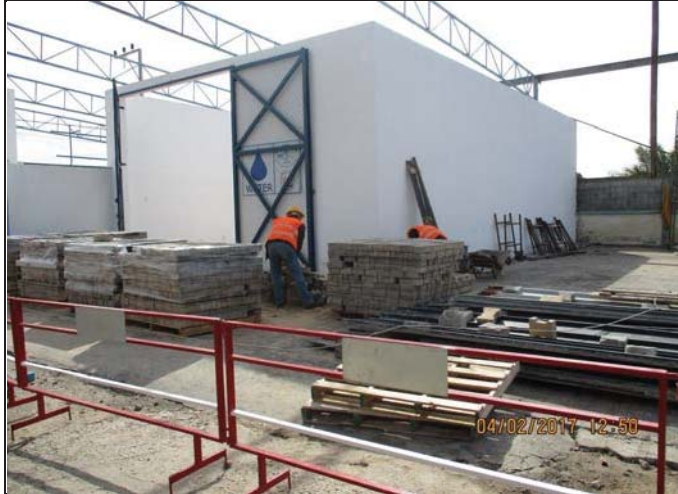
Photo No.05: Continue interlocks demolition.
