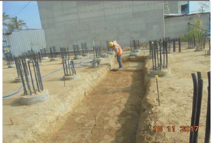
Photo No. 20: R.O building – excavation for electrical trench. Date: November 18, 2017
