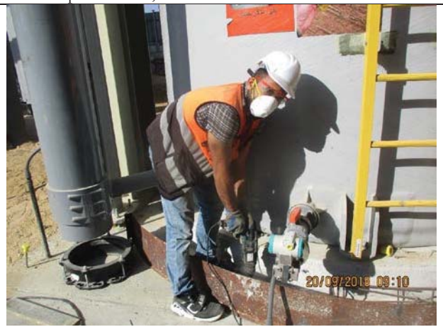
Photo No.24: Connection works for instruments Date: September 20, 2018
