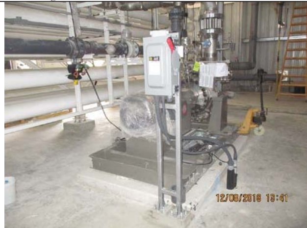
Photo No.17: Connection works for instruments Date: August 12, 2018
