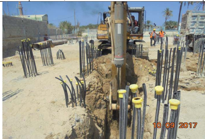
Photo No.17: Structural excavation (excavation for brine tank) Date: September 10, 2017
