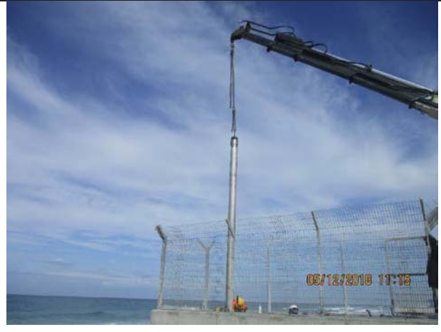
Photo No.08: Installation works for beach well No. 3 Pump Date: December 05, 2018
