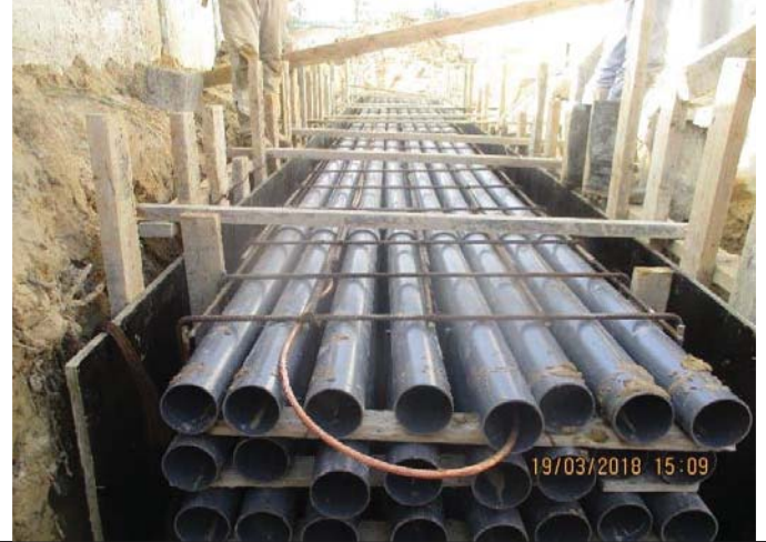
Photo No.18: Electrical conduits installation for duct bank No. 18. Date: March 19, 2018
