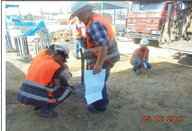
Photo No.03: RO building piles center allocation.
