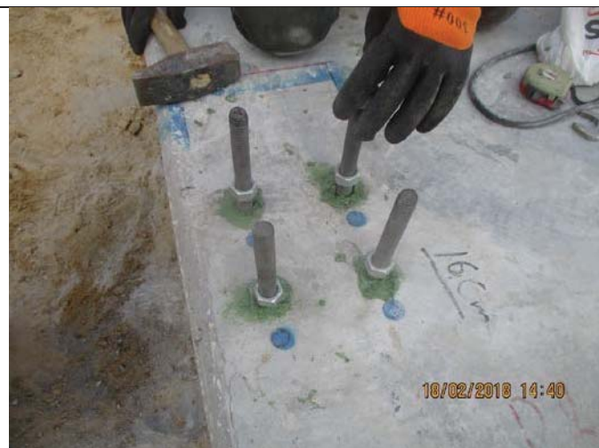
Photo No.26: Install anchor bolts for pretreatment steel structure. Date: February 18, 2018
