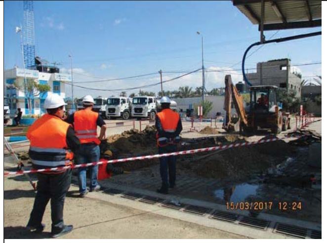
Photo No.12: Start storm water catchment relocation. Date: March 15, 2017
