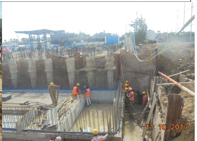
Photo No.16: Brine tank area - cleaning work. Date: October 11, 2017
