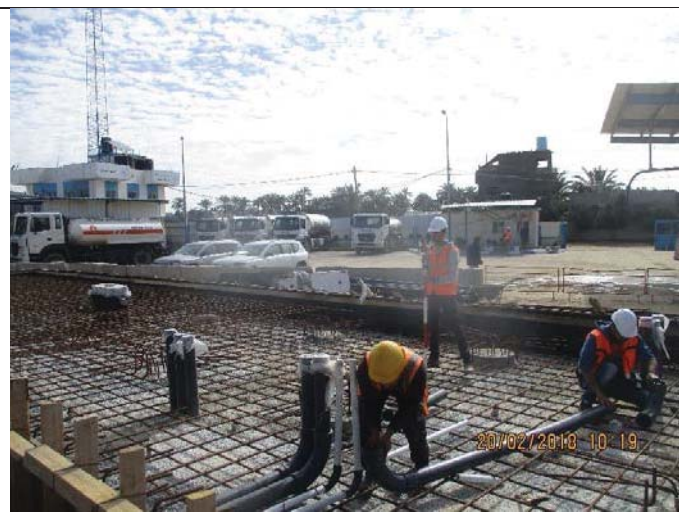
Photo No.30: Electrical conduits installation for generator pad. Date: February 20, 2018
