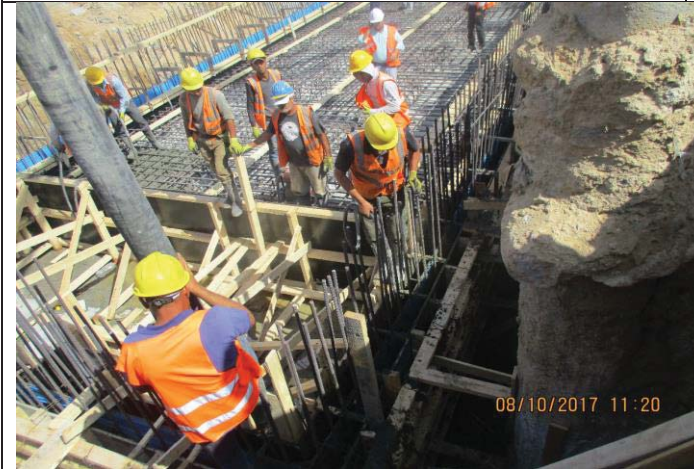
Photo No.11: Brine tank construction activity (concrete casting) Date: October 8, 2017
