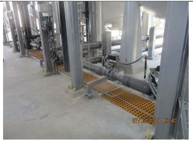
Photo No.30: FRP grating installation for pretreatment area Date: September 27, 2018
