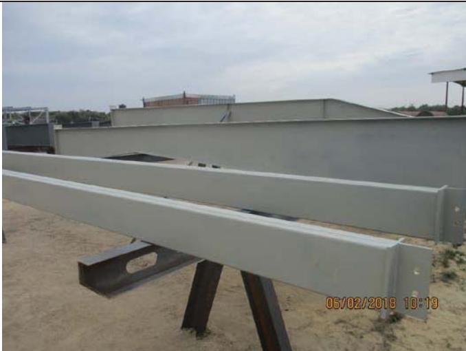
Photo No.11: Continue epoxy coating for steel structure Date: February 06, 2018
