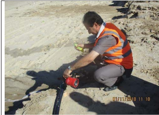
Photo No.01: Disinfection for Beach Well No. 1 Date: November 01, 2018
