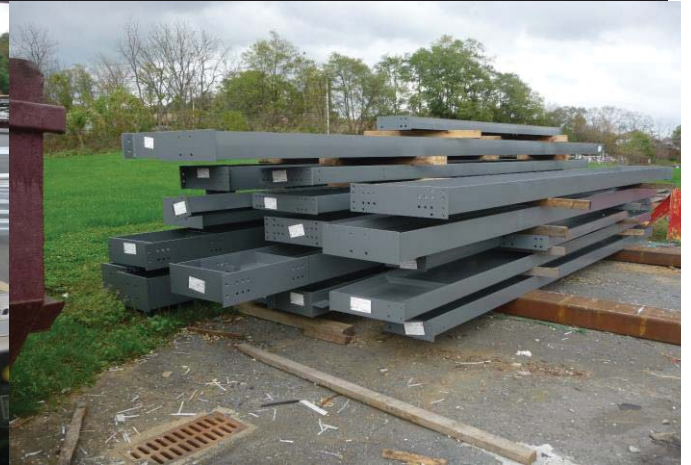
Photo No.50: Pre-engineered steel structure: fabrication, painting and packing. Date: October 25, 2017
