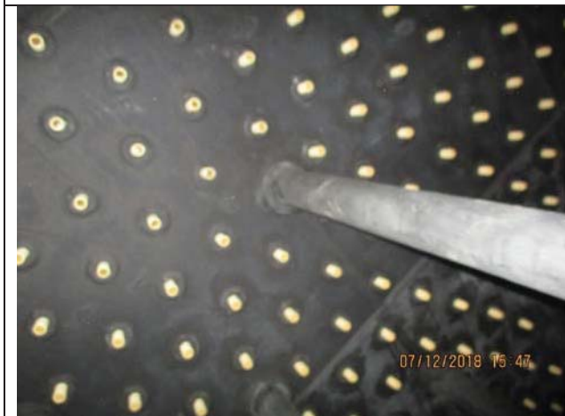
Photo No.11: Nozzles installation in filter tanks Date: December 07, 2018
