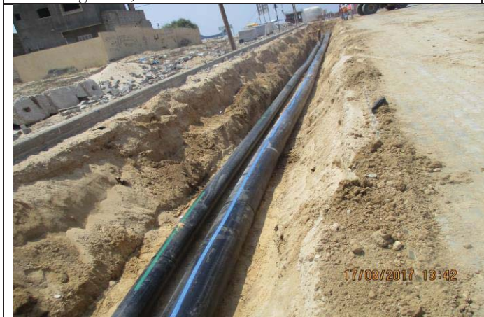
Photo No.41: Pipeline construction activity (trench excavation). Date: August 17, 2017
