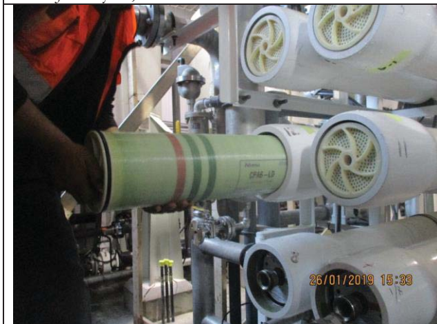
Photo No.21: Membrane loading for the 2 nd pass Date: January 26, 2019
