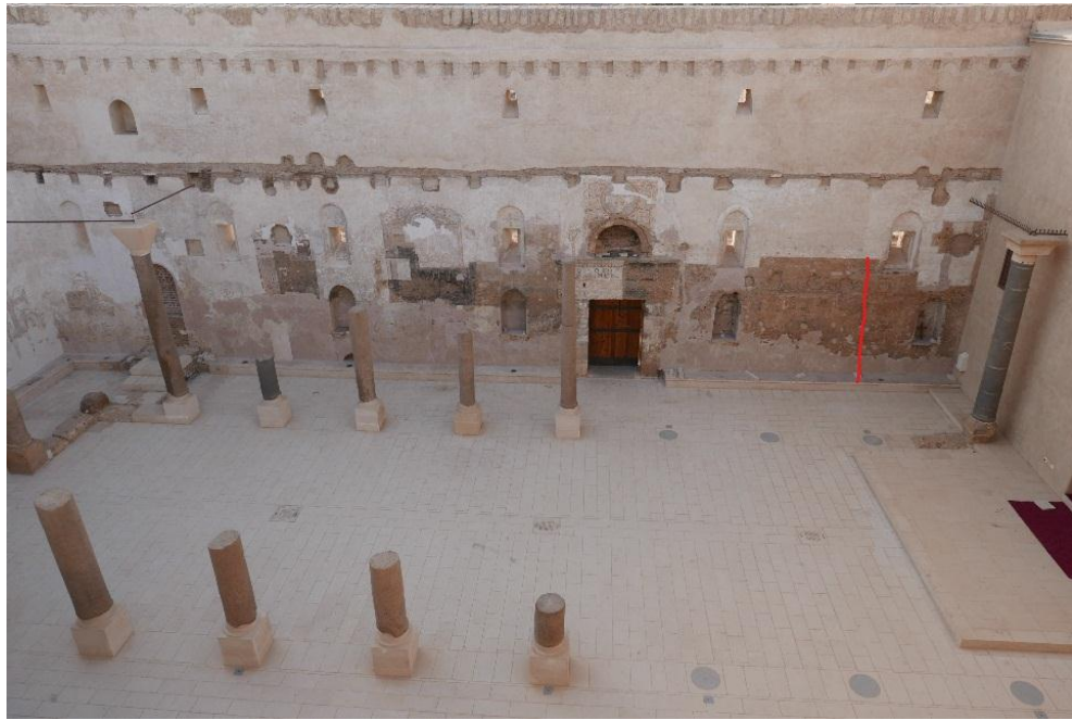
Figure 6: View of the Nave walls after the Spring 2018 campaign
