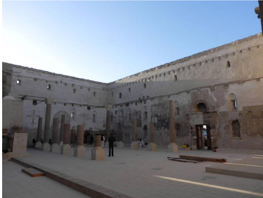
Figure 5: View of the Nave walls after the Fall 2017 campaign
