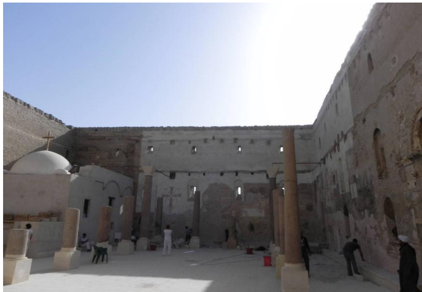
Figure 4: View of the Nave walls after the Spring 2017 campaign
