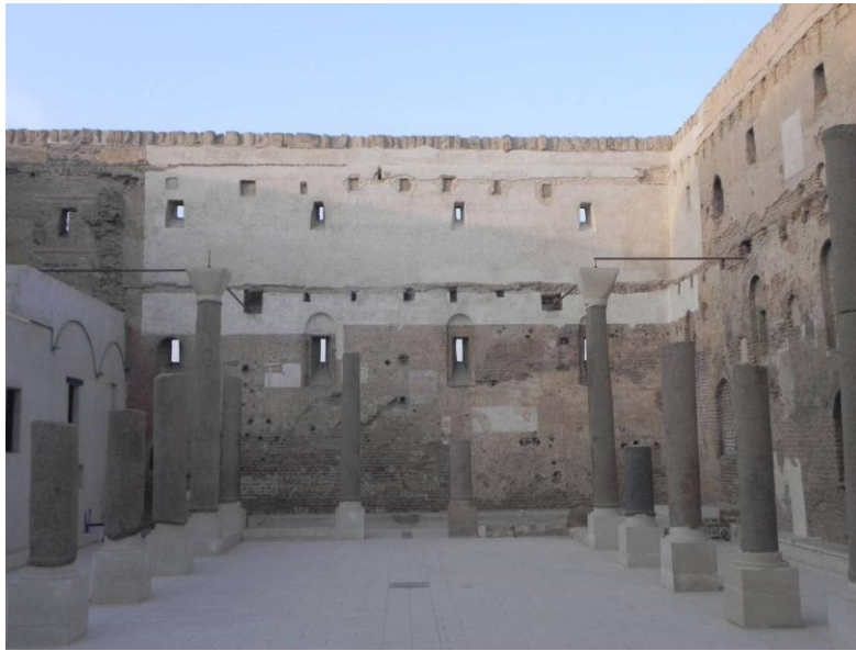
Figure 3: View of the Nave walls after the Fall 2016 campaign
