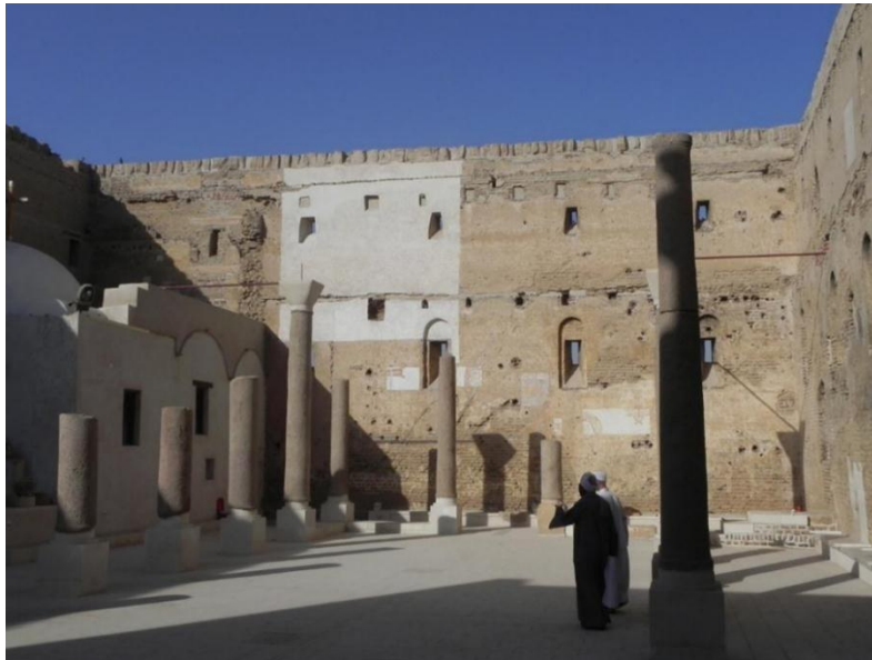
Figure 2: View of the nave walls after Spring 2016 campaign
