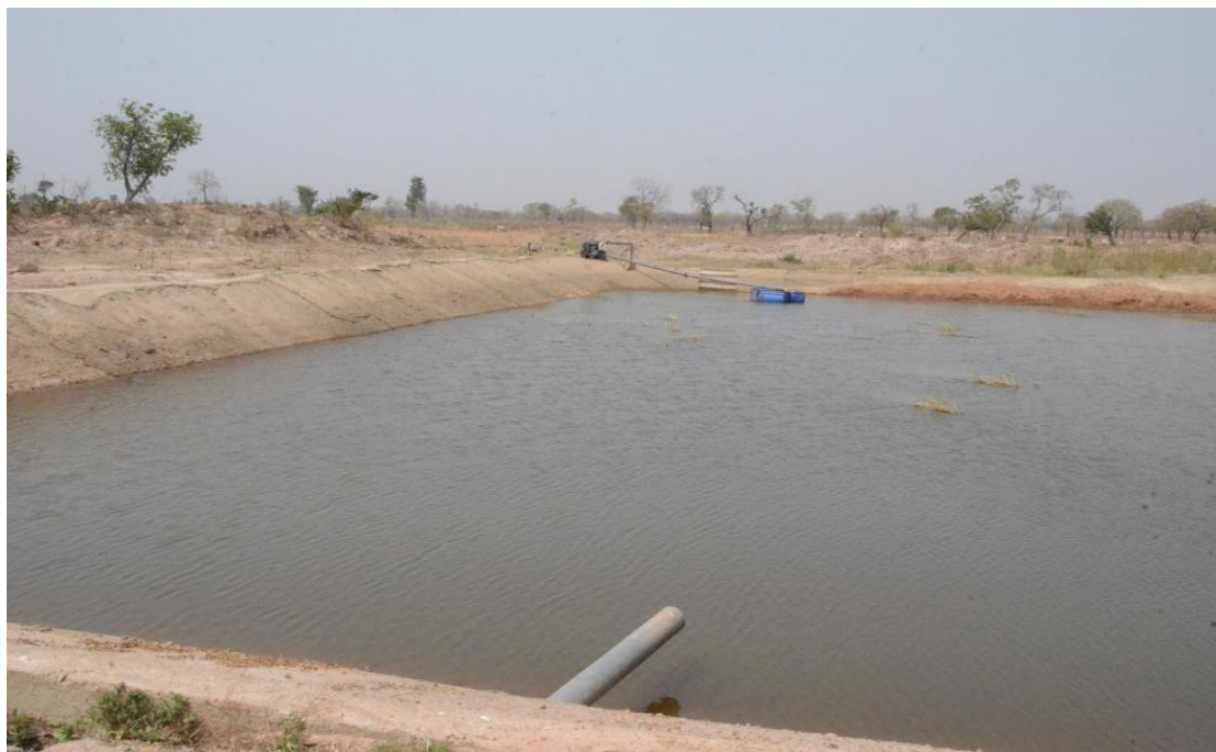
Wambong Dam Irrigation Facility after rehabilitation
