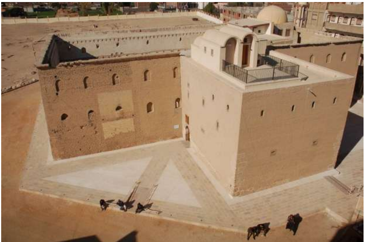
Figure 6: Completed hard landscaping on the south side of the church and tower [Photo: N. Warner, 2018]
