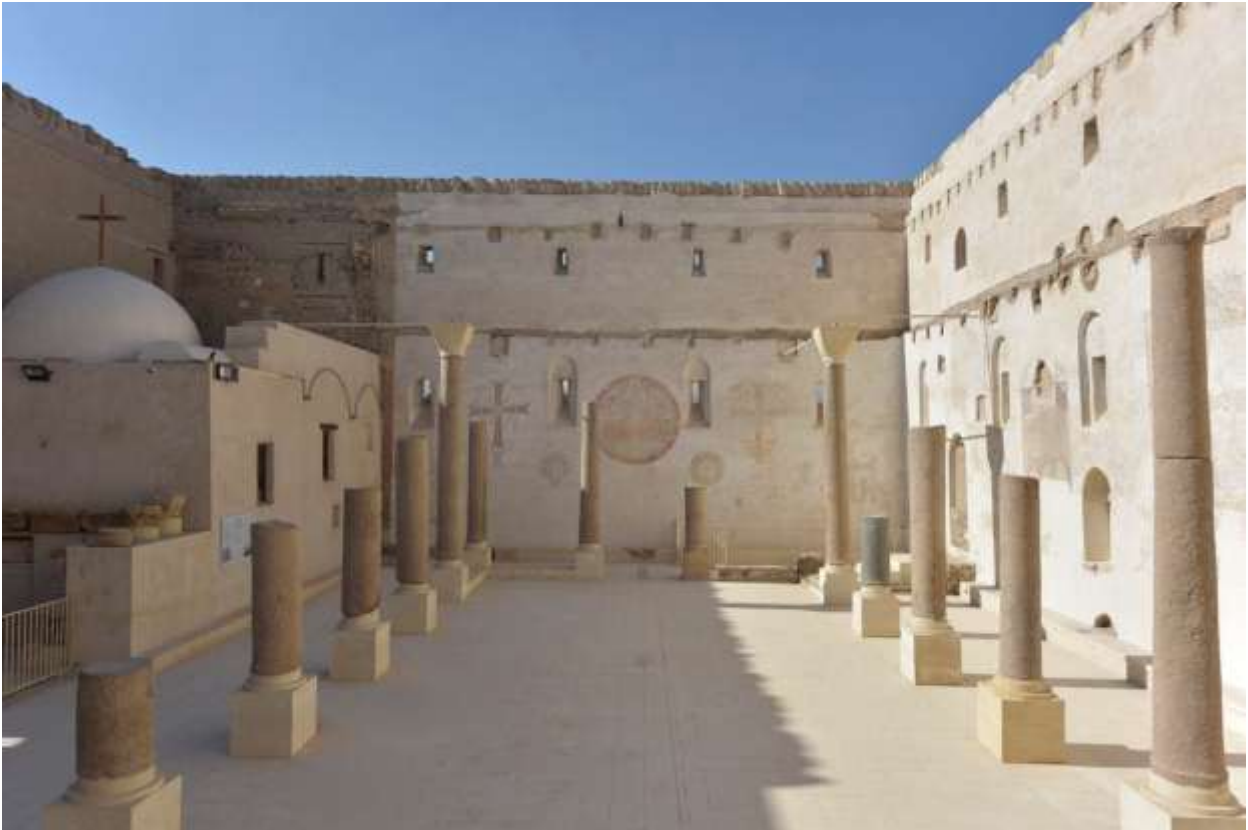
Figure 5: The nave looking west after anastylosis of columns and conservation of wall-paintings
