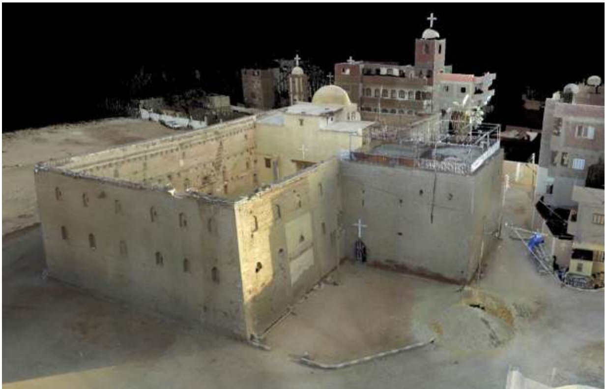
Figure 2: View of the Red Monastery church and tower from southeast in 2015 with monastic rest-house behind (image generated by 3D Laser Scan by P. Gasparri)
