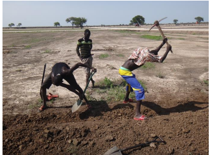
Laborers digging tertiary drains in Bentiu PoC (UNI030)
