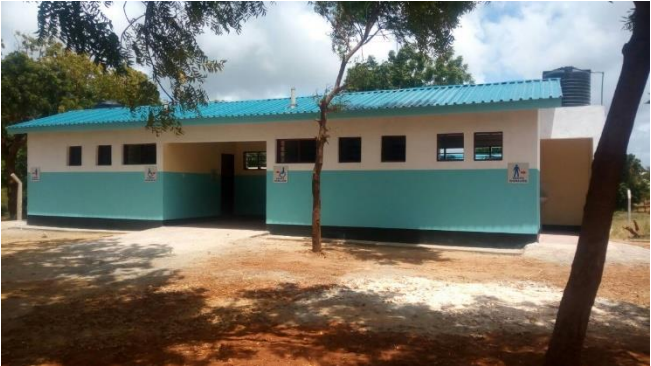
Gongoni six-door VIP latrine
