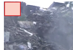
e) Many houses were destroyed by hurricanes.
