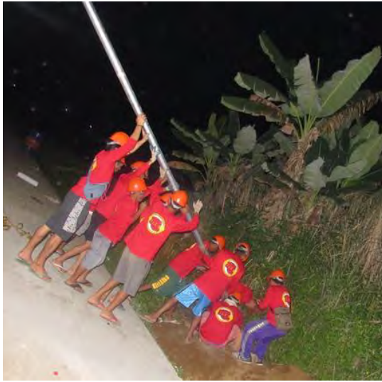
Installation of solar PV streetlights at Sagonsongan temporary shelter in Marawi City. Photo credit by B-LEADERS.
