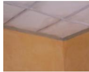
Room after renovation
