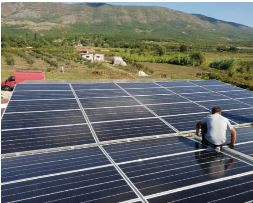
Rapsodia agribusiness undergoes solar panel installation
