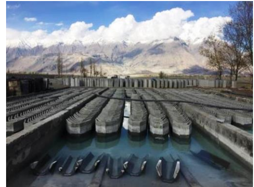
PSPS Segments Ready at PCPS Yard Skardu
