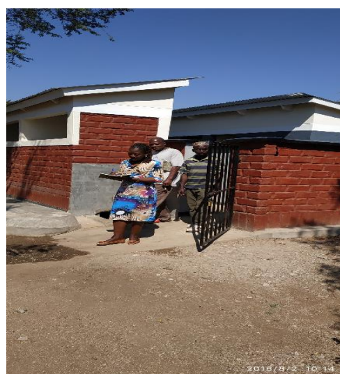
USAID's WASH Specialist inspecting a latrine block at Kafulafula in Balaka
