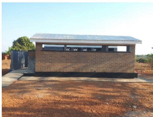
A latrine block at Likangala Primary School, in Zomba that had no defects after six months.
