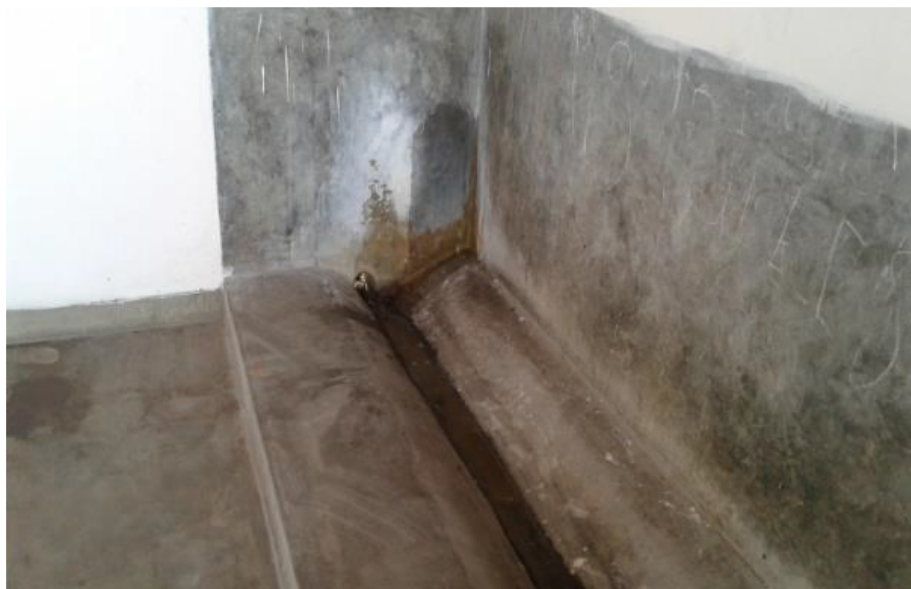
Figure 6:1: Detail of male urinal channel
