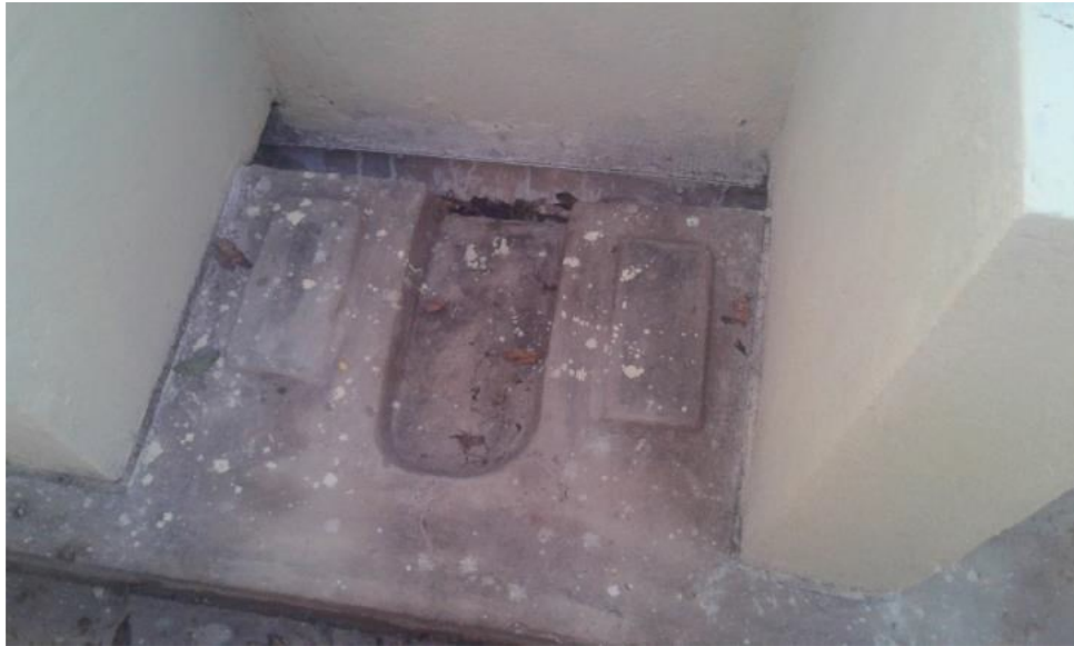
Figure 6:2: Detail of female urinal channel and partition
