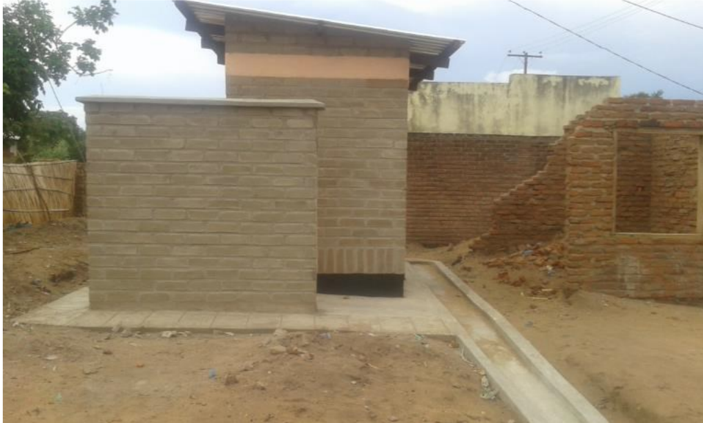
Figure 5:3: A storm drain
