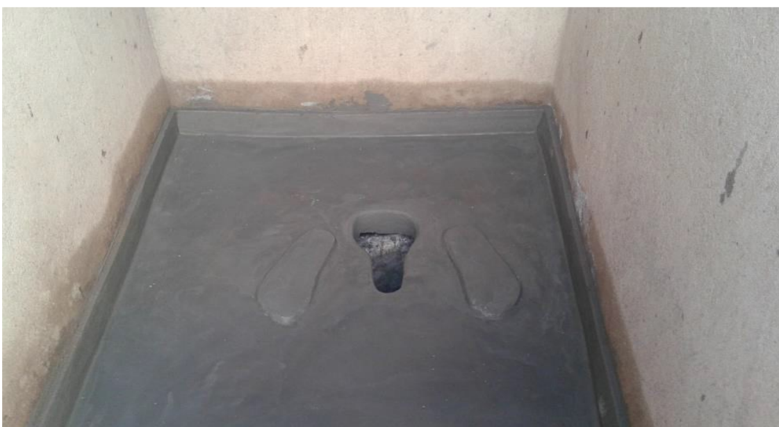
Figure 5:1: A new san plat (made in Liwonde) fitted over the old slab/drop hole
