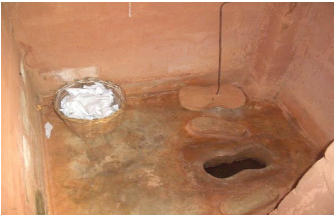
Figure 5:1: A new san plat (made in Liwonde) fitted over the old slab/drop hole
