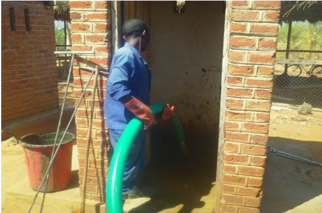
Figure 5:4: Desludging in process
