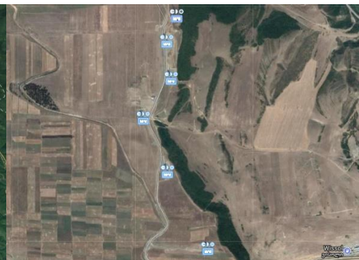
Picture 2: Qartli Wind Farm
