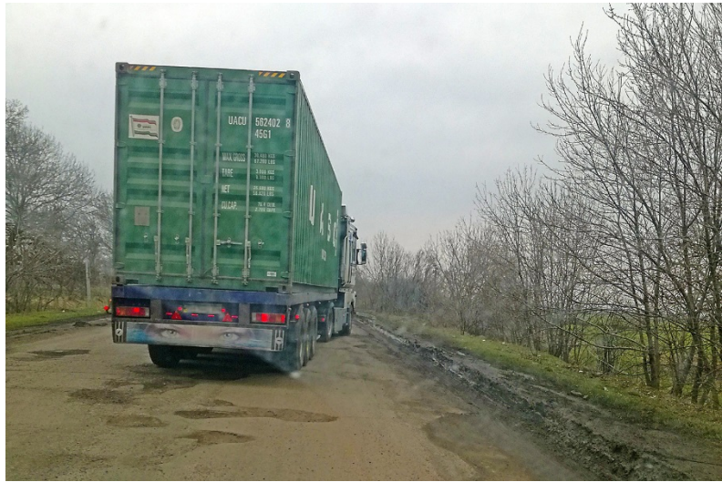
Road conditions on Route E87 from Chişinău to Odessa.
