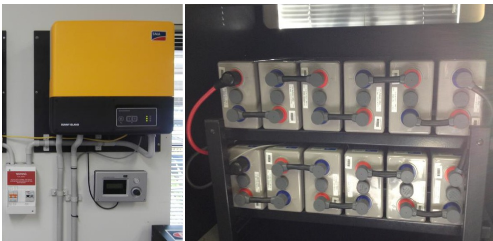
Figure 22: Grid-connected multimode inverter and storage battery
