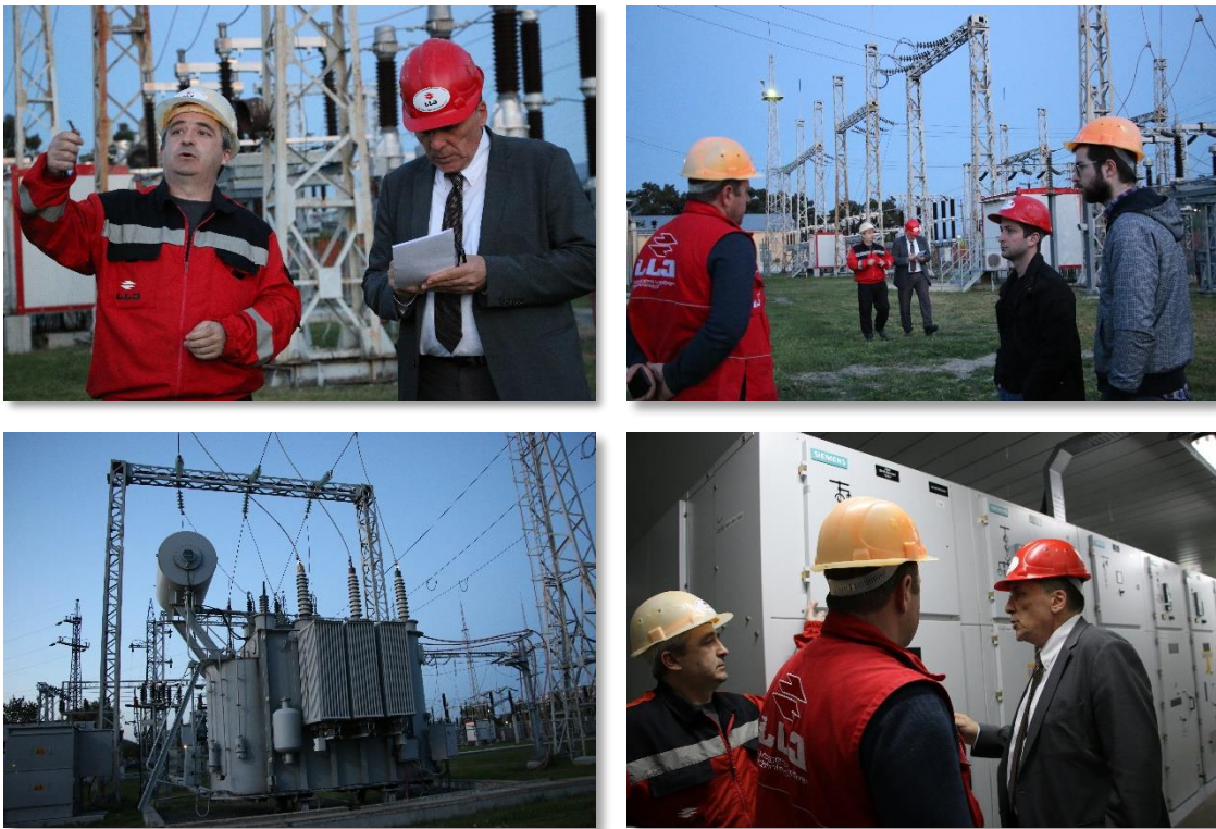
USAID Energy Program visiting GSE substation Gori 220kV
