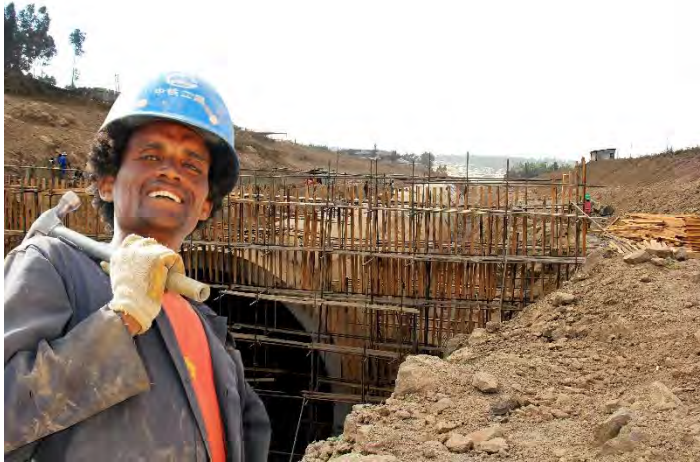
An employee working in irrigation construction at a MULU Worksite
