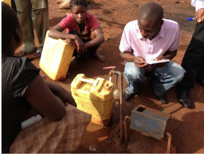
Figure 4.2.3 Metered public standpipe at Ki-Karamoja
