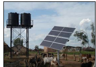
High volume solar-powered water supply provides populations returning from prolonged conflict with water for drinking and agriculture
