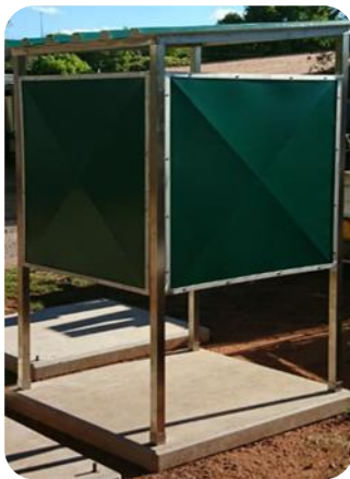
Figure 17: Naturally ventilated outdoor sputum booth
