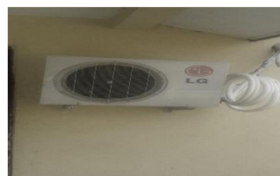
Newly installed 2 HP AC in the laboratory
