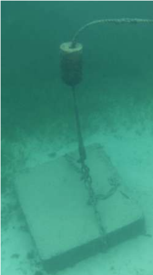
Figure 25. Image showing concrete block anchor with chain and float that is preventing scouring of the surrounding seabed (Reed, 2016).
