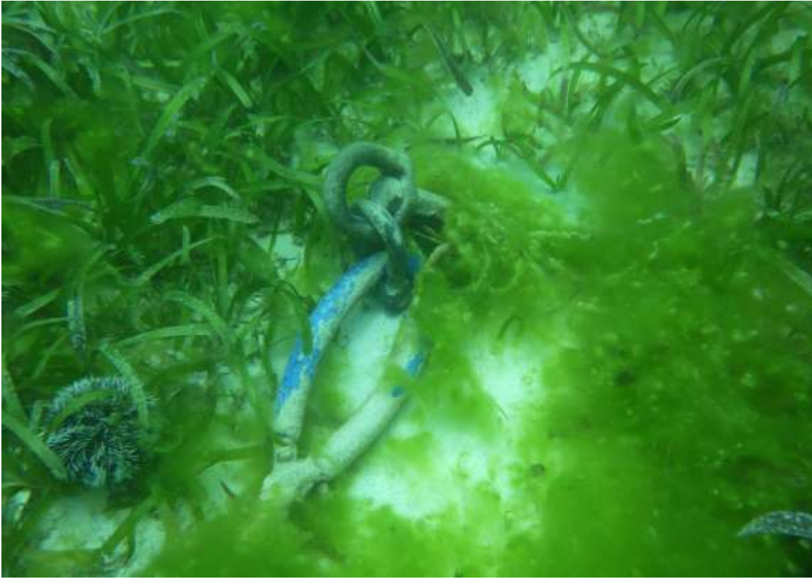
Figure 20. Image showing a single manta pin anchor with downline attached, surrounded by seagrass and green algae (Reed, 2016).
