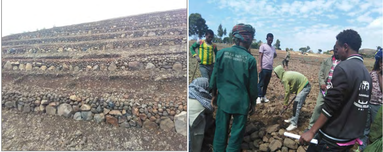
Figure 1: Stone bund and trench construction in PW (Simada woreda)
