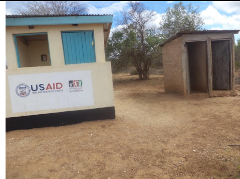
Latrines at Chewele Primary School
