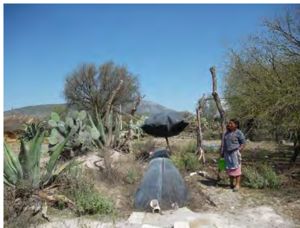
Figure 6: Typical domestic scale biodigester installed by Sistema Biobolsa in the state of Hidalgo with funding from SEMARNAT (PESA).
