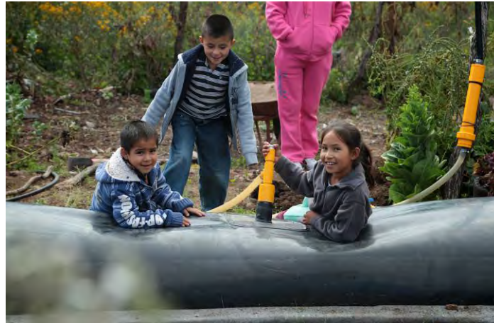
Image 2: Tubular modular polyethylene biodigester installed in a backyard farm as part of the Strategic Food Security Program (PESA) run by the Secretary of Agriculture and Rural Development (SAGARPA) in the state of Hidalgo.
