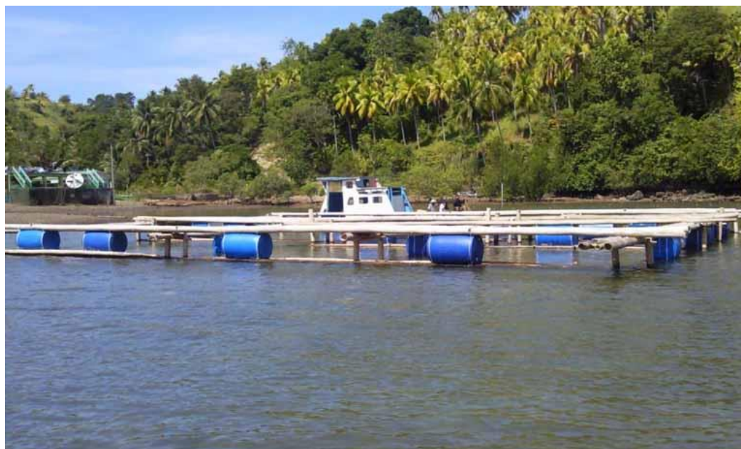
All-weather resilient 8-compartment floating fish cage module (photo courtesy of C. Andigan)
