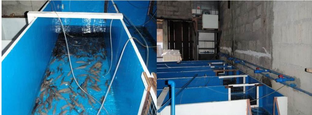
Small-scale fish consolidation station, with holding tanks equipped with aeration, filtration, and water supply systems
