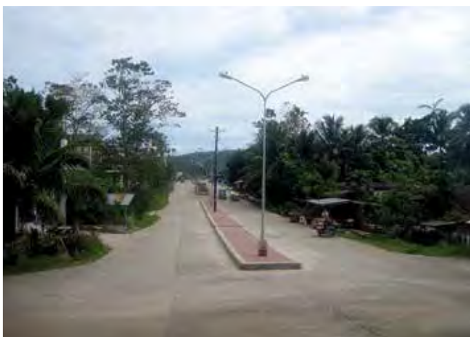
REAP incentives consisted of infrastructure projects.
