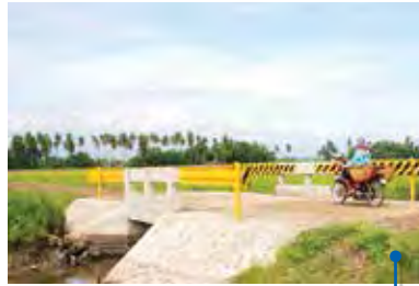
Laguinding Barangay Bridge Esperanza, Sultan Kudarat
