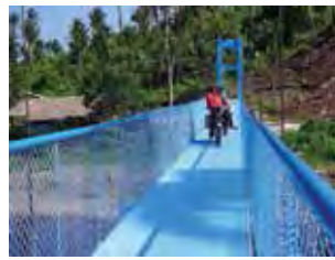
San Jose Suspension Footbridge in Boston, Davao Oriental
