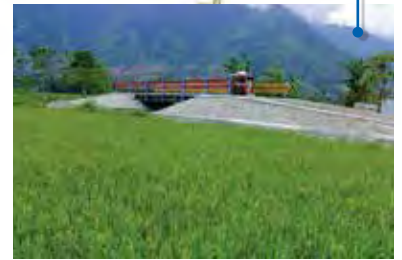
Mangilala Barangay Bridge Isulan, Sultan Kudarat
