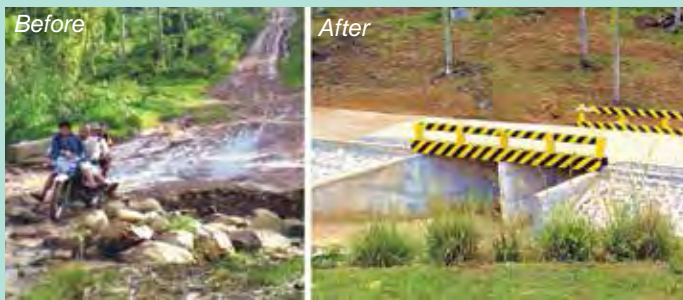
Kabug-Kabug Barangay Bridge, North Upi, Maguindanao
