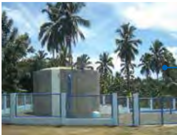
Jolo Water Supply Upgrading Jolo, Sulu
