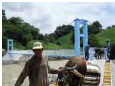
Barangay Bridge in Sultan Kudarat
