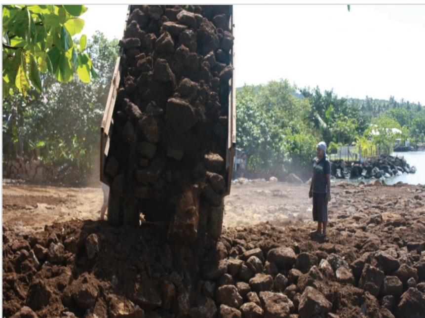
Samoa: Rising sea level requires coastal communities to develop adaptation methods, such as using construction rocks to protect the villages.
