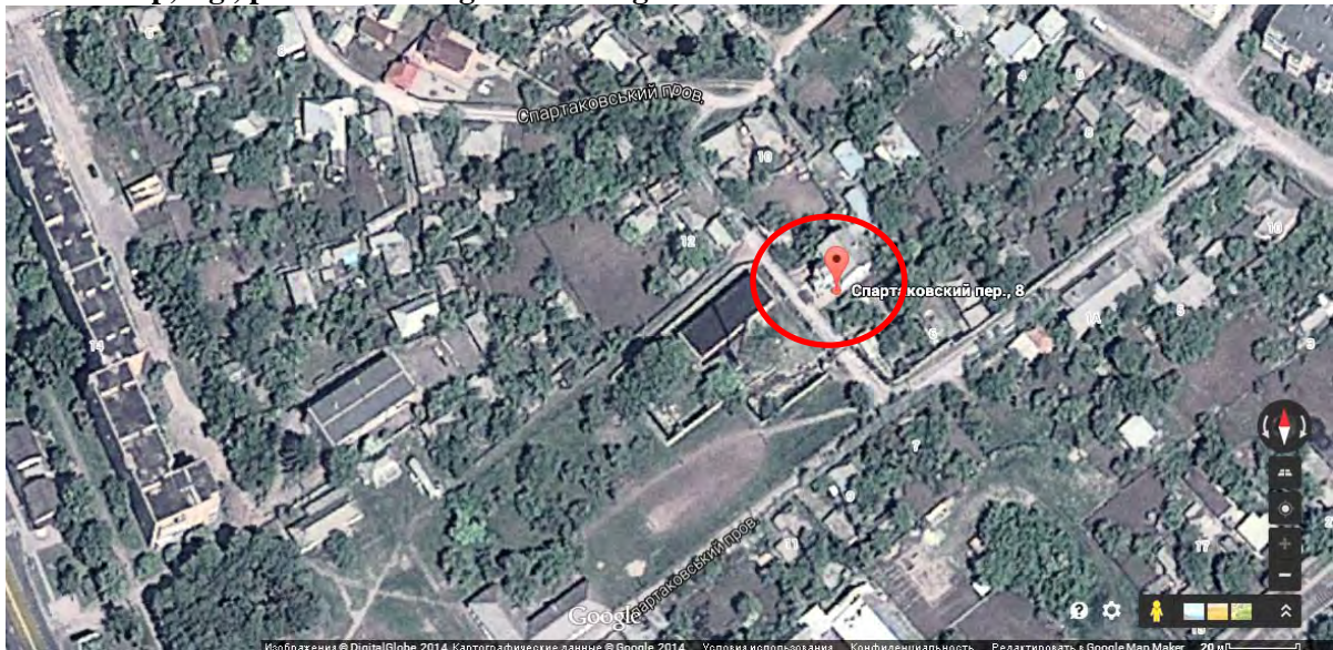
Picture 2. Location of the gas boiler house, 8, Spartakivsky Provulok, Myrhorod.
