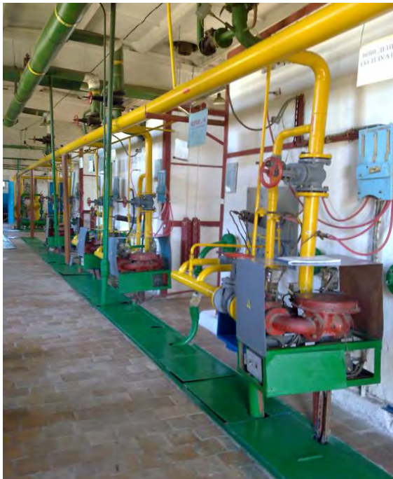
Picture 6. Existing gas boilers (produced in 1987, efficiency 80%)
