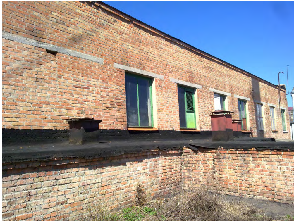
Picture 4. Existing gas boiler house building.
