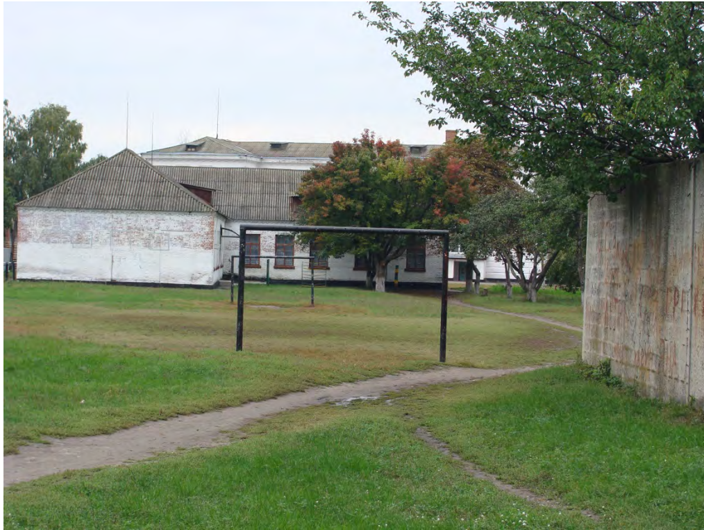
Picture 3. School #3 and its territory near the gas boiler house fence.
