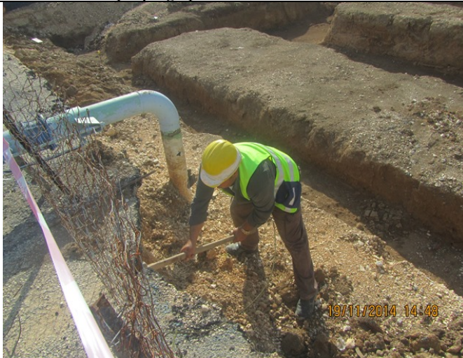
Opening the drainage pipe to remove the rainwater from the pumps area-SNW
