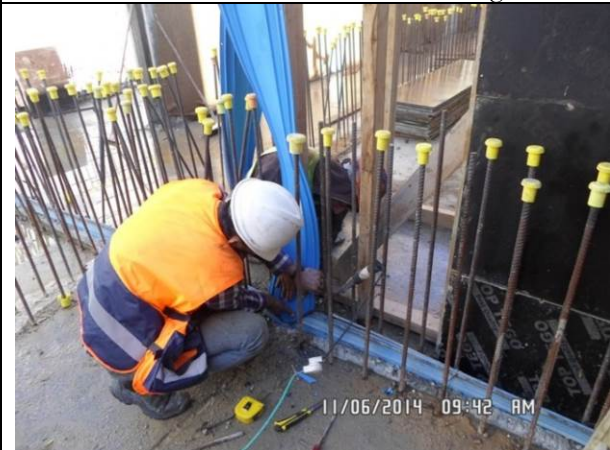
Arraba Well: Visual inspection for water stop welding by manufacturer (FOSROC) representative- balance tank wall section (E2).
