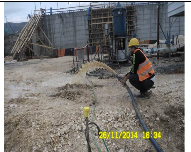
Rainwater suction by pump from the excavated rooms-SNW
