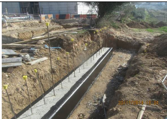
Photo date- 19 th of November, 2014: Start spreading, leveling and compaction of base course layer under chlorination room foundation.
