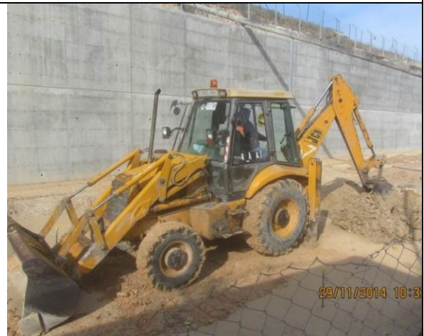
Photo Date- 29 th of November, 2014: Start excavations for re-located living quarter.
