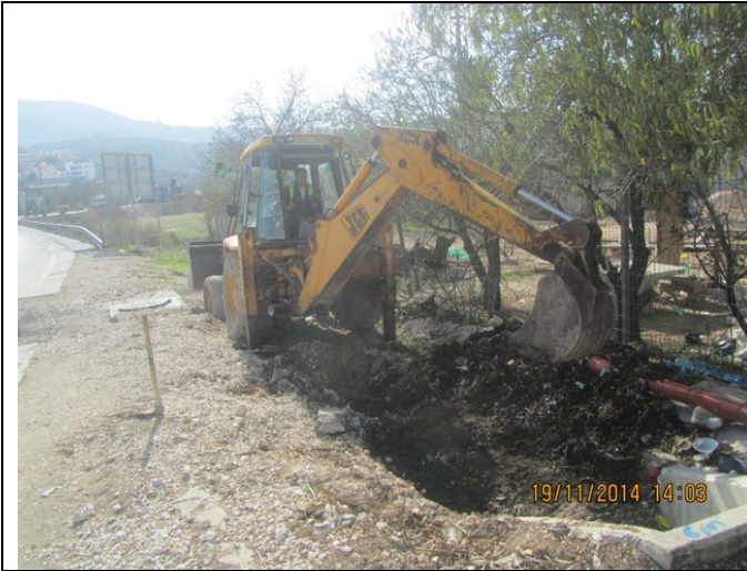
Trenches for rainwater-SNW
