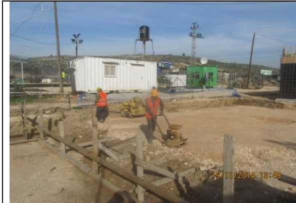
Photo date- 19 th of November, 2014: Start spreading, leveling and compaction of base course layer under chlorination room foundation.
