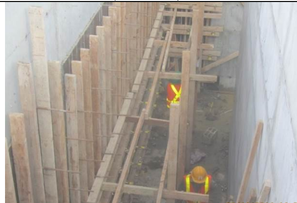
Photo date- 21 st of November, 2014: Start and finish casting concrete for balance tank wall (Section E1).
