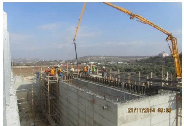
Photo date- 21 st of November, 2014: Start and finish casting concrete for balance tank wall (Section E1).
