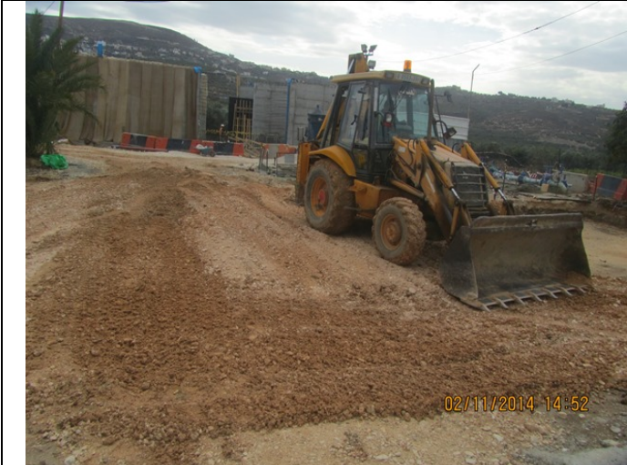
Spreading base course on the mud areas- SNW
