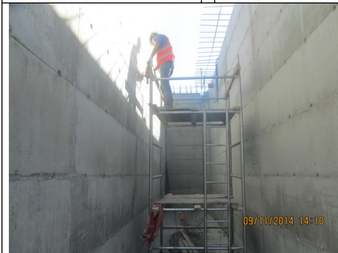
Steel scaffold for repair job inside the balance tank-ARW
