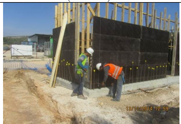
Photo date- 13 th of November, 2014: Continue formwork for living quarter building.
