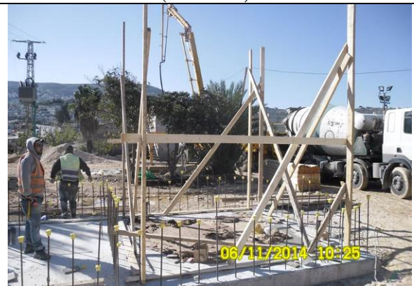
Photo Date- 6 th of November, 2014: Start formwork for living quarter walls.
