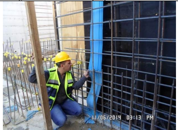
Arraba Well: Visual inspection for water stop welding by manufacturer (FOSROC) representative- balance tank wall section (E2).
