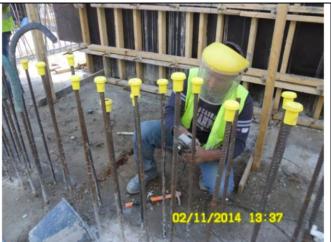
Special PPE while cleaning the steel bars-SNW
