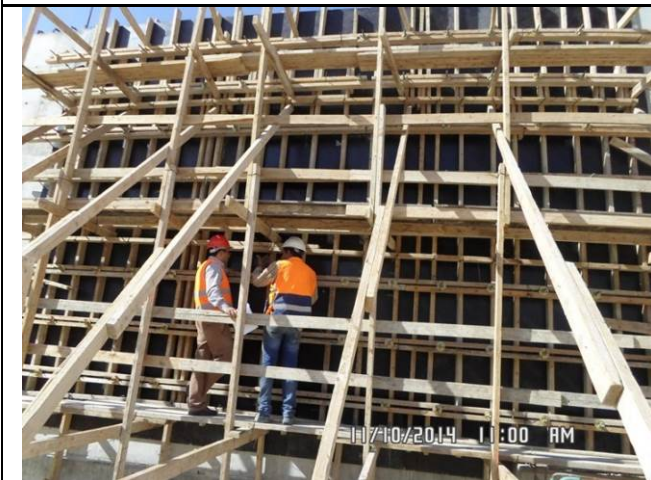
Formwork and scaffolding check -ARW
