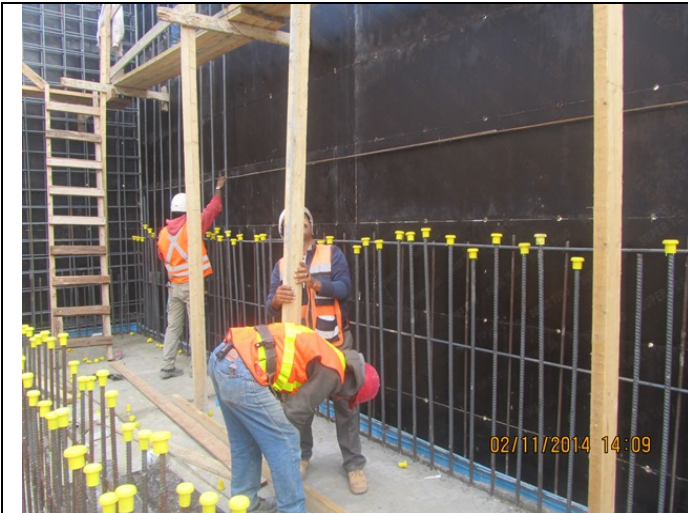
Scaffolding bracing-SNW
