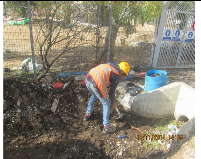
Trenches for rainwater-SNW
