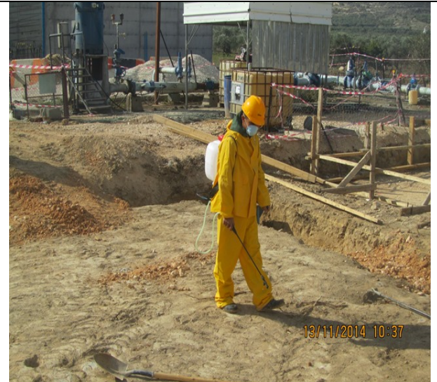
Spraying special material to remove the remaining tree roots wearing all safety PPEs-SNW
