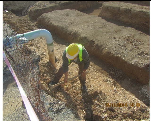
Opening the drainage pipe to remove the rainwater from the pumps area-SNW
