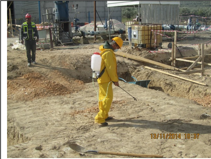
Spraying special material to remove the remaining tree roots wearing all safety PPEs-SNW
