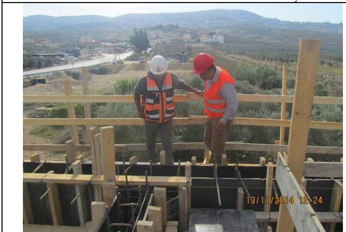
Formwork and scaffolding check -SNW
