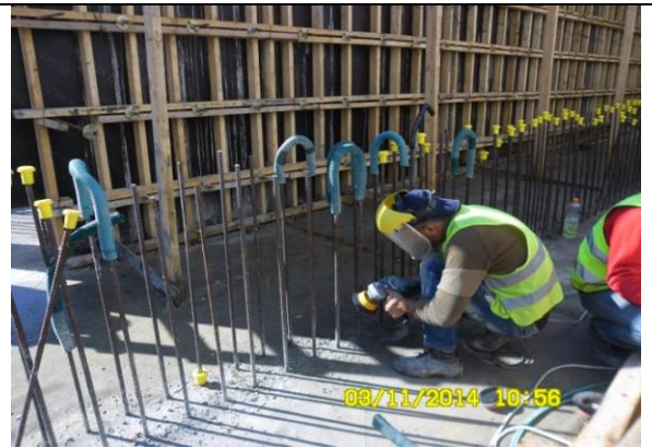
Photo Date- 3 rd of November, 2014: Dowels cleaning.
