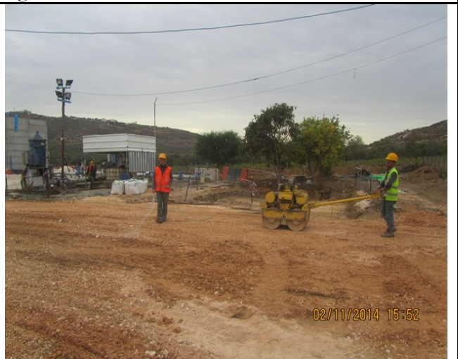
Spreading and compacting base course over the mud areas-SNW
