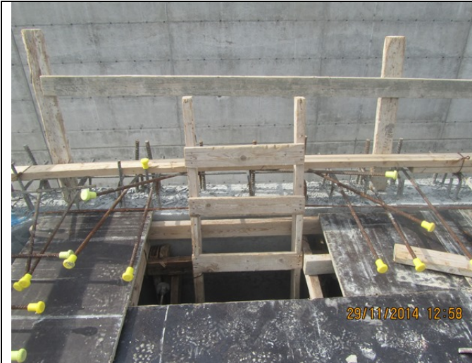
Safe access ladder to enter the balance tank-ARW
