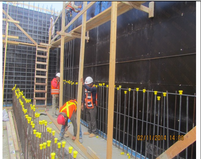
Scaffolding bracing-SNW
