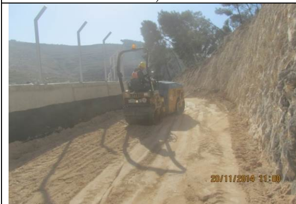
Photo date- 20 th of November, 2014: Continue backfilling and compaction over the underdrain system behind retaining wall.
