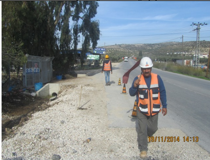
Flagman and reflective cones while working on the street to open trenches for rainwater-SNW
