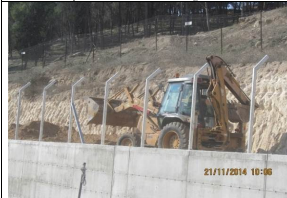
Photo date- 20 th of November, 2014: Continue backfilling and compaction over the underdrain system behind retaining wall.
