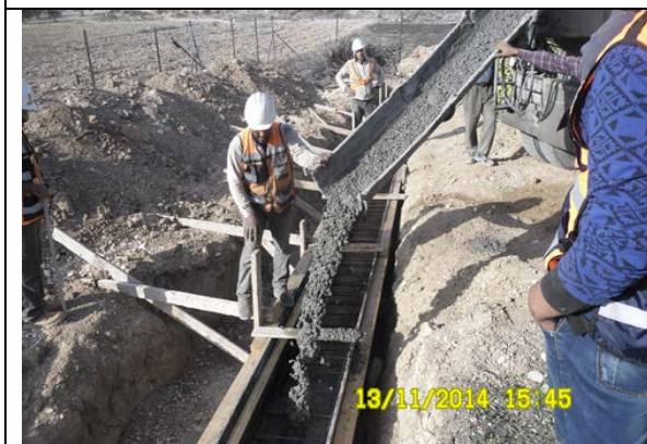
Photo date- 13 th of November, 2014: Casting concrete for fence wall (Segment-AB).
