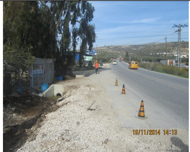
Flagman and reflective cones while working on the street to open trenches for rainwater-SNW
