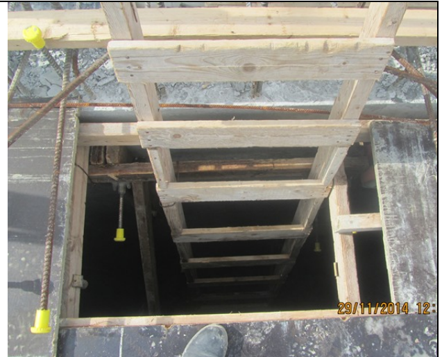
Safe access ladder to enter the balance tank-ARW
