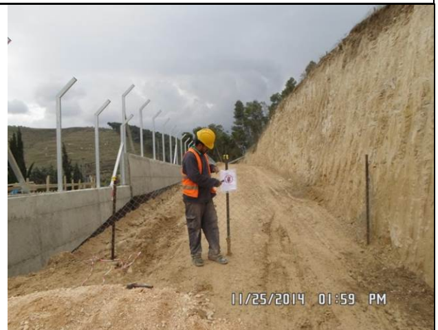
Fence installation with warning sign behind the retaining wall-ARW
