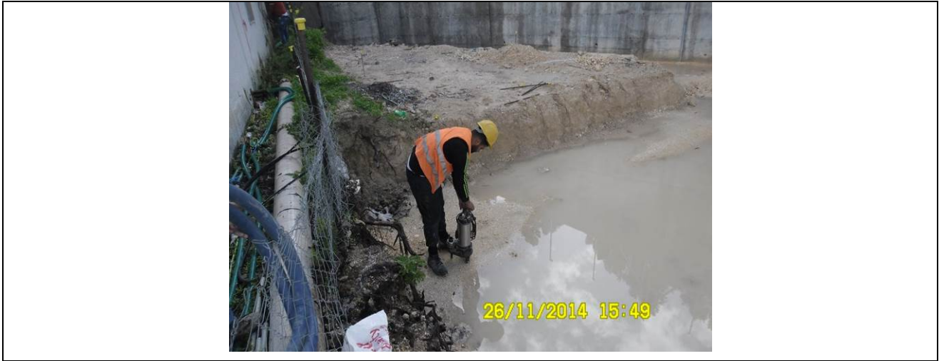
Rain water suction by pump from the excavated rooms-ARW
