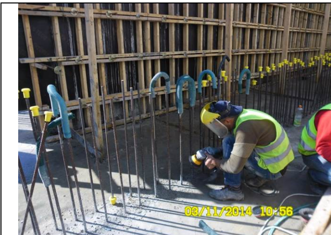
Special PPE while cleaning the steel bars-SNW
