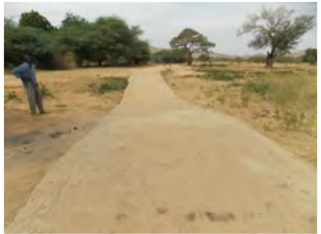
Rural road and bridge built with Nema FFW (Douentza) (November 2013) (Photographer: Isack Dolo).
