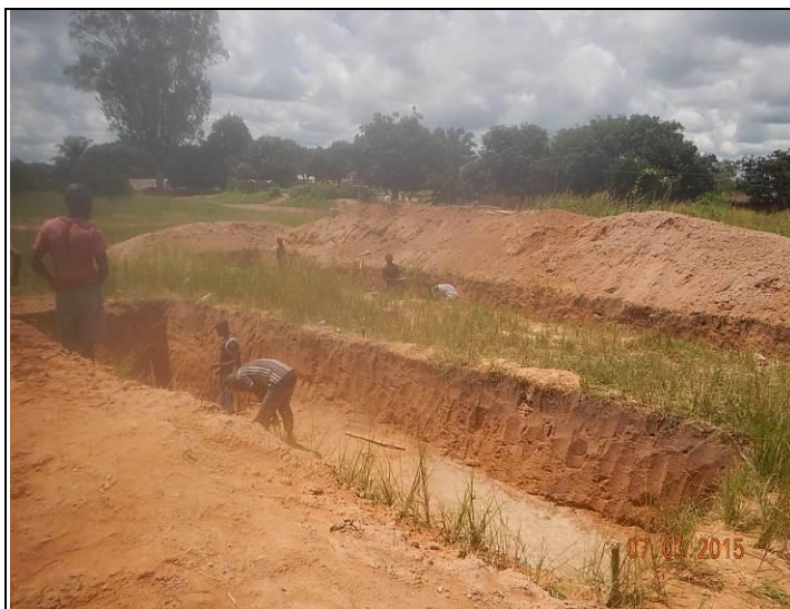
Photo de site EP. BUKANDA (At the beginning of the intervention)
