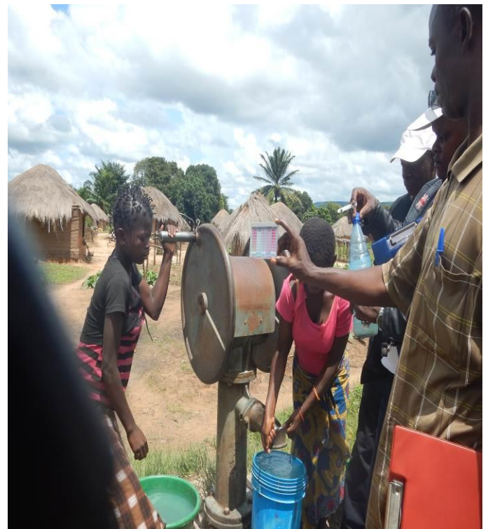
Photo of the borehole in LWINYA village (after maintenance)
