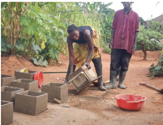
Women alongside men molding hand wash systems in concrete
