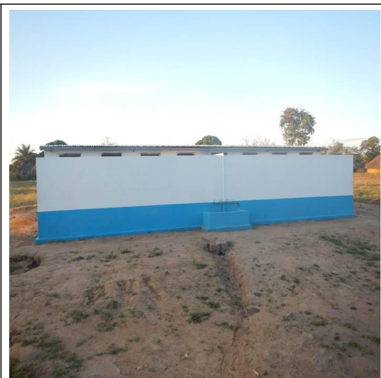
Photo de site EP. NKAMBO (after construction)
