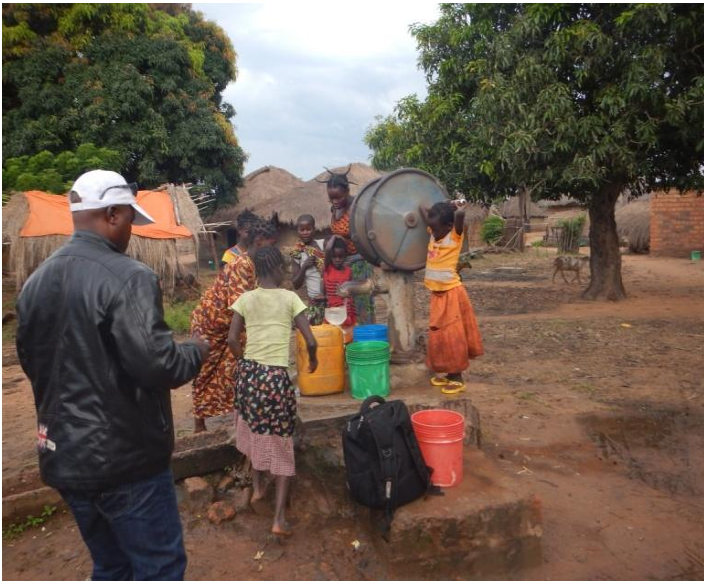
This water point in Nsange has been broken down for the past 3 years. Now in use after maintenance from the project
