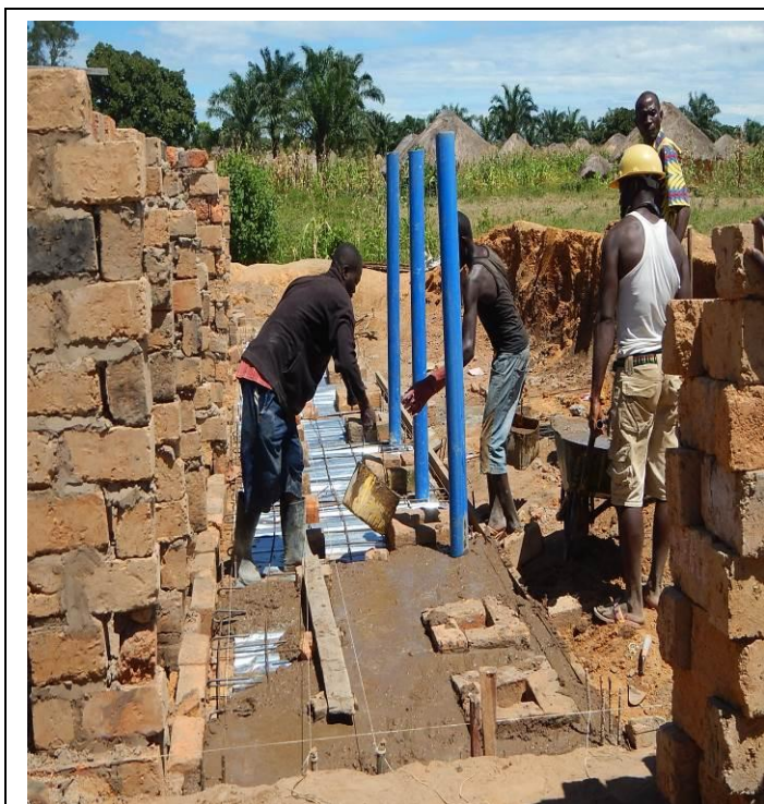
Photo of the site EP. NKAMBO (during construction)
