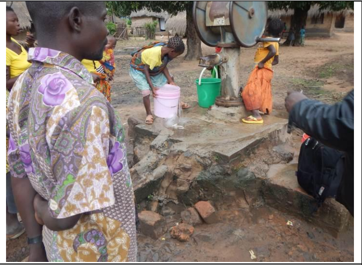
Photo of the borehole in LWINYA village (after maintenance)
