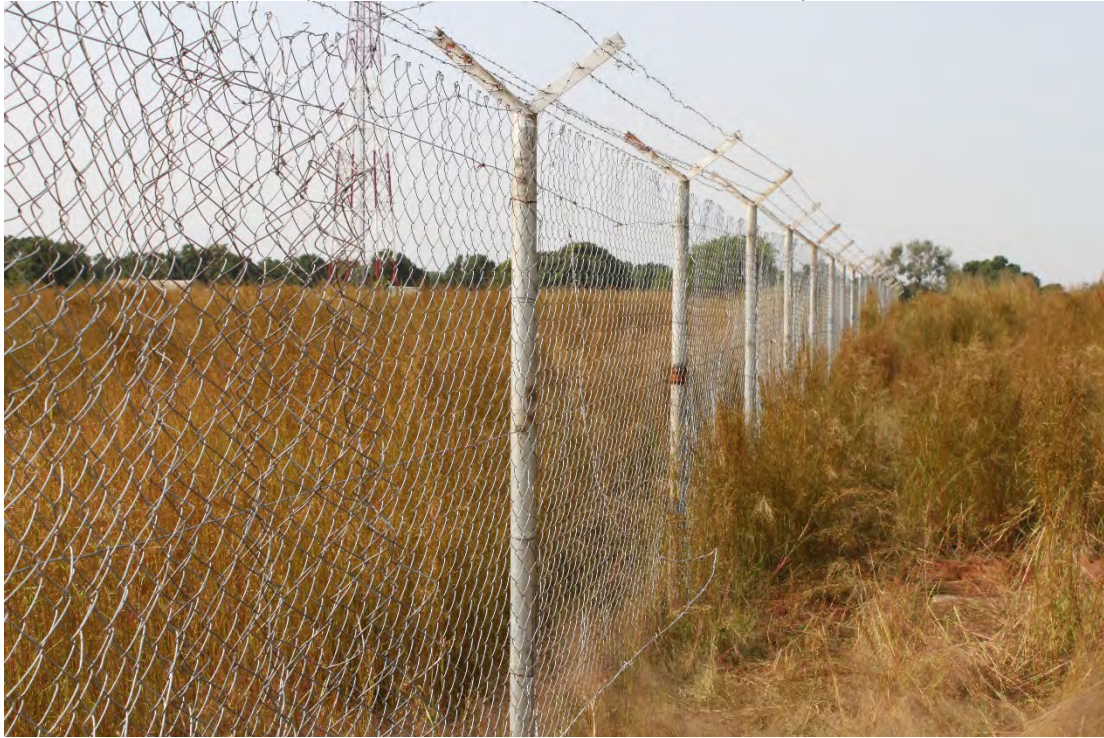
(Installation of New Fence-CUoSS, Wau)
