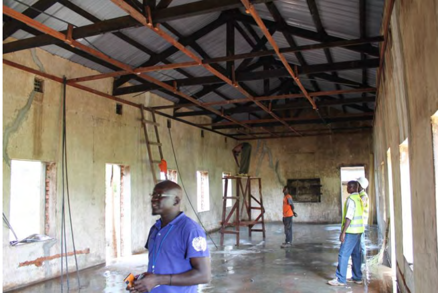
Renovation of Existing Classroom Space, CUoSS, Wau (2013)
