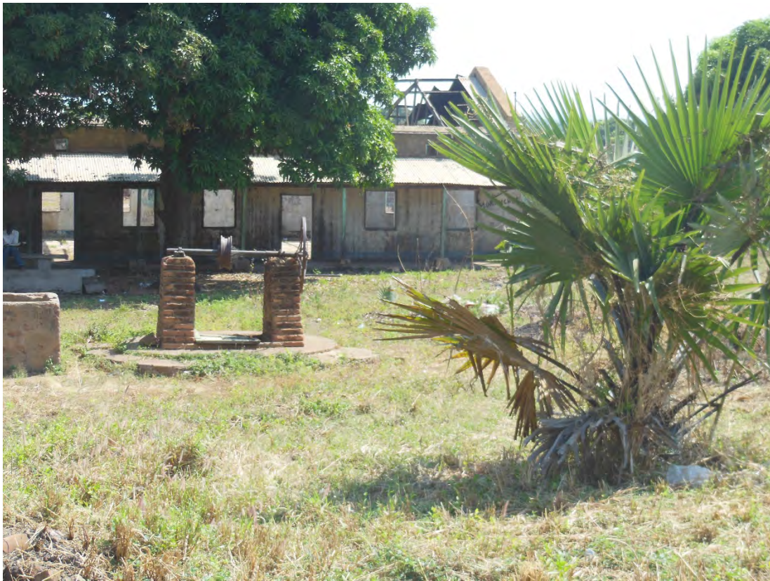
(New borehole and water supply system, CUoSS-Wau)
