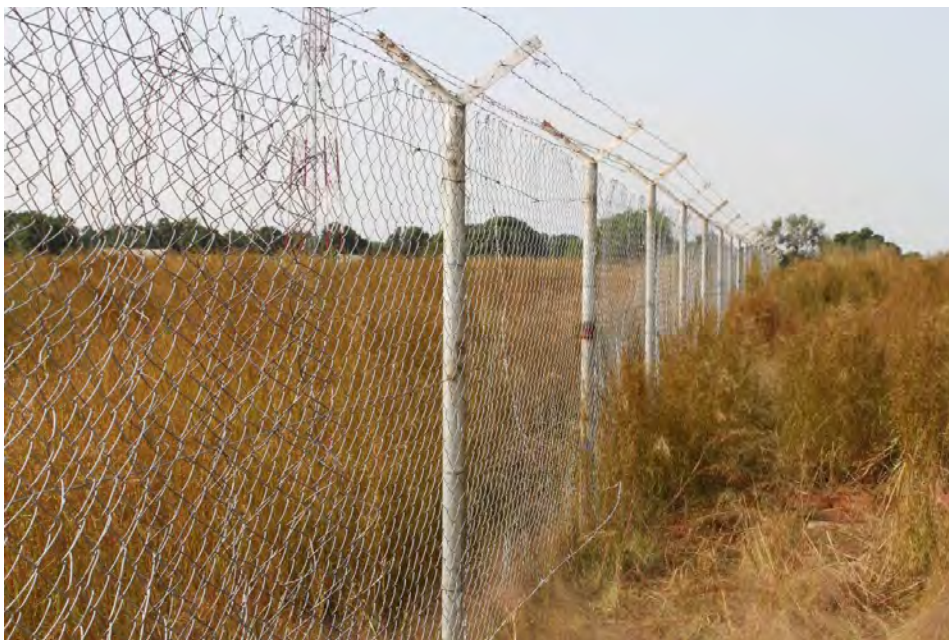
Installation of New Fence, CUoSS, Wau (2013)
