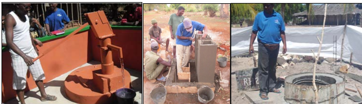
Photo 7. Newly rehabilitated pump well, Well rehabilitation (Boeny), 'Two-headed' fountain (Menabe)
