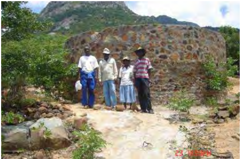
Water storage tank under construction in Nyatondo Village. Water will be piped from a reservoir uphill to be stored in the tank. Four committee members stand in front of the tank.
