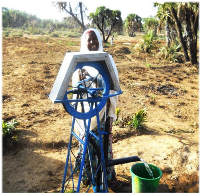
Aissata Moumouni using the shallow borehole with manual hand-pump installed by FABRIC
