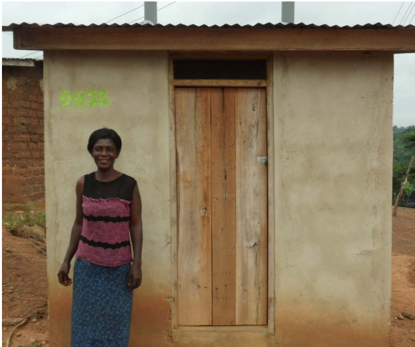
Beneficiary excited about completed household latrine
