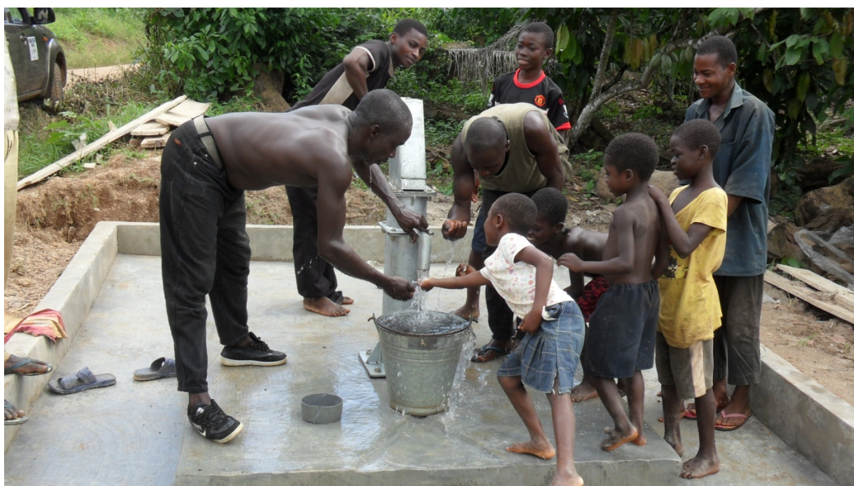
Local community members testing newly installed borehole pump
