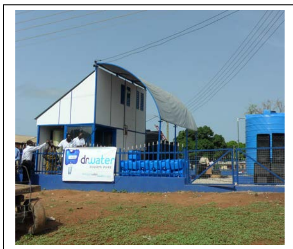
Water Health Kiosk – Dambai, Volta Region
