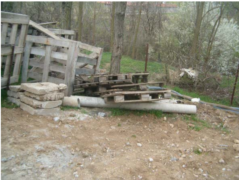
Asbestos water pipe.
