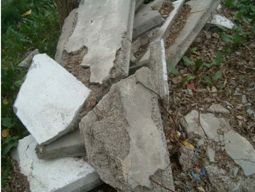
Removed damaged fibrous asbestos-cement sandwich.
